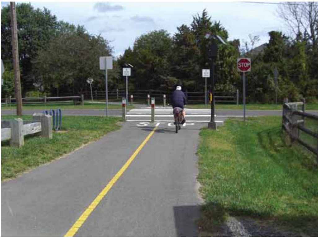
Wall Township's Route 18 Bike Path is a local example of a trail facility serving a transportation function.
