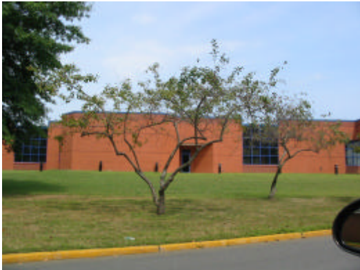
Slope on the south east side of the Ag. Building allowed water run off to spill from storm drains into the stream located next to the rear parking lot.
