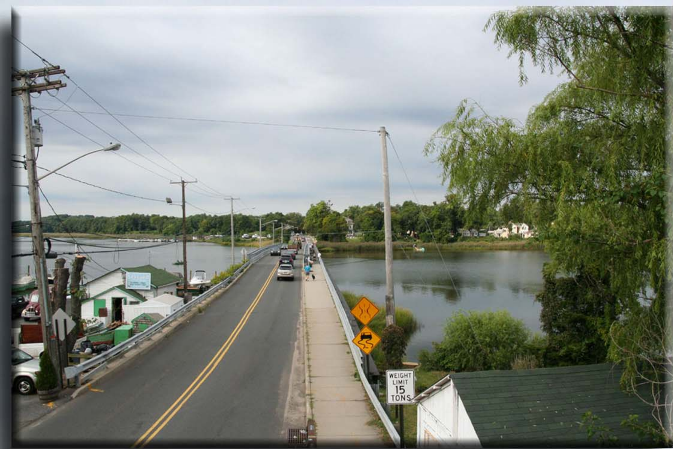
Existing Site Condition
