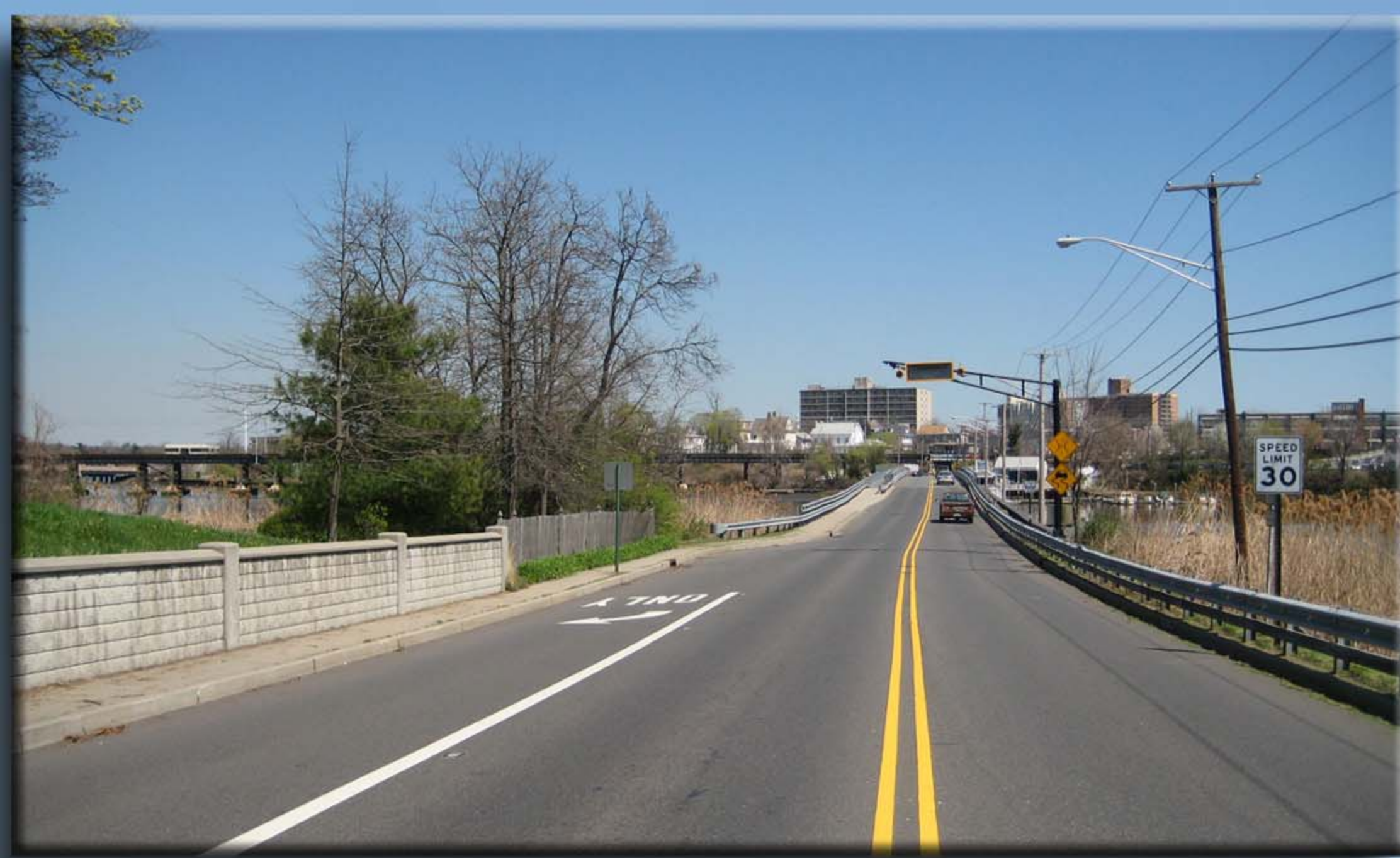
Existing Site Condition
