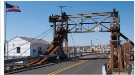
Brielle Road over The Glimmer Glass (W-9)
