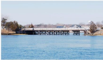
Green Avenue over Debbie's Creek (W-7)
