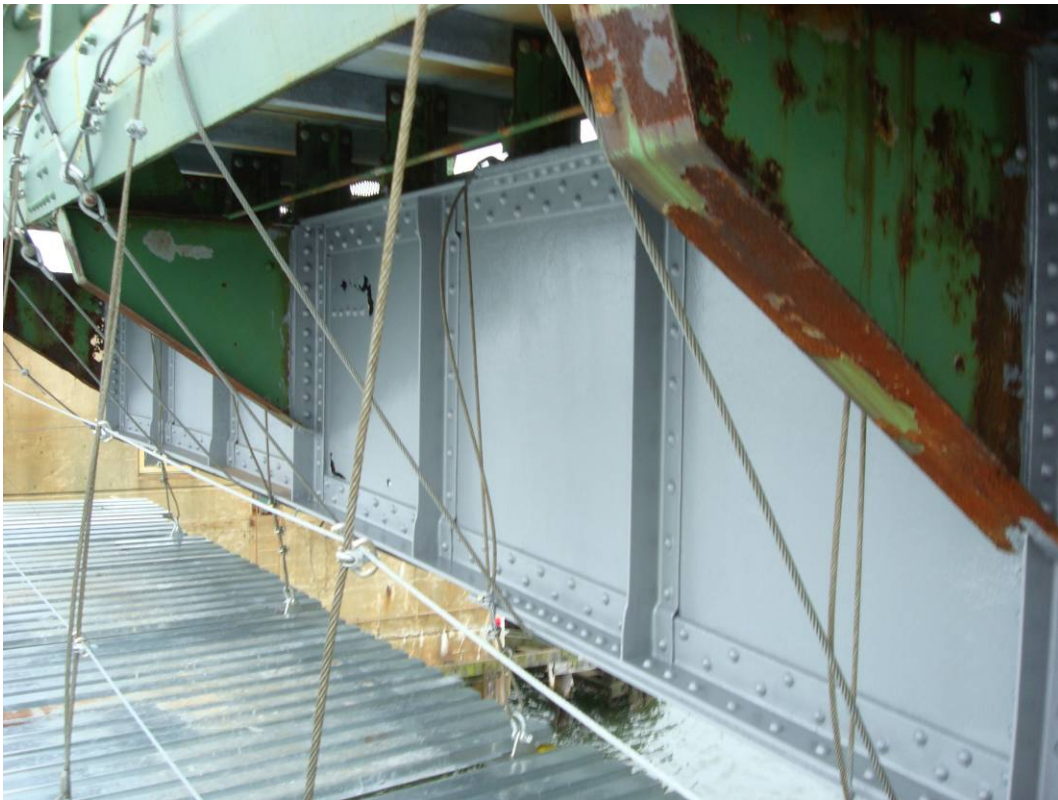
Photo 18: East bascule girder cleaned with hand and power tools. Looking South.
