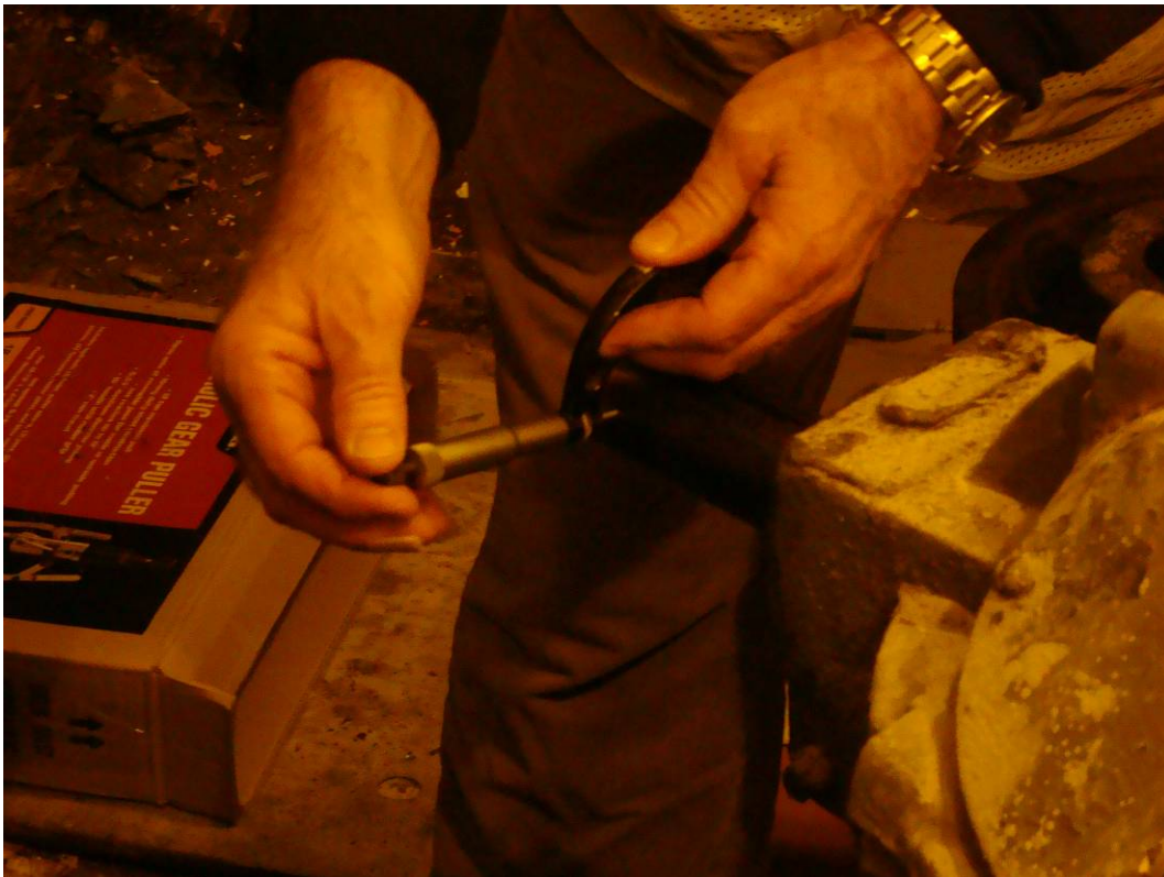
Photo 29: North leaf machinery components- The Contractor field measured the shaft diameters of the main electric and auxiliary gas motors, auxiliary reversing unit and the main differential reducer so that the openings of the new components will sized correctly.
