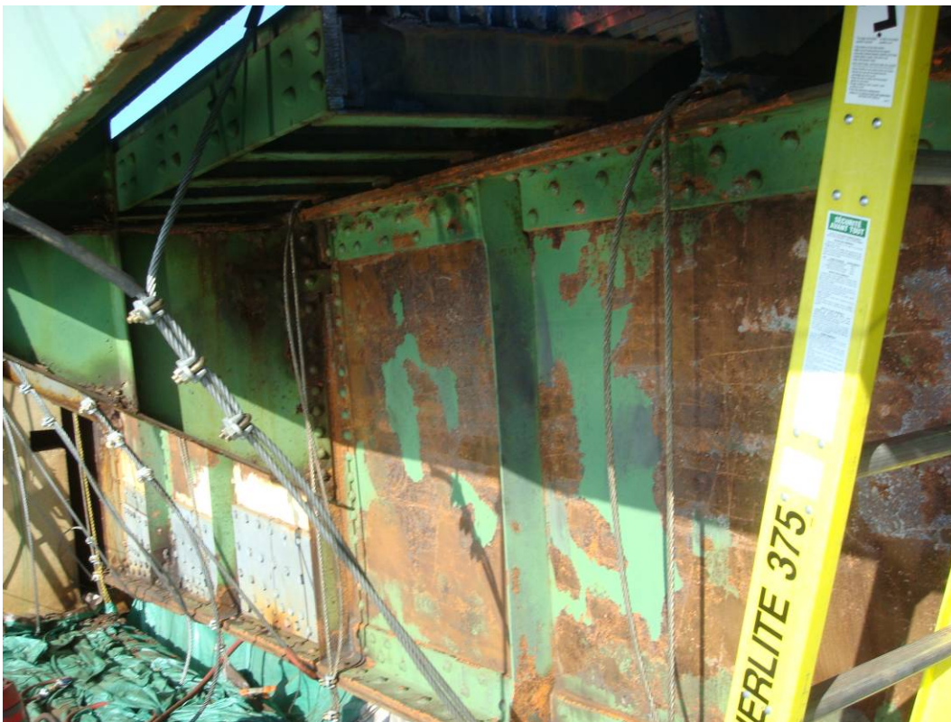
Photo 11: West bascule girder cleaned with hand and power tools. Looking North.
