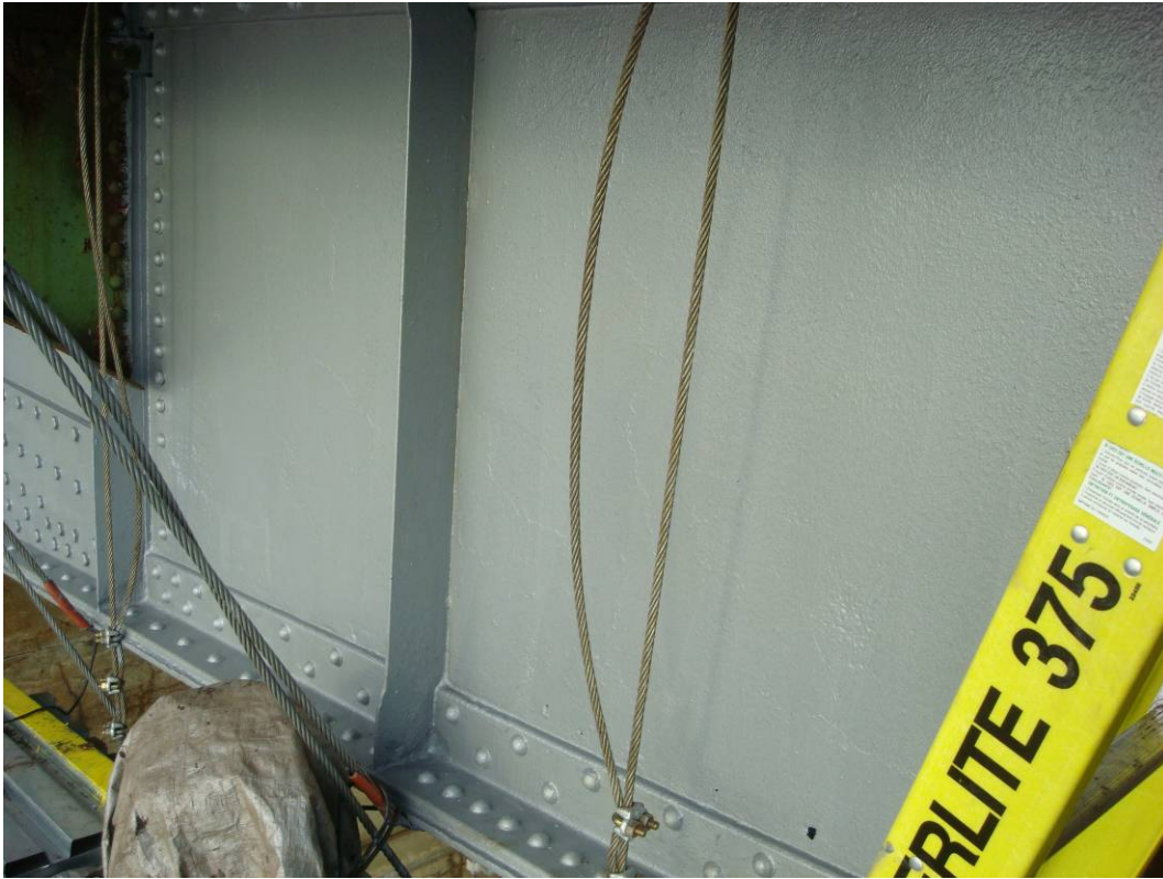
Photo 12: West bascule girder primed with Epoxy Mastic Aluminum.
