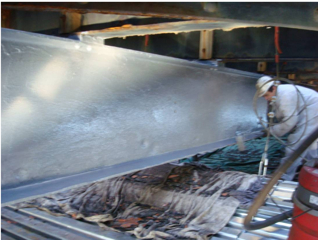
Photo 15: South face of Intermediate Floorbeam FB2 primed with Epoxy Mastic Aluminum.
