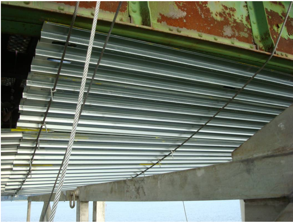
Photo 3: Installation of Temporary work platform.
