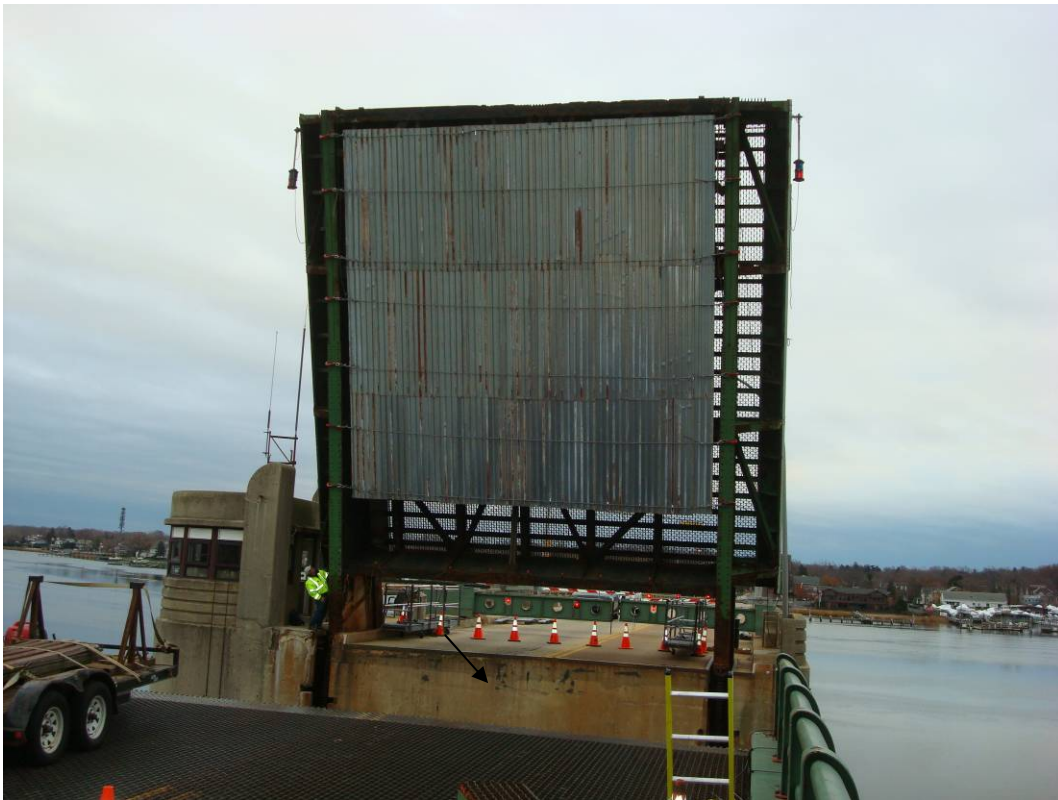
Photo 30: South Leaf –Temporary Platform.
