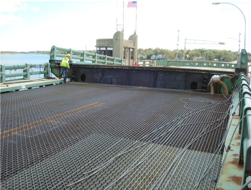
Photo 2: Installation of temporary work platform of North leaf.
