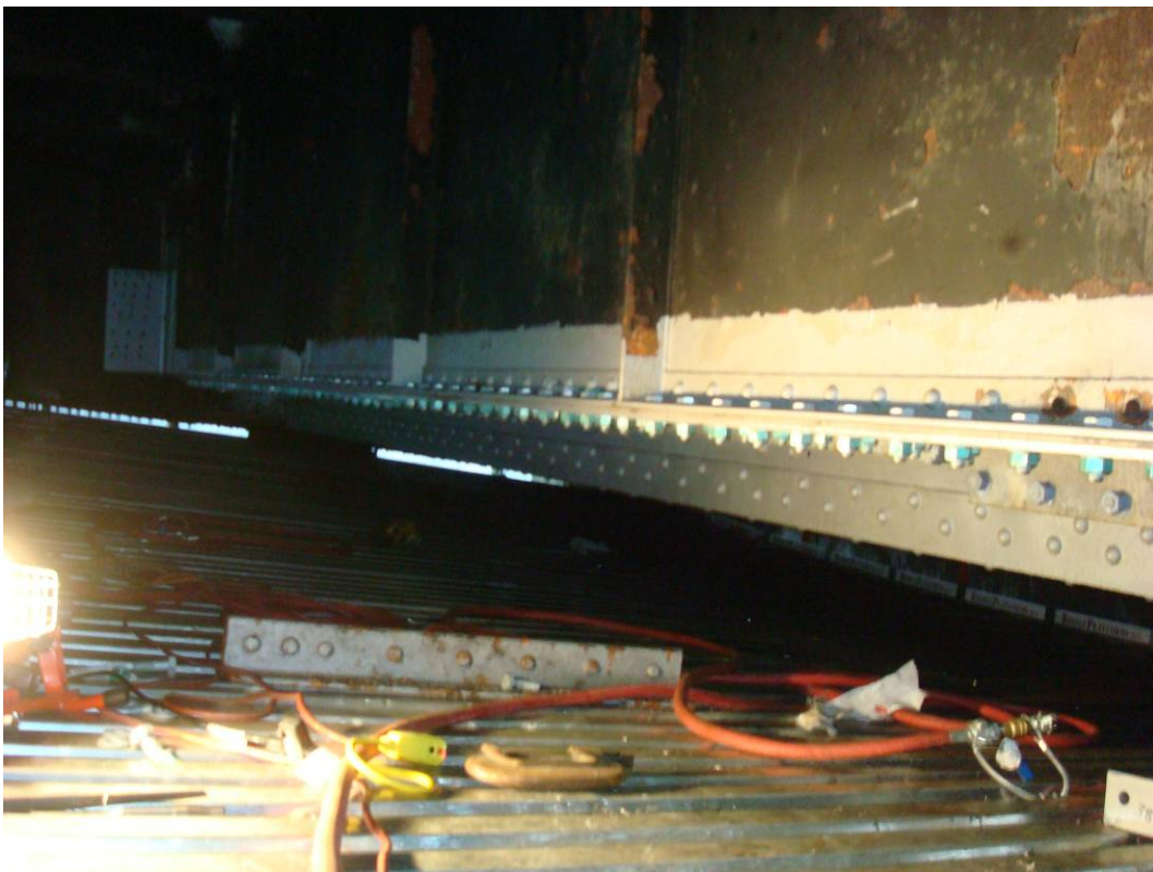
Photo 21: Floorbeam FB5, Bottom flange strengthening plate repair nearly completed.
