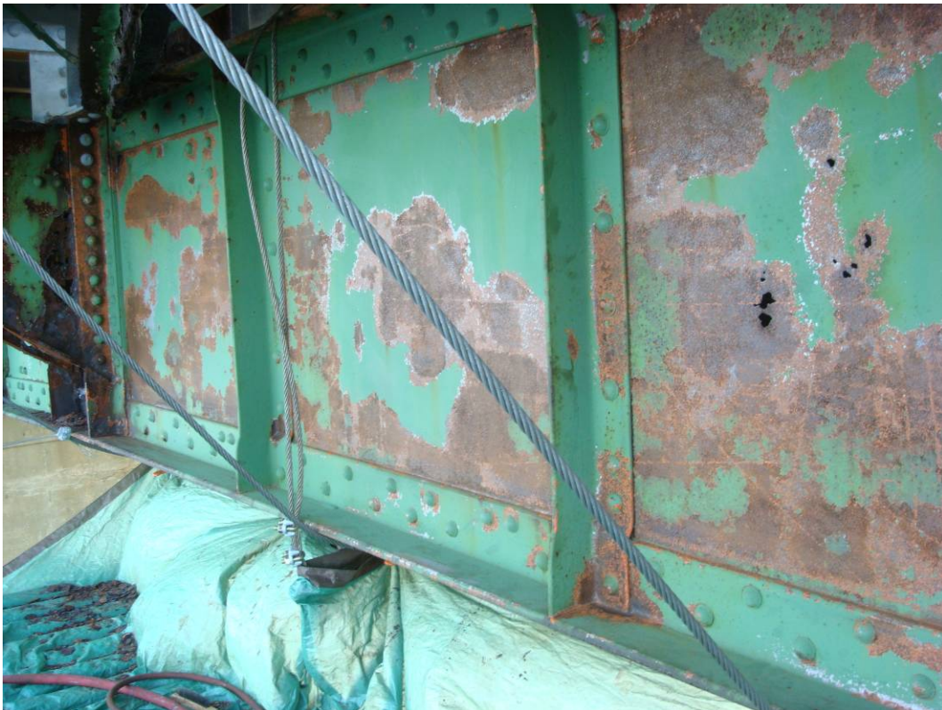
Photo 17: East bascule girder cleaned with hand and power tools. Looking South.
