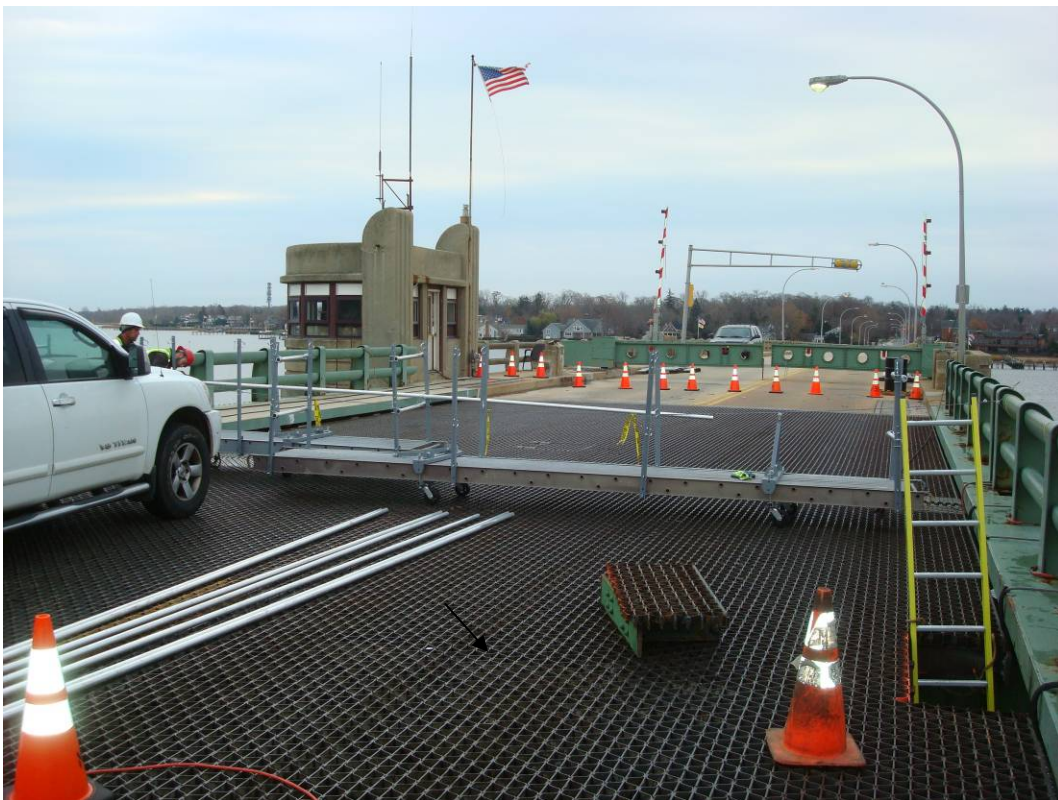
Photo 31: Swing stages to facilitate FB1 replacement.
