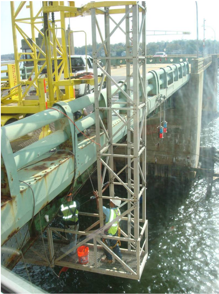
Photo 5: Installation of temporary work platform.
