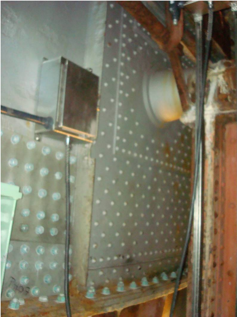
Photo 95: Navigation lighting droop cable installed.
