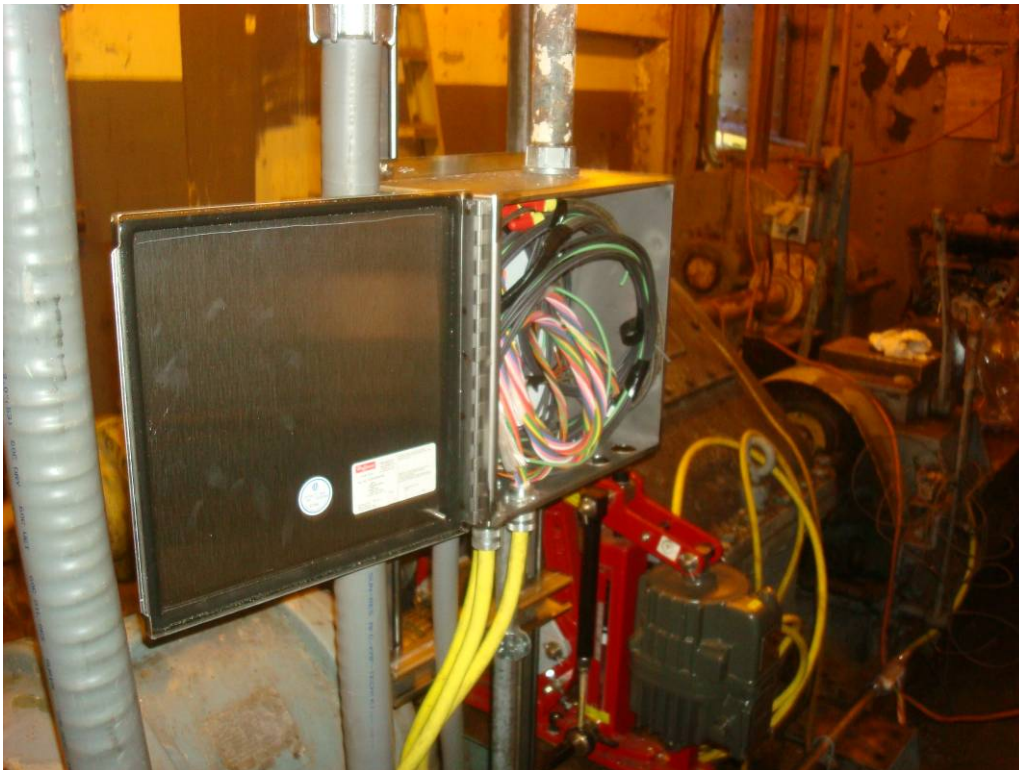
Photo 91: New junction box for the machinery and motor brake tie into the bridge wiring.
