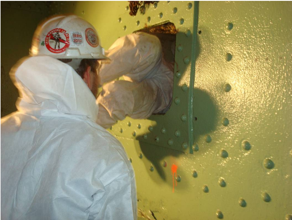
Photo 76: New lead brick being installed into the west counterweight pocket in progress.
