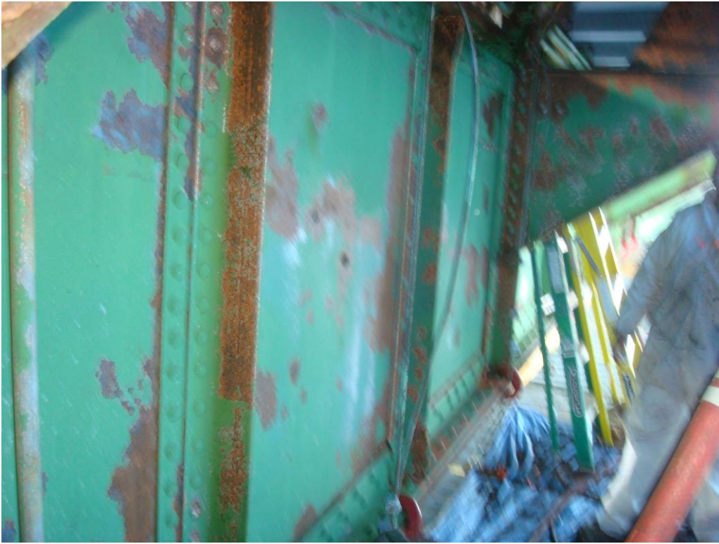
Photo 28: The East girder elevation looking at FB3 of the South leaf cleaned with hand and power tools.
