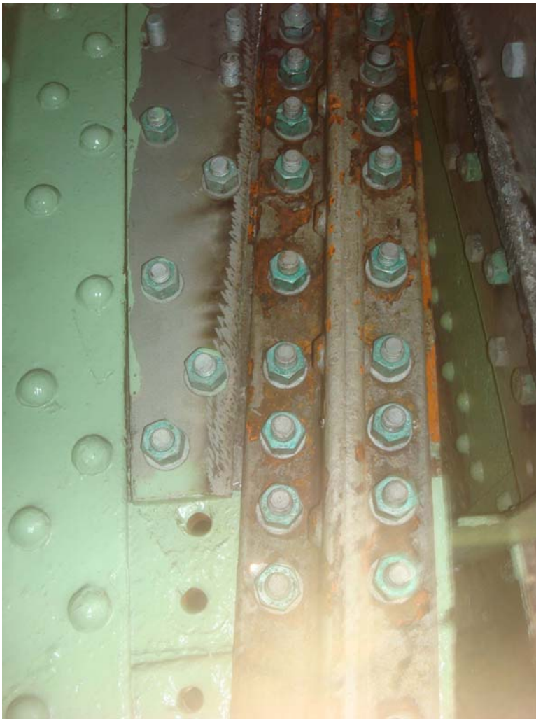
Photo 80: The temporary tie-down has been removed and the existing vertical stiffener has been re- installed.
