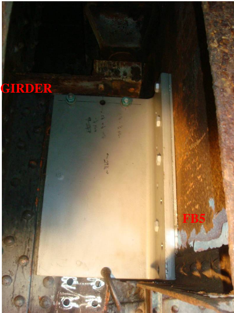
Photo 83: Installation of Temporary tie down between the FB5 and the East girder in progress.
