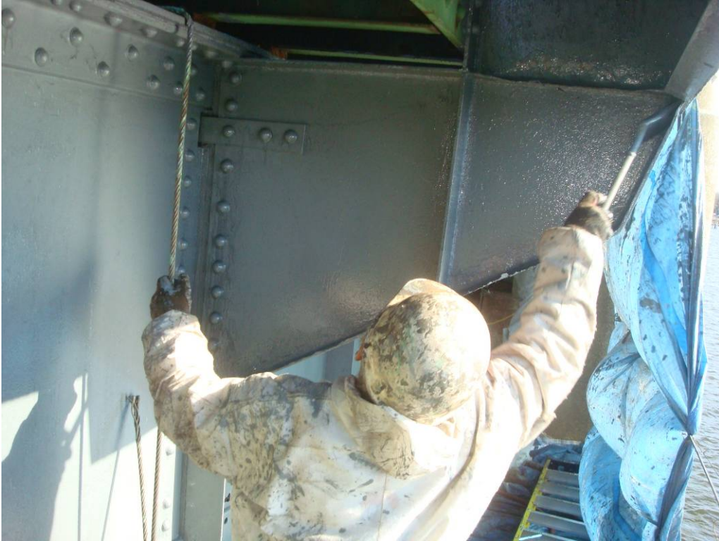
Photo 40: The Southwest girder cantilevered bracket at FB3 in progress of being primed with Epoxy Mastic Aluminum.
