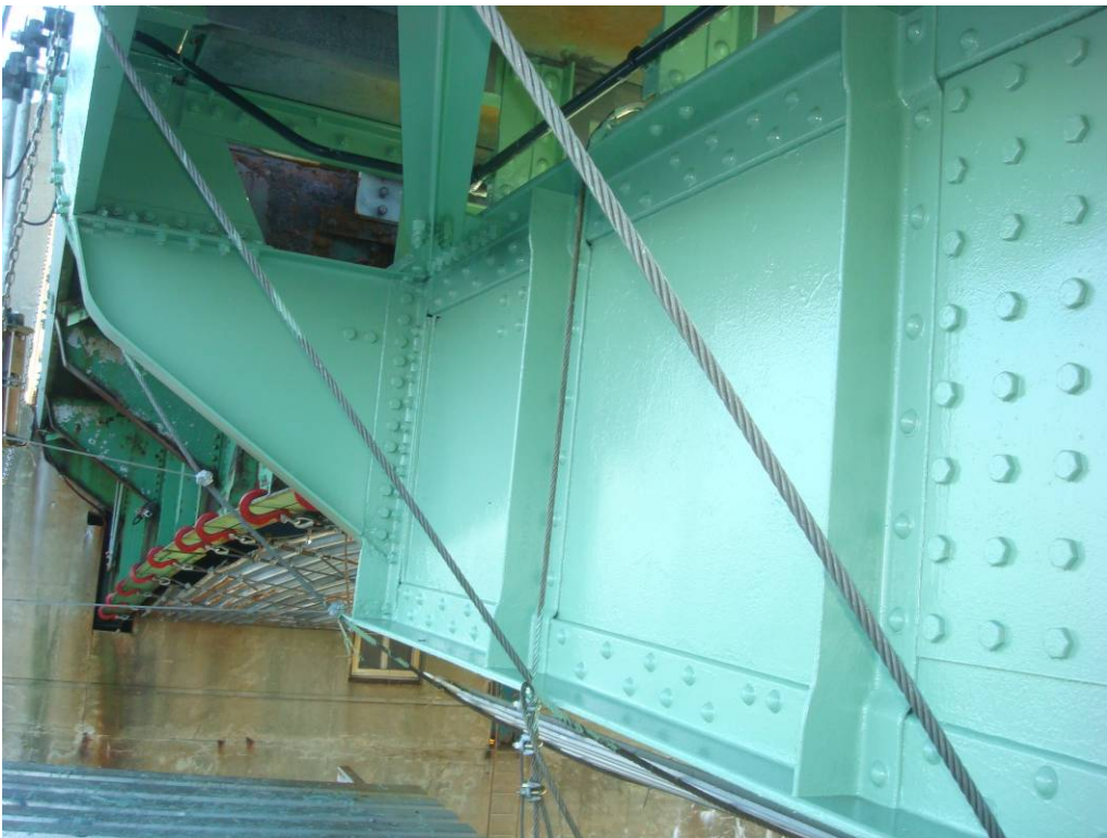
Photo 11: The painters primed the West fascia and touched up previously primed areas that were damaged due to the steel repairs.
