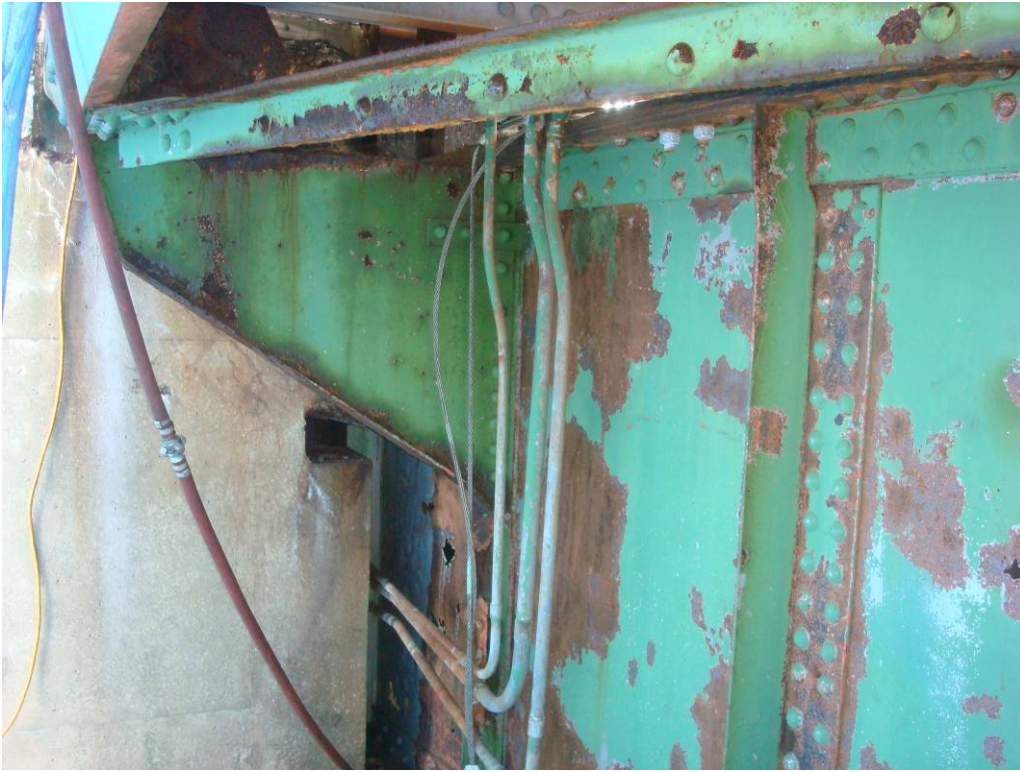
Photo 26: The East girder elevation looking at FB4 of the South leaf cleaned with hand and power tools.
