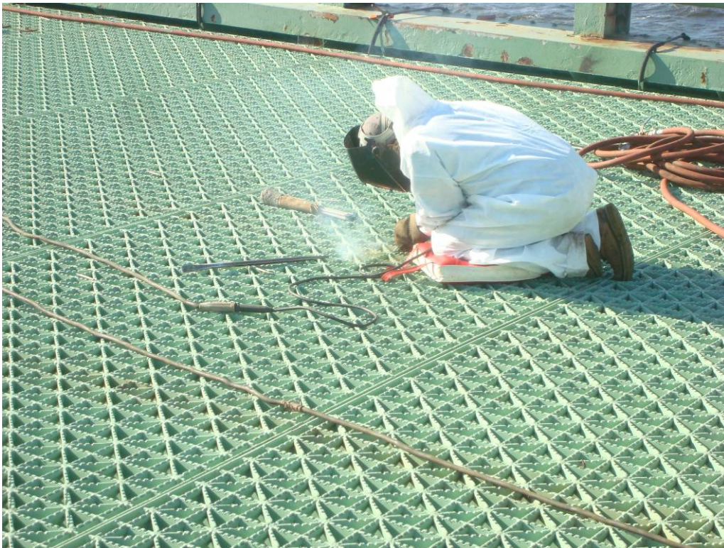
Photo 56: Welding the main bars of the new grating to the top flange of the stringers in progress.
