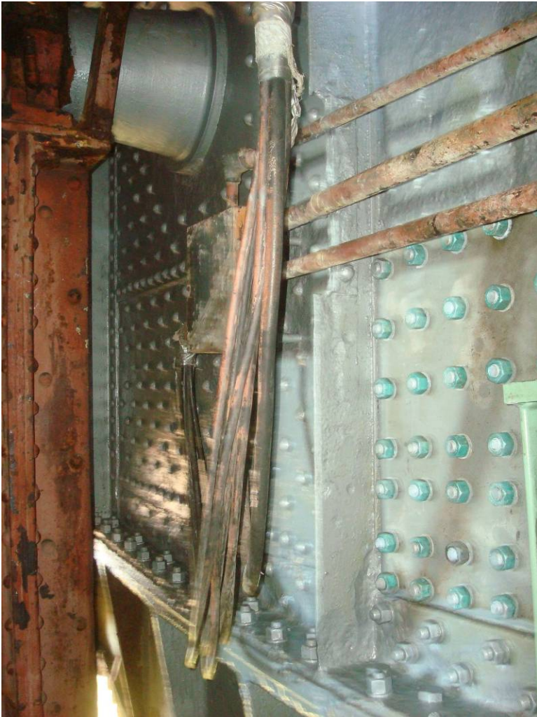
Photo 7: The painters primed the Southeast bascule girder and a portion of the rack at the trunnion area. East face shown.
