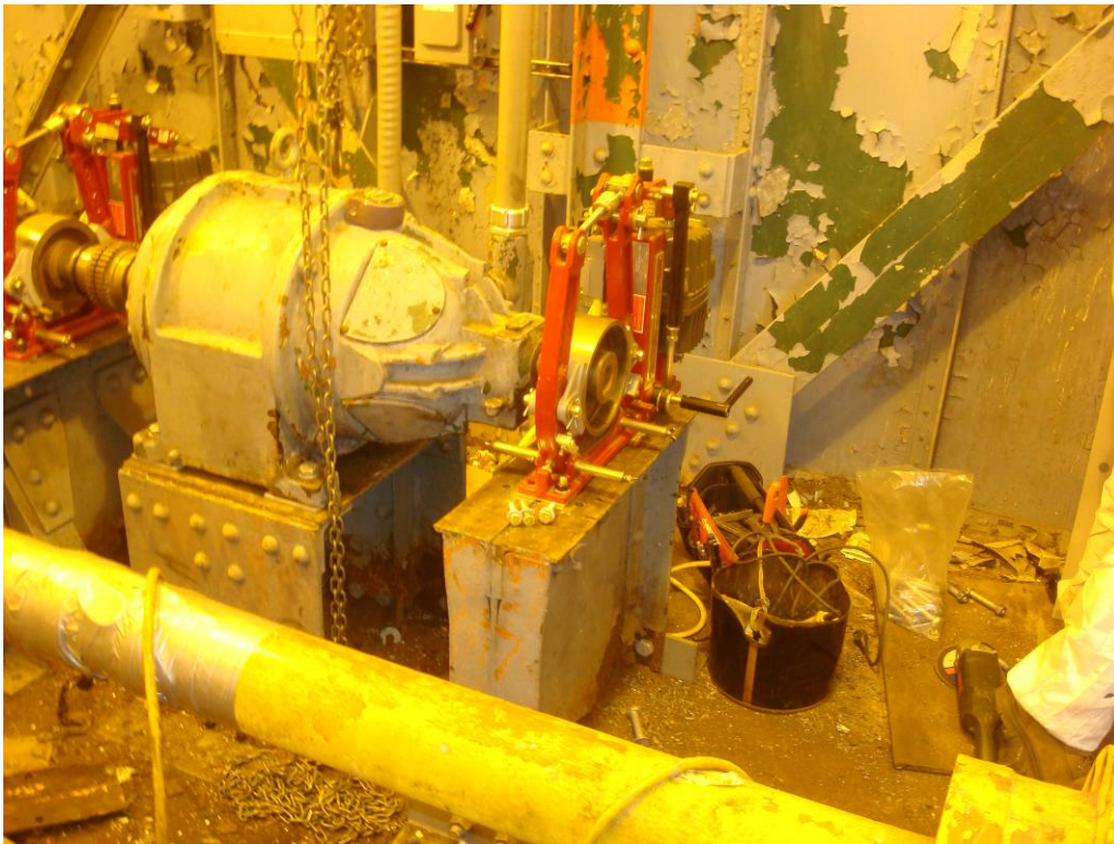
Photo 90: Motor brake installed.
