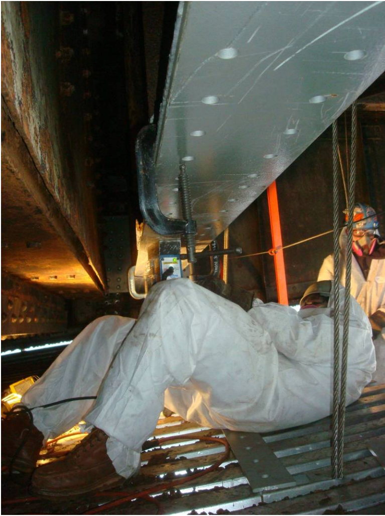
Photo 85: Bottom Flange of FB5 of South leaf repair in progress using the new repair plate as a template for field drilling of holes into flange.
