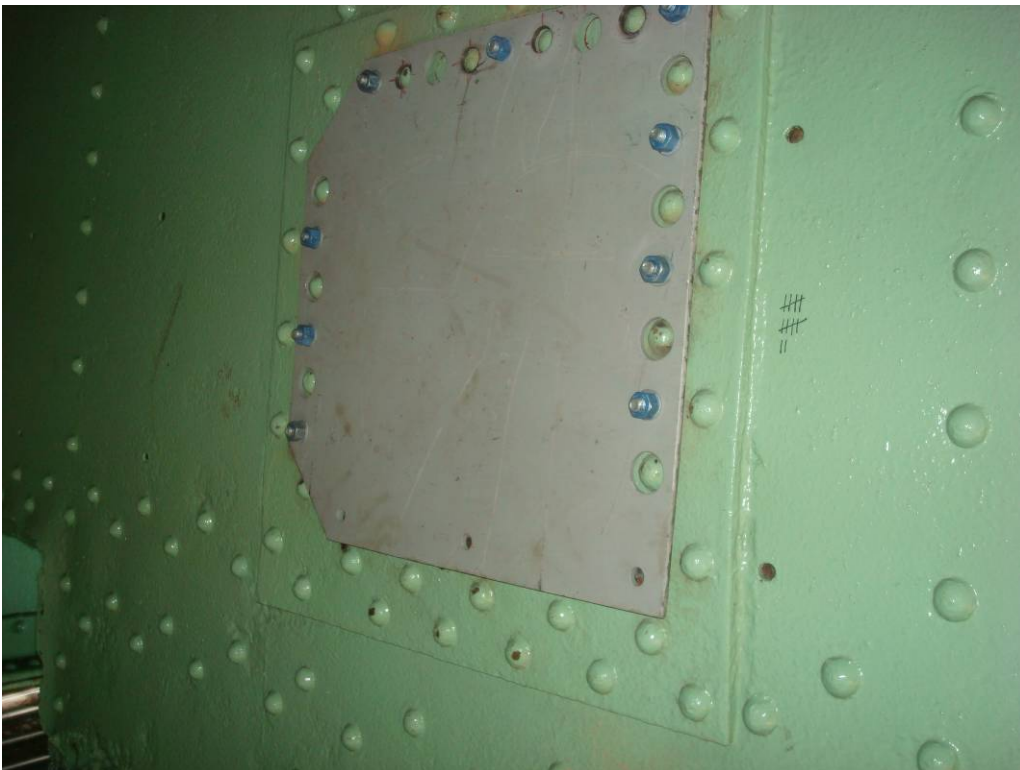
Photo 78: The ironworkers installed the west counterweight pocket cover plate.
