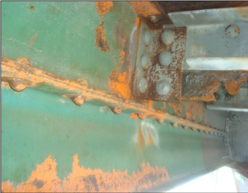
Photo 32: The Southeast girder elevation between the FB1 and FB2 cleaned with hand and power tools looking South.
