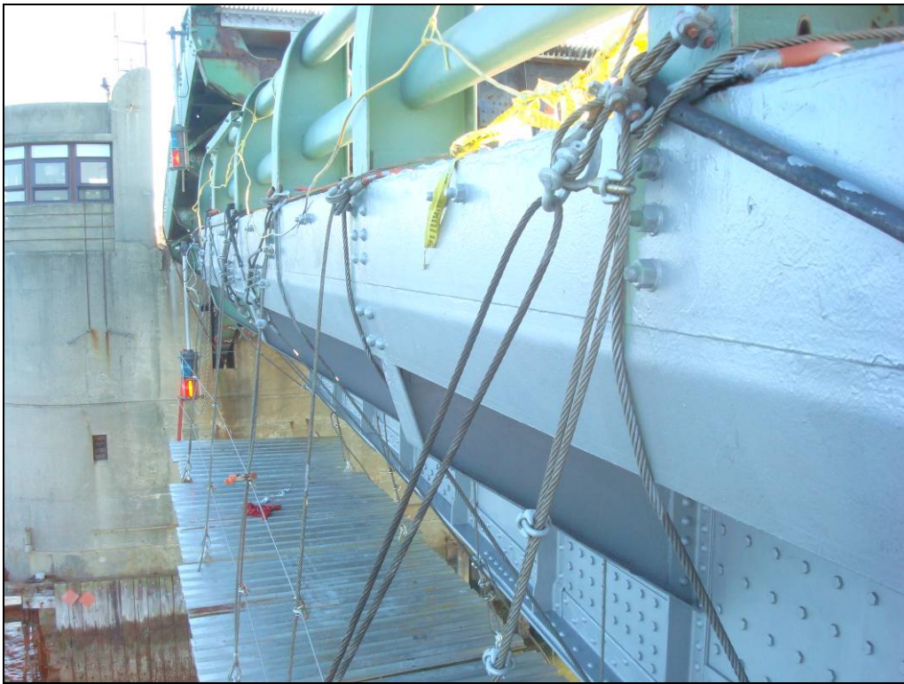
Photo 3: The painters primed the fascia plate and touched up previously painted areas on the East fascia. Ready for the top finish coat to be applied.
