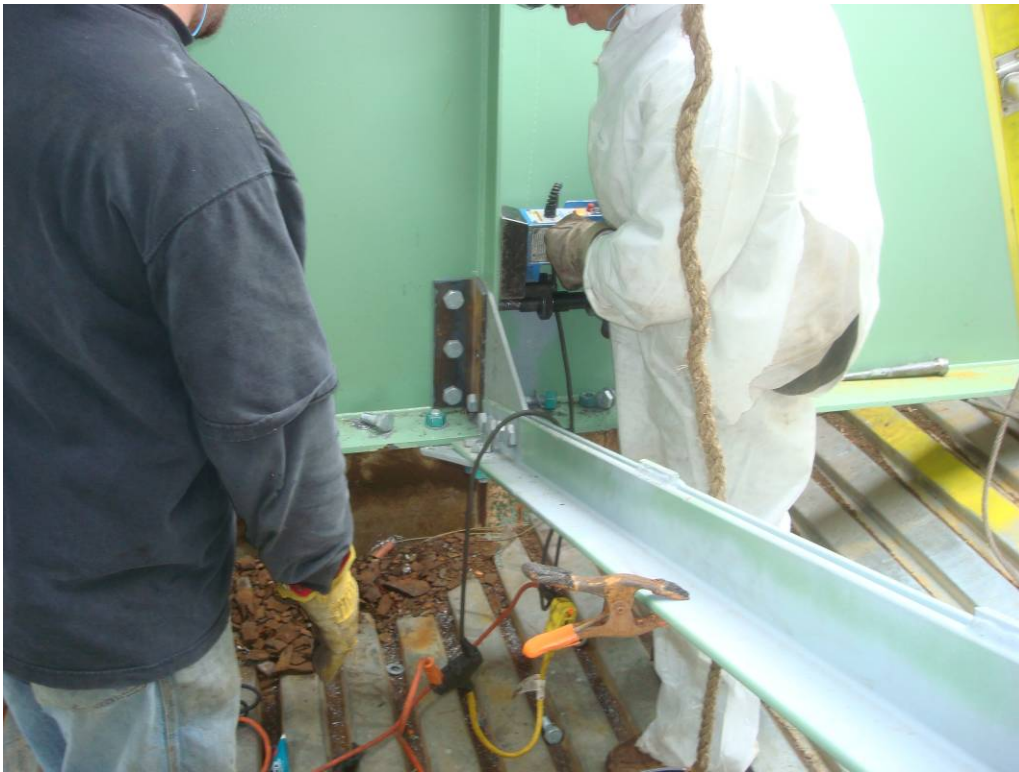
Photo 58: The iron workers are in progress of completing miscellaneous bracing connections on the north bascule span.
