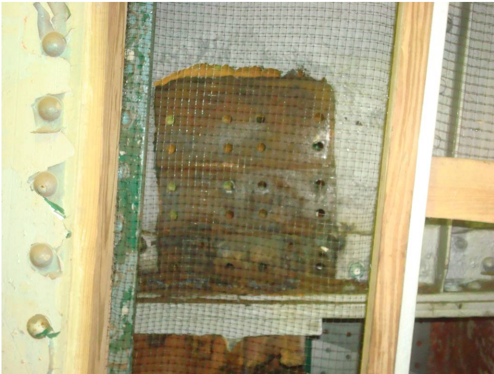
Photo 67: East face of Southwest bascule girder with front rack stiffeners removed.
