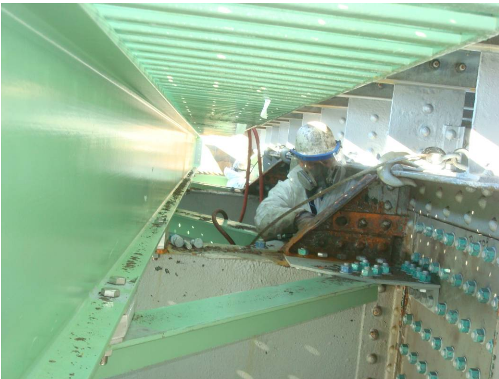
Photo 2: The painters were preparing the span for one final application of primer to the cleaned steel and touch up of previously primed steel.
