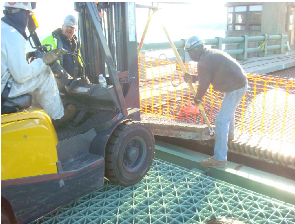
Photo 46: Installing the first section of toe joint using the forklift.
