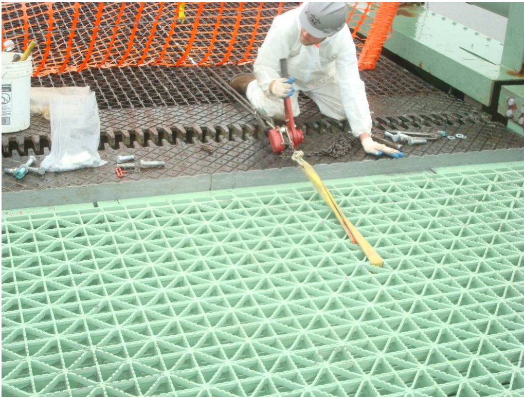
Photo 55: The ironworkers utilizing come-alongs to slide the grating deck into final position.
