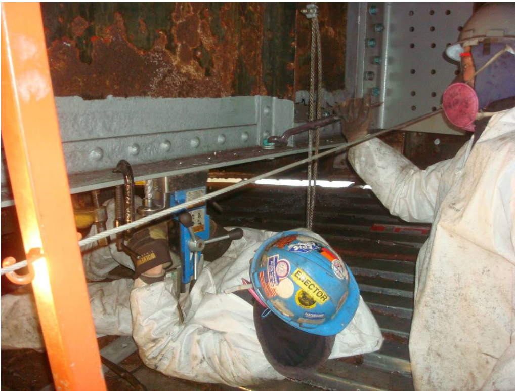
Photo 84: Bottom Flange of FB5 of South leaf repair in progress using the new repair plate as a template for field drilling of holes into flange.
