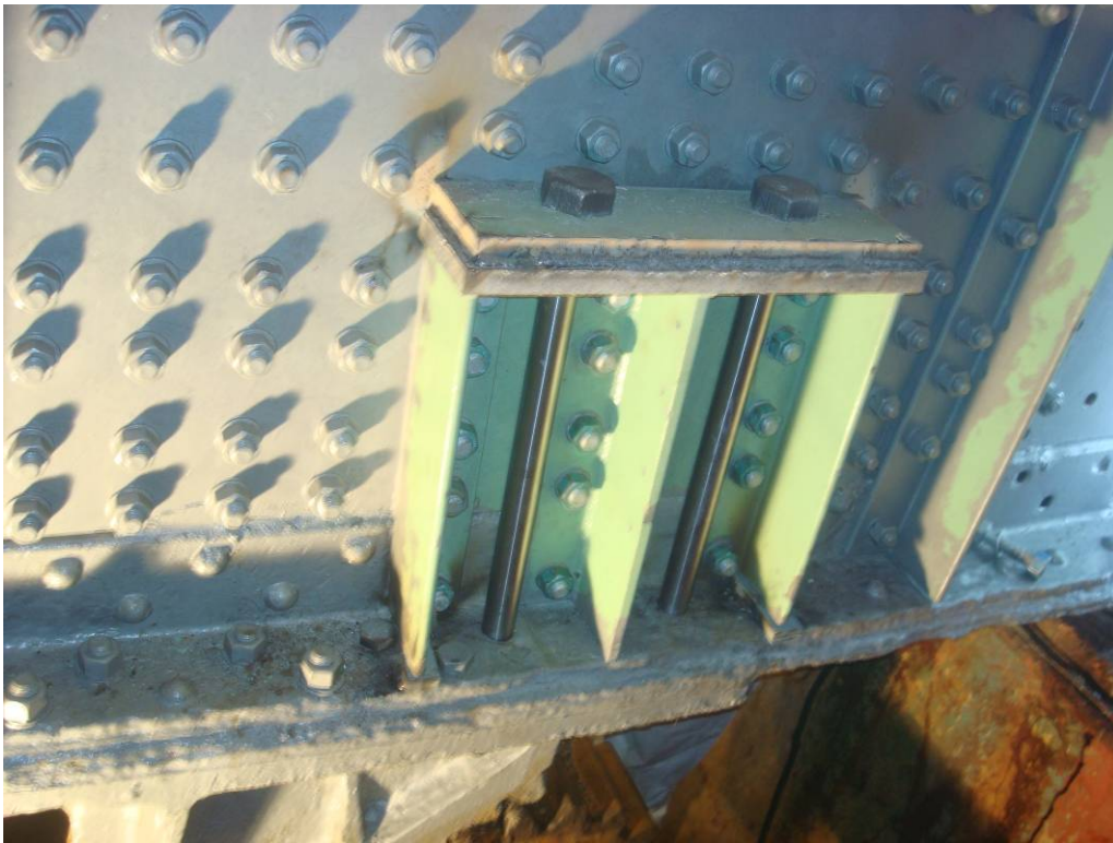
Photo 65: The West face of the West girder rack cap plate field welded to the top of the front rack stiffener.
