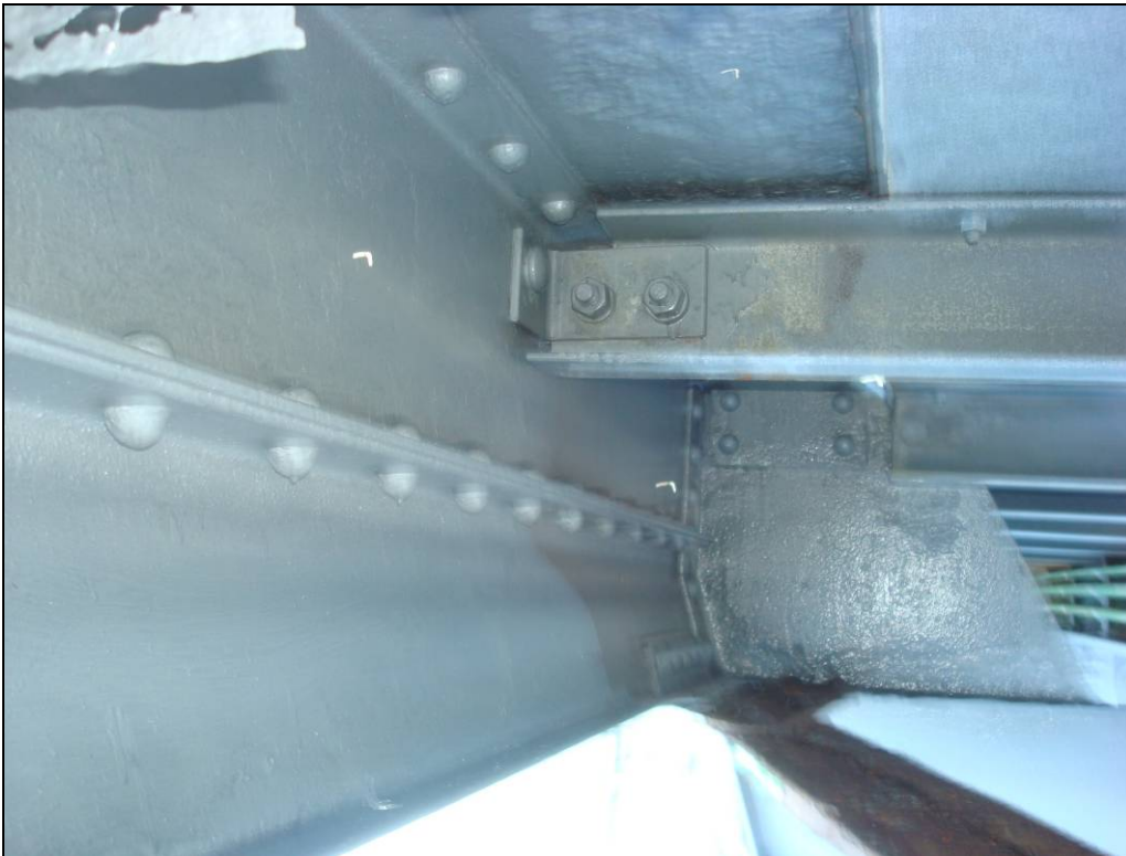
Photo 35: The Southeast girder under the fascia between the FB1 and FB2 primed with Epoxy Mastic Aluminum.
