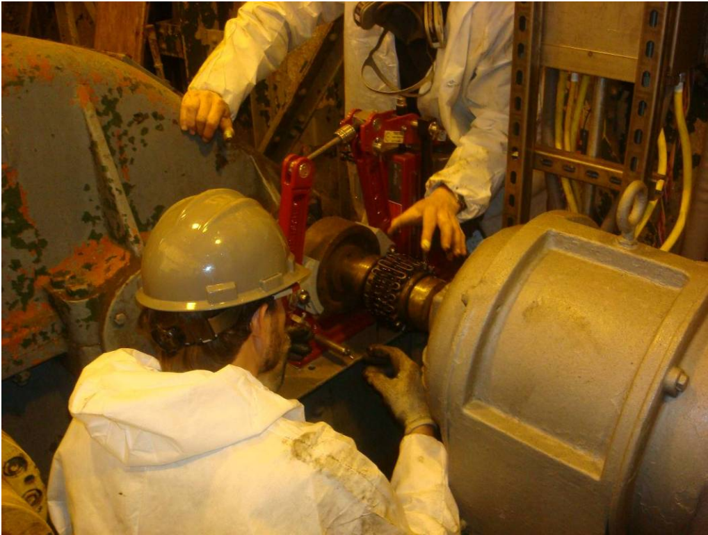
Photo 96: Final assembly of the machinery and motor coupler with the installation of the steelflex grid element between the motor and machinery in progress.
