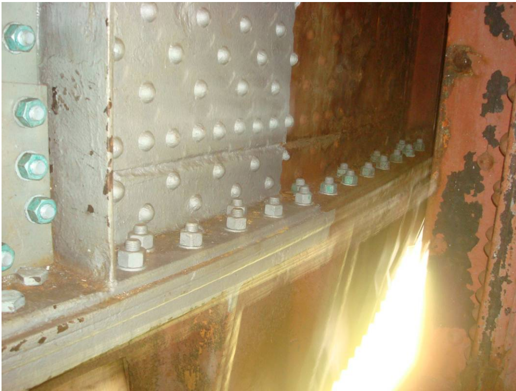
Photo 69: The Southwest girder rivet replacement between the girder bottom flange and the rack casting. Existing rivets have been replaced with 1" diameter H.S. bolts on the west side.
