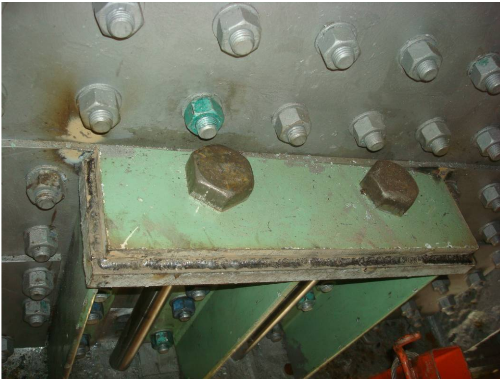
Photo 63: The West face of the East girder rack cap plate field welded to the rack stiffener. All four cap plate locations have been welded.
