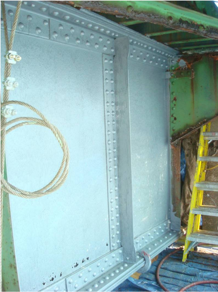
Photo 36: The Southwest girder elevation between the FB1 and FB2 primed with Epoxy Mastic Aluminum.
