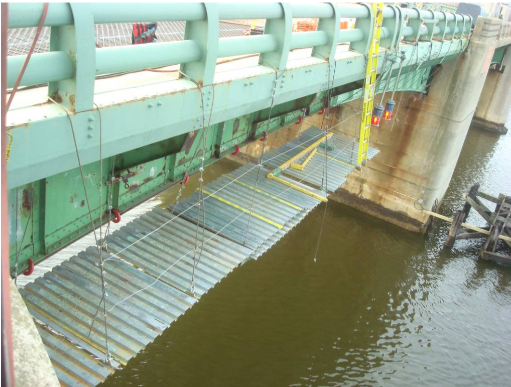
Photo 23: The painters began moving the east fascia temporary platform from the north leaf to the south leaf. Looking north from the control house.
