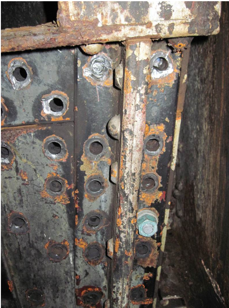
Photo 82: Removal of rivets at rear south leaf bascule girder in preparation for tie down installation.
