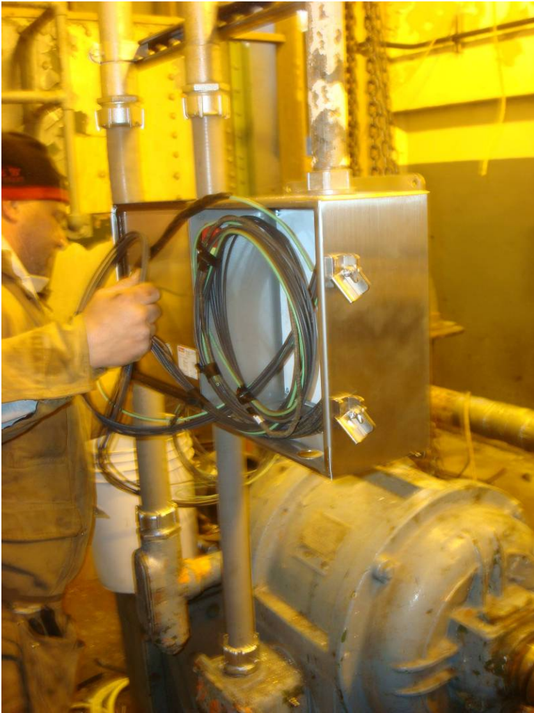
Photo 87: Installation of junction box for motor and machinery brake conductors in progress.
