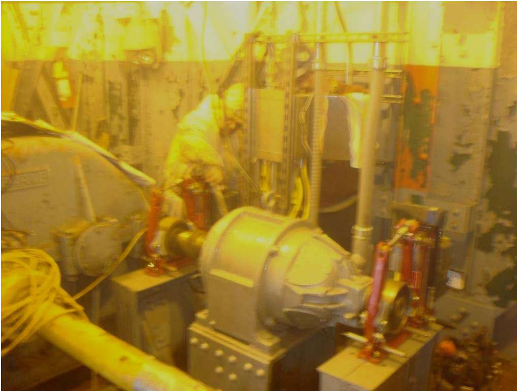
Photo 22: The motor and machinery supports have been painted with Epoxy Mastic Aluminum.
