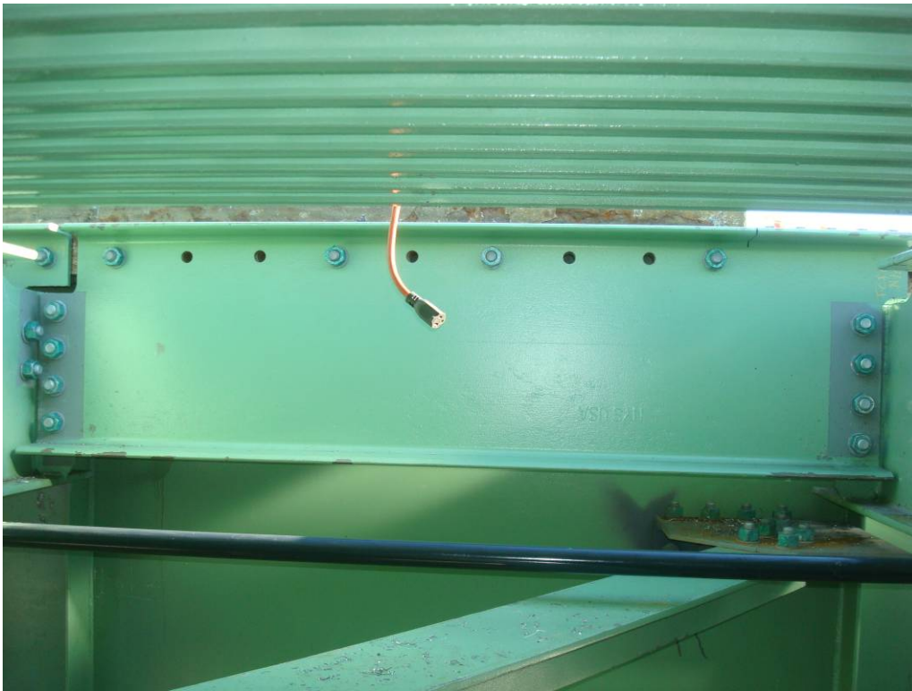
Photo 49: Diaphragm with field drilled holes in place to match the spacing in the casting of the toe joint.
