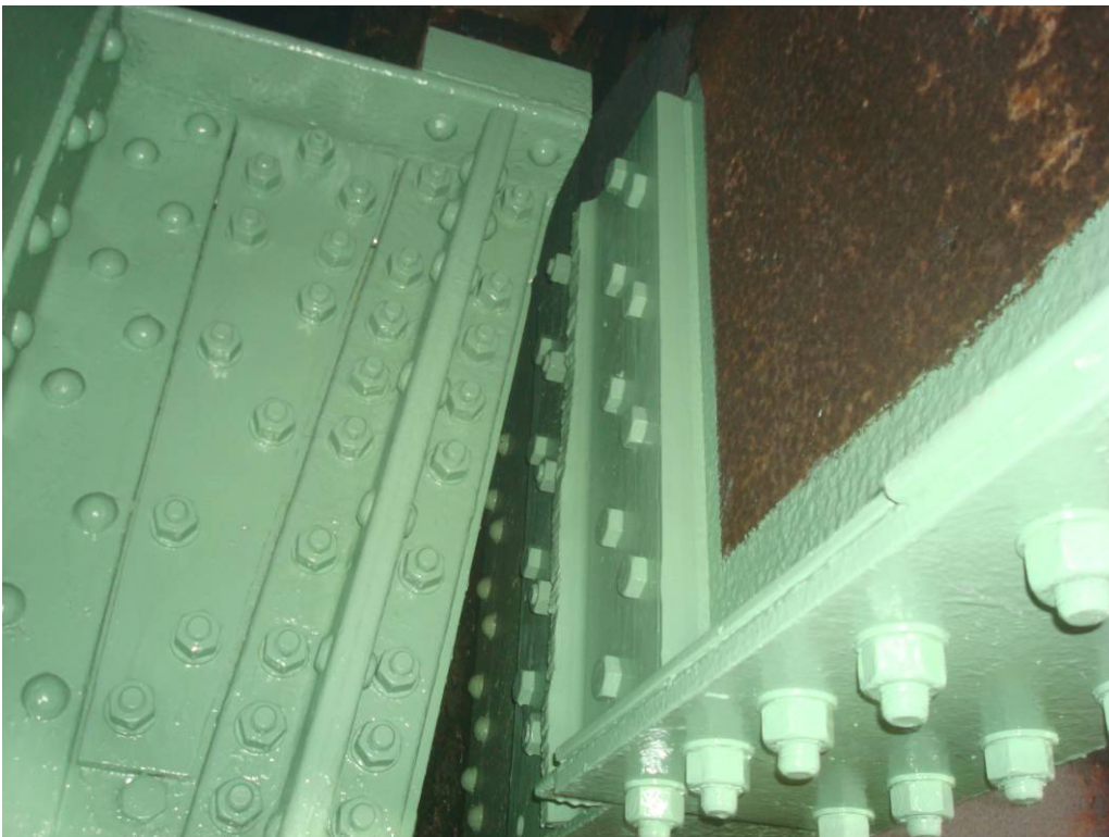
Photo 21: The application of the Acrolon 218 HS Acrylic Polyurethane finish coat on the existing live load bearing stiffener has been completed.
