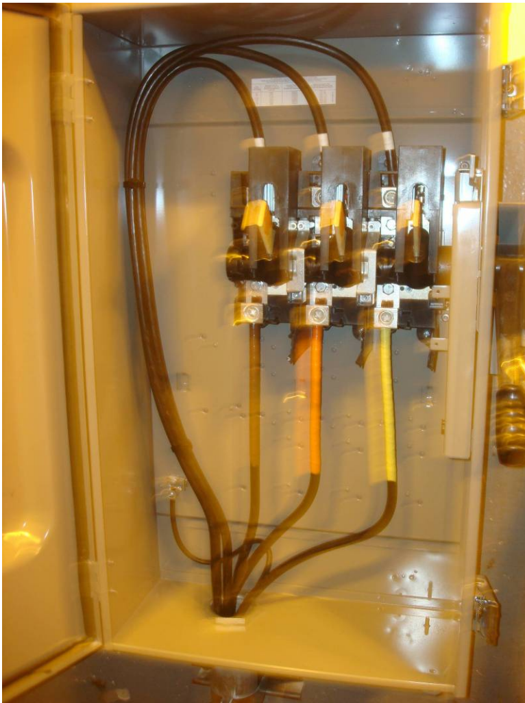
Photo 89: New shut off panel mounted for the span motor on machinery room wall has been wired.
