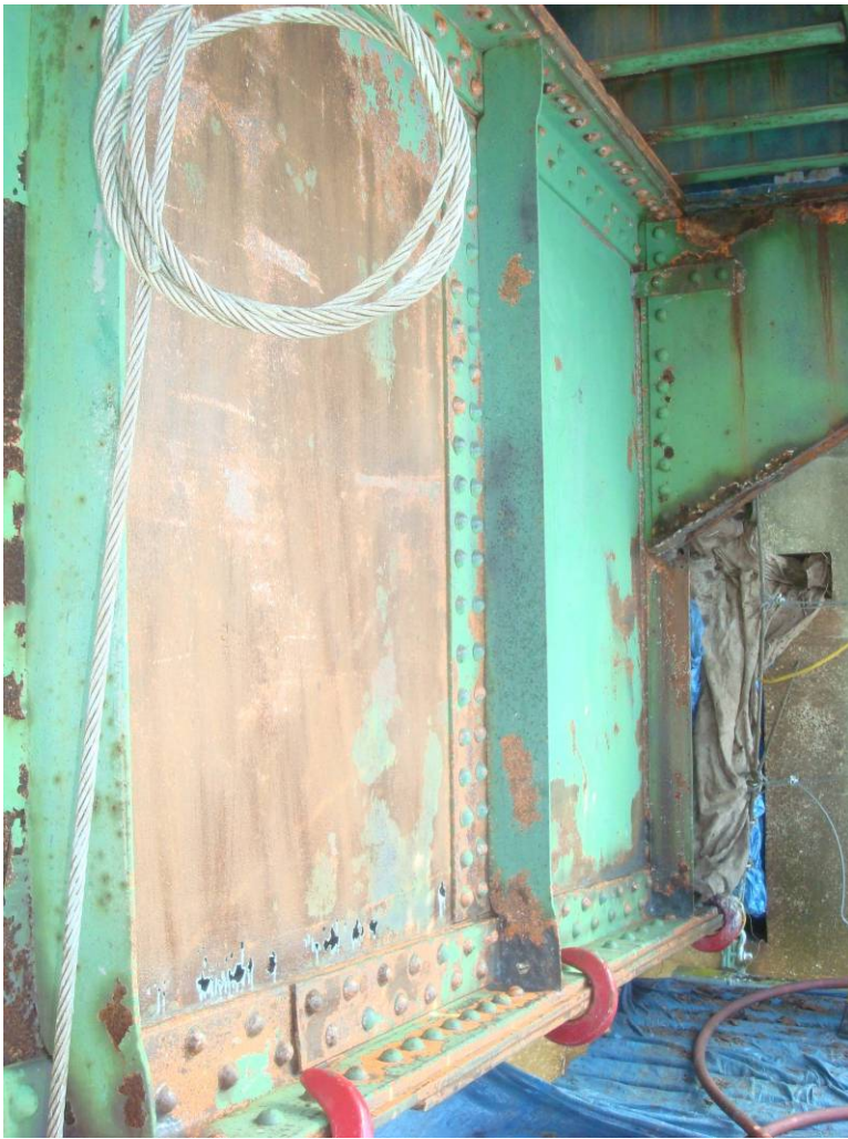
Photo 33: The Southwest girder elevation between the FB1 and FB2 cleaned with hand and power tools.
