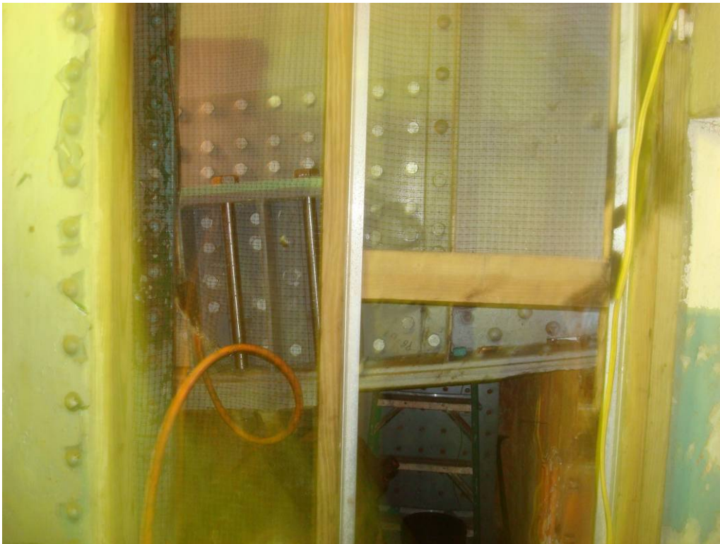
Photo 68: The Southwest girder (East face of girder) rack stiffener repair. Shims need to be completed.
