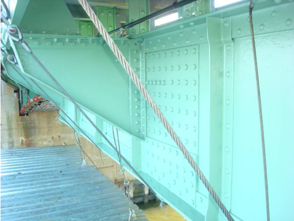
Photo 13: The painters primed the Southeast bascule girder and a portion of the rack at the trunnion area. East face shown.
