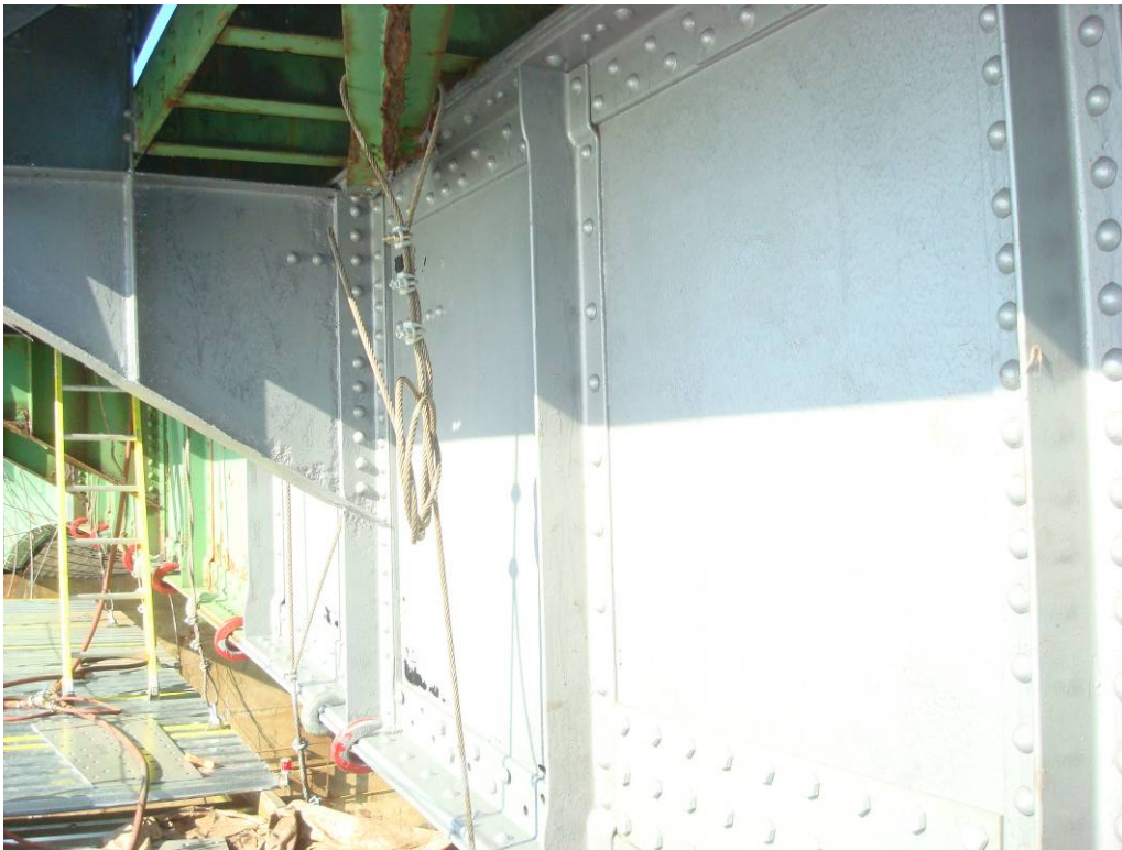
Photo 41: The Southwest girder elevation between the FB3 and FB4 and one girder panel towards FB2 primed with Epoxy Mastic Aluminum.
