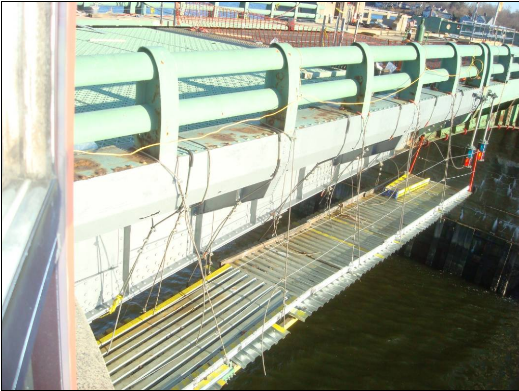
Photo 5: The painters primed the West fascia and touched up previously primed areas that were damaged due to the steel repairs.
