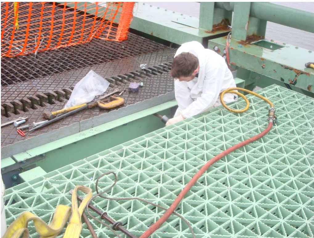
Photo 54: The ironworkers in progress of installing the H.S. bolts for the final section of the toe joint
