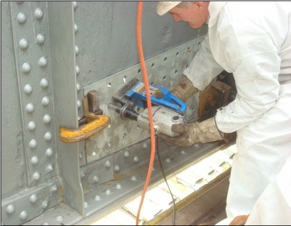
Photo 71: The Southeast girder repairs between the FB1 and FB2 in progress. Field drilling holes in the girder web using the repair plate as template.
