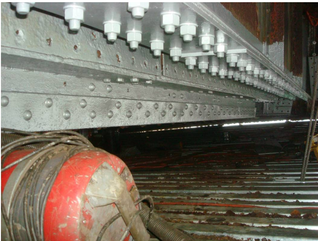
Photo 44: The south face of FB5 and Counterweight of the South leaf painted with Epoxy Mastic Aluminum primer.
