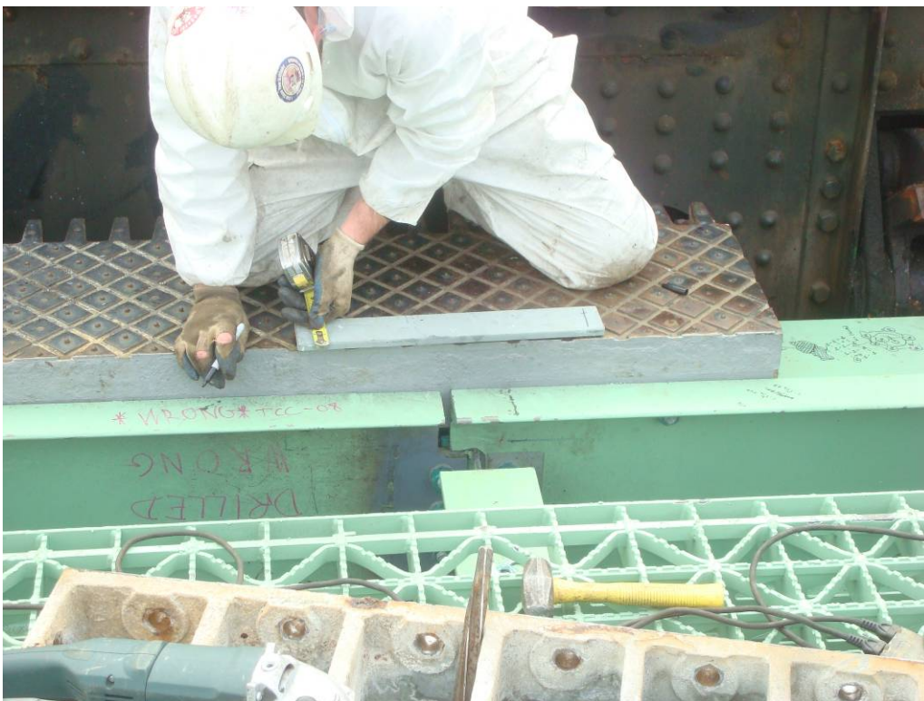
Photo 52: The ironworkers in progress of laying out the field drilled holes in the tie plate to match the hole spacing of the toe joint casting.
