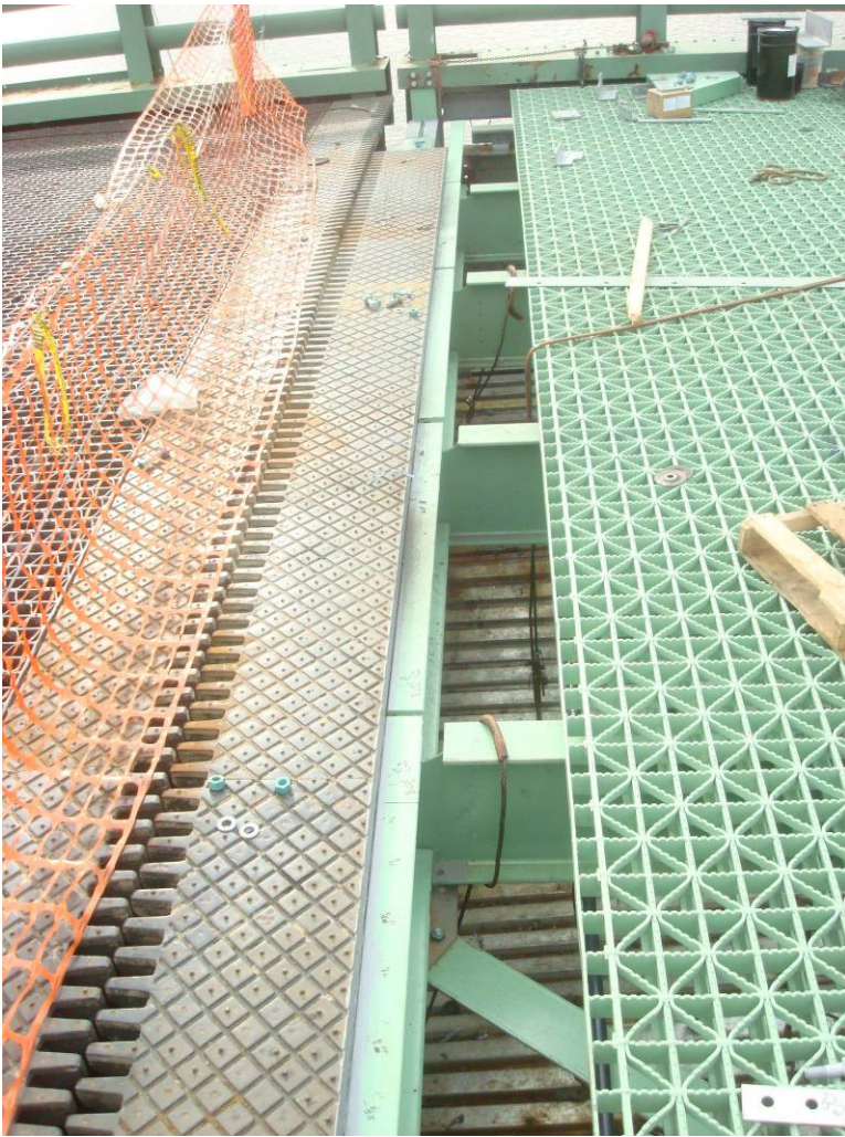
Photo 50: All but one section of the toe joint yet to be installed. All diaphragms installed except one between the stringer and the west girder.
