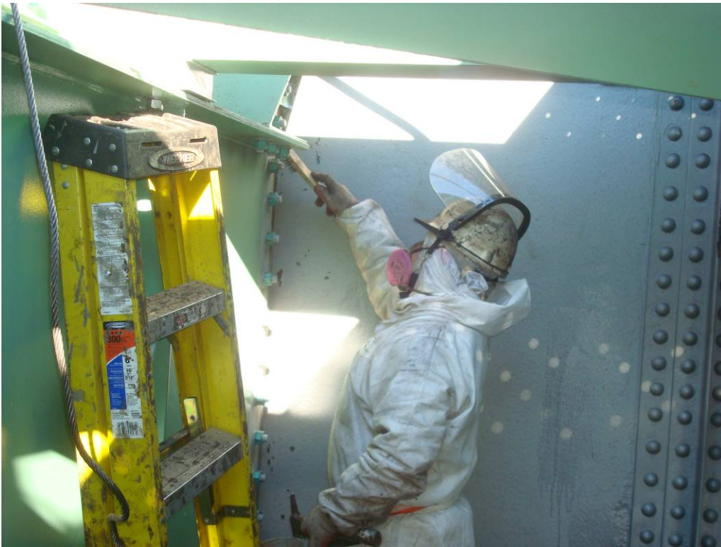
Photo 1: The painters were preparing the span for one final application of primer to the cleaned steel and touch up of previously primed steel.
