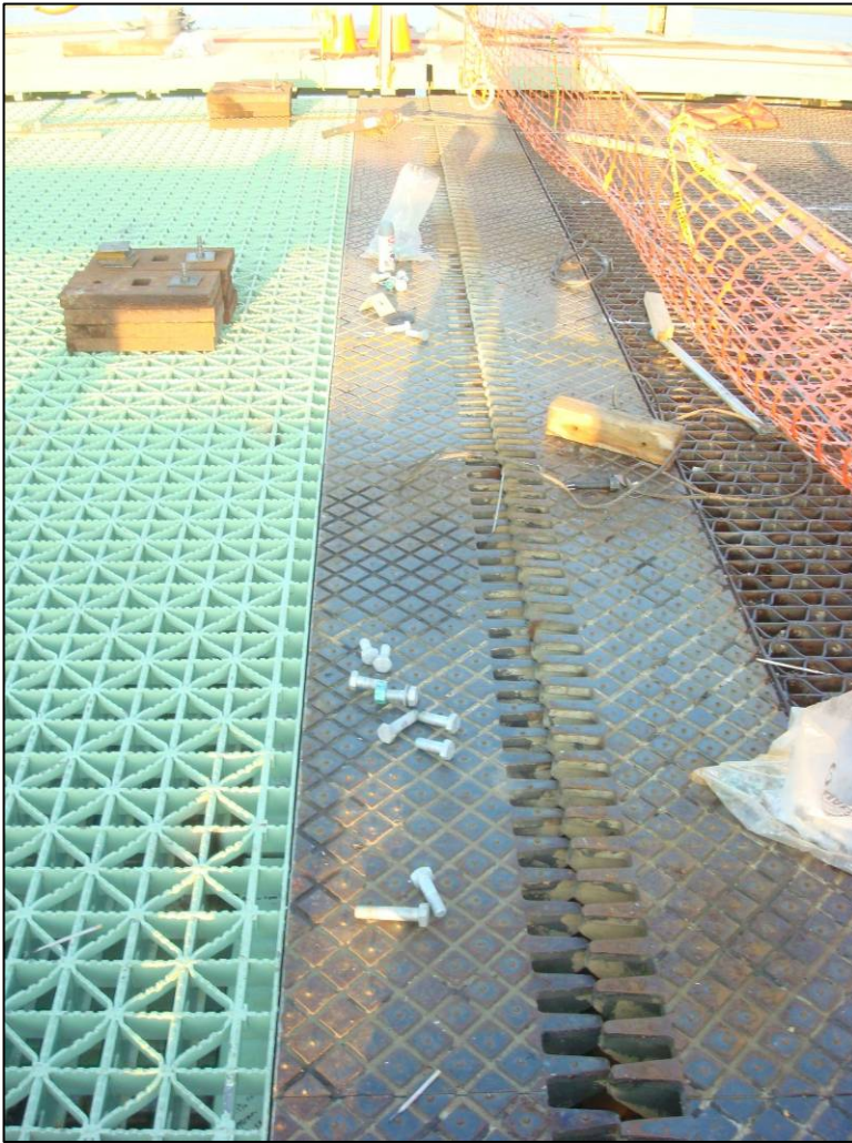
Photo 57: General Configuration. The toe joint is installed and the grating has been pushed into final position.
