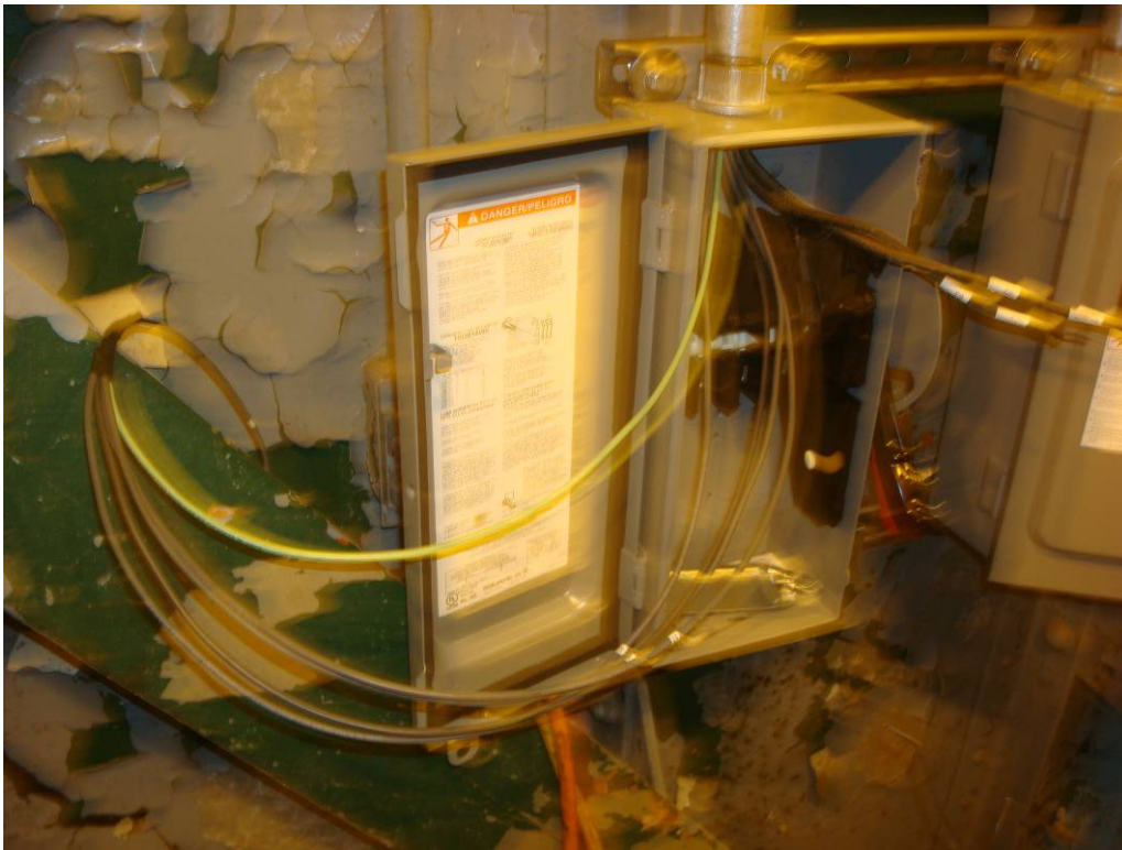
Photo 88: Wiring of machinery brake switch panel in progress.
