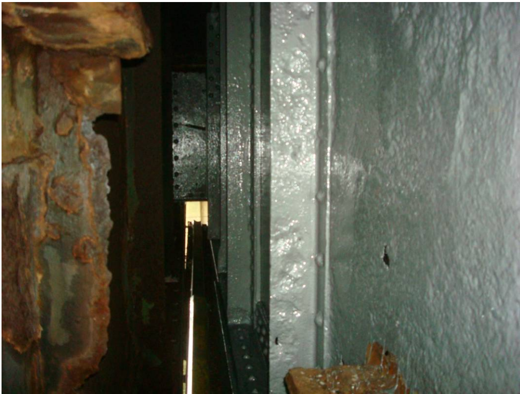
Photo 43: The East face of the Southeast bascule girder looking towards FB5 of the South leaf painted with Epoxy Mastic Aluminum primer.
