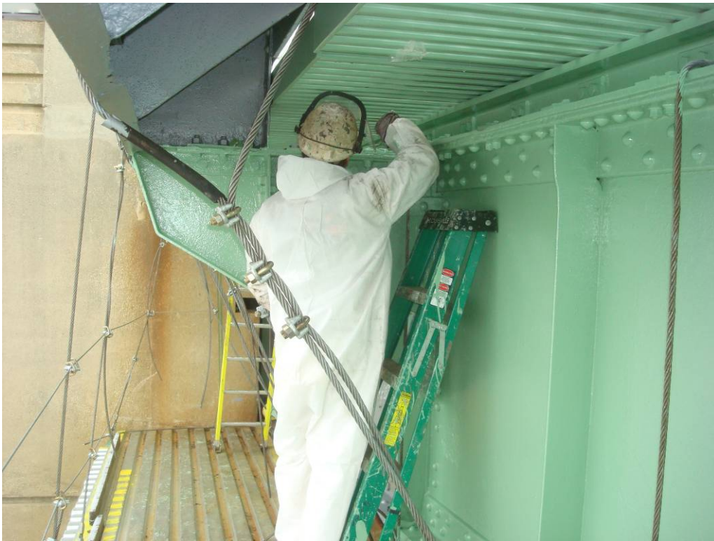
Photo 14: The application of the Acrolon 218 HS Acrylic Polyurethane finish coat in progress on the West bascule girder elevation.
