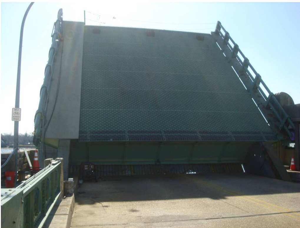
Photo 99: North Leaf opened on Tuesday 2/28/12. Note that the Final section of grating was also installed.
