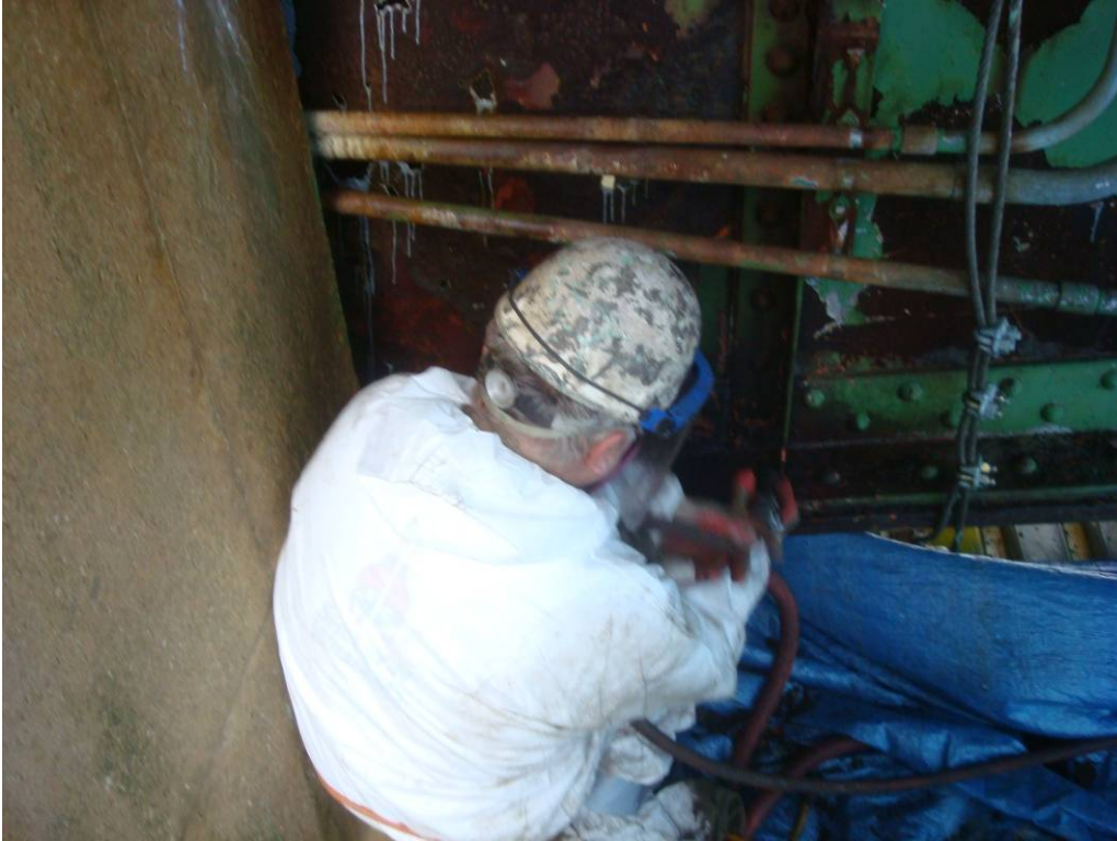
Photo 25: The Painter cleaning the bottom flange of the East girder near FB4 on the South leaf.
