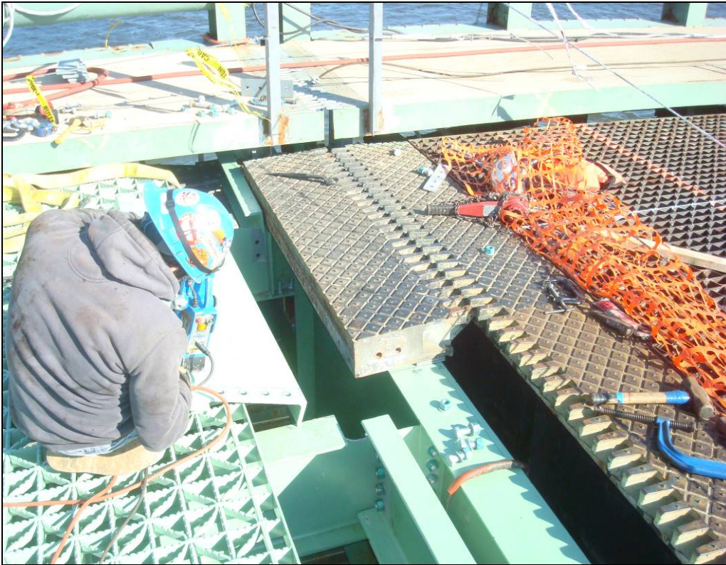
Photo 47: Field drilling of the diaphragm to match the existing hole spacing in the toe joint casting.
