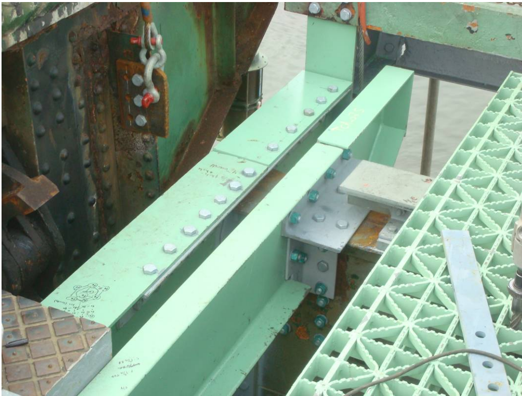
Photo 53: The final section of the toe joint diaphragm and cantilevered deck support installation completed.
