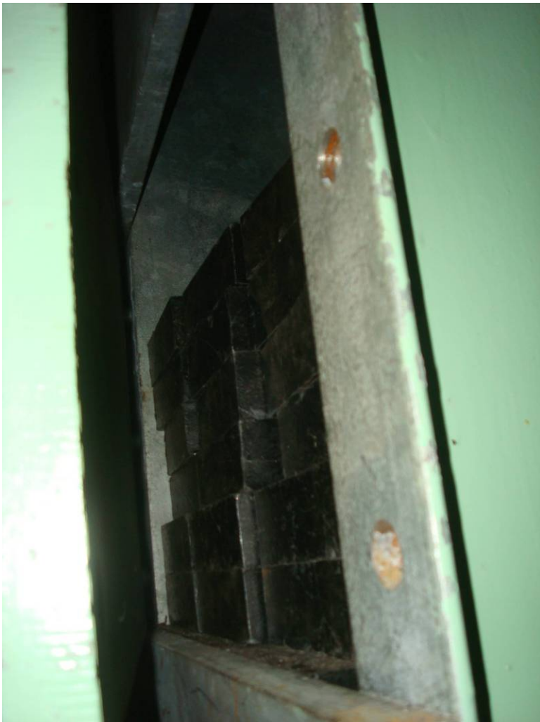
Photo 79: General configuration of the lead ballast blocks in the Northwest pocket installed.
