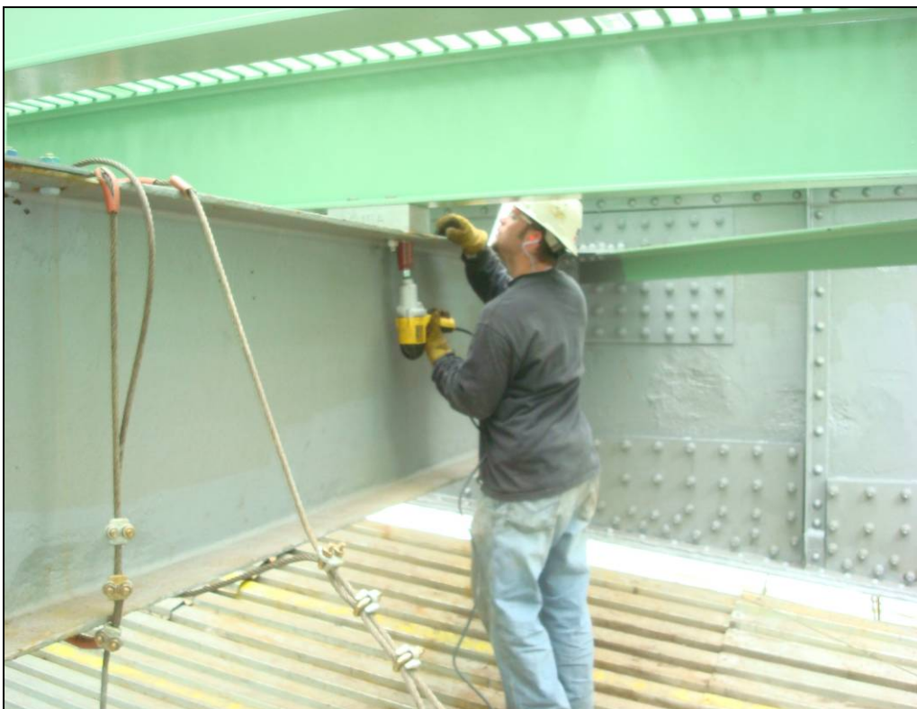
Photo 59: The iron workers are in progress of performing the final tightening of the connections between the stringer and floorbeam on the north bascule span.
