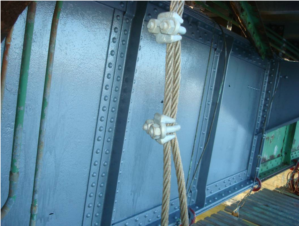
Photo 29: The East girder elevation looking at FB3 of the South leaf primed with Epoxy Mastic Aluminum.
