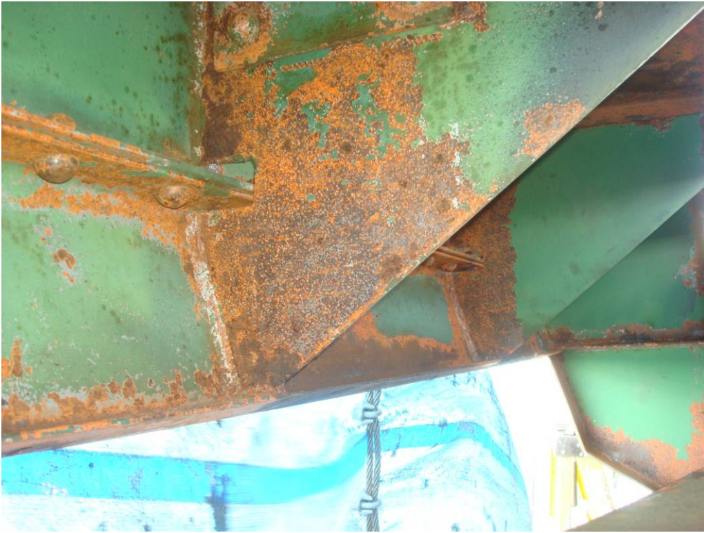
Photo 39: The Southeast girder underside of fascia between the FB3 and FB4 cleaned with hand and power tools looking North.
