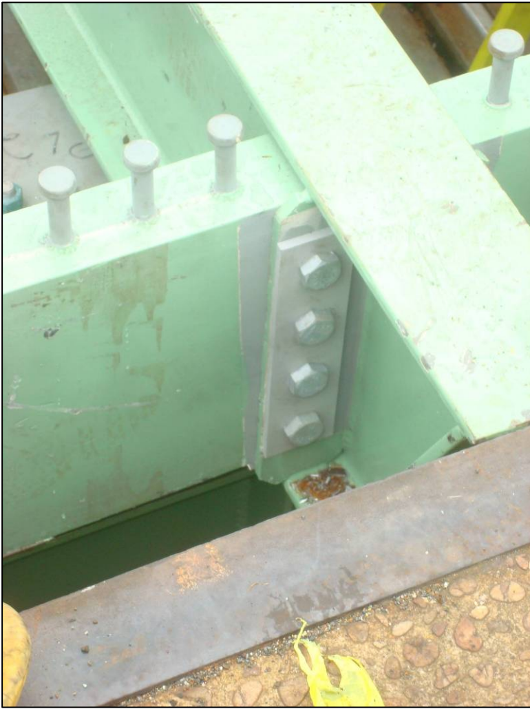
Photo 60: Cover plate installed over the section of mis-aligned holes of stringer connection plates to the diaphragms.
