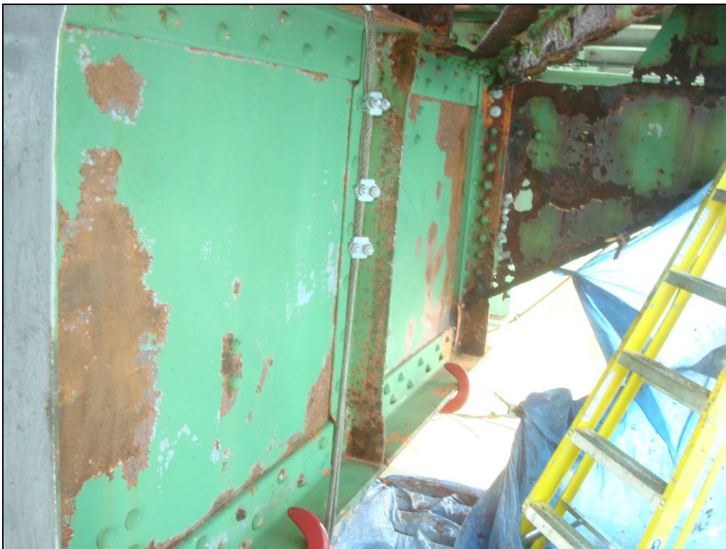
Photo 31: The Southeast girder elevation between the FB1 and FB2 cleaned with hand and power tools.
