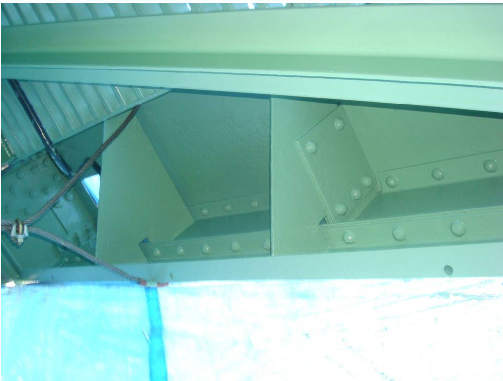
Photo 17: The application of the Acrolon 218 HS Acrylic Polyurethane finish coat in progress on the West bascule girder elevation.
