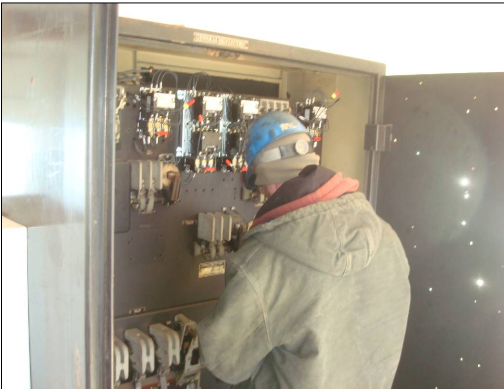
Photo 94: Ongoing electrical work and testing in progress.
