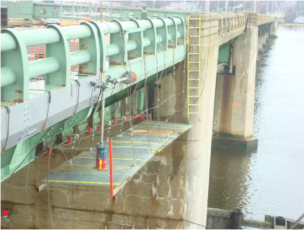
Photo 24: The west fascia temporary platform has been removed from the north leaf and installed onto the south leaf.
