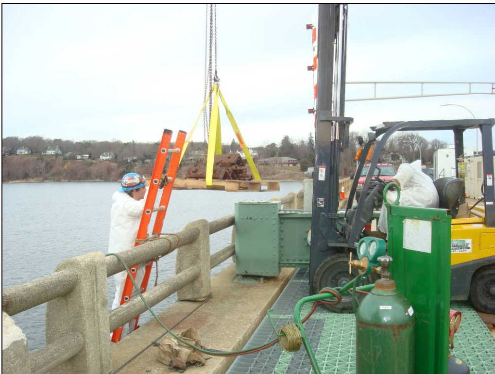
Photo 74: Removal of steel ballast plates in progress.
