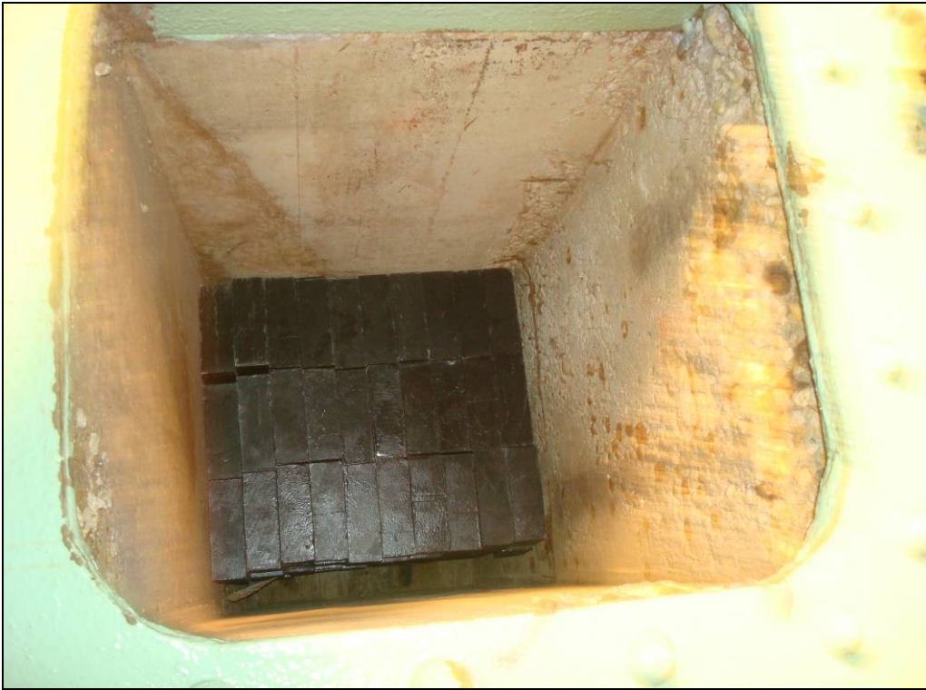
Photo 77: New lead brick in the west counterweight pocket in progress.
