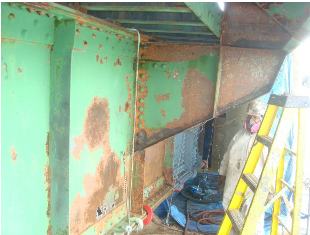
Photo 38: The Southwest girder and cantilevered bracket at FB3, looking South, cleaned with hand and power tools.
