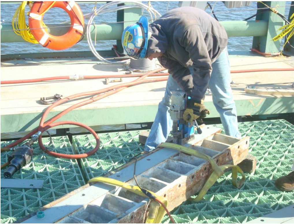
Photo 45: Field drilling of the shim to match the spacing of the existing holes of the toe joint.
