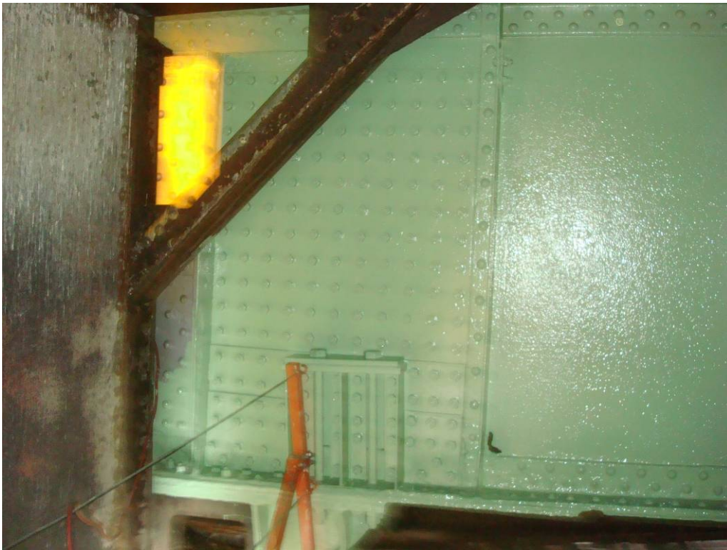
Photo 18: The application of the Acrolon 218 HS Acrylic Polyurethane finish coat on the West bascule girder at the east face of the rear rack has been completed.
