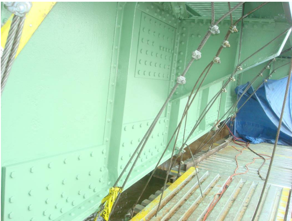
Photo 15: The application of the Acrolon 218 HS Acrylic Polyurethane finish coat in progress on the West bascule girder elevation.
