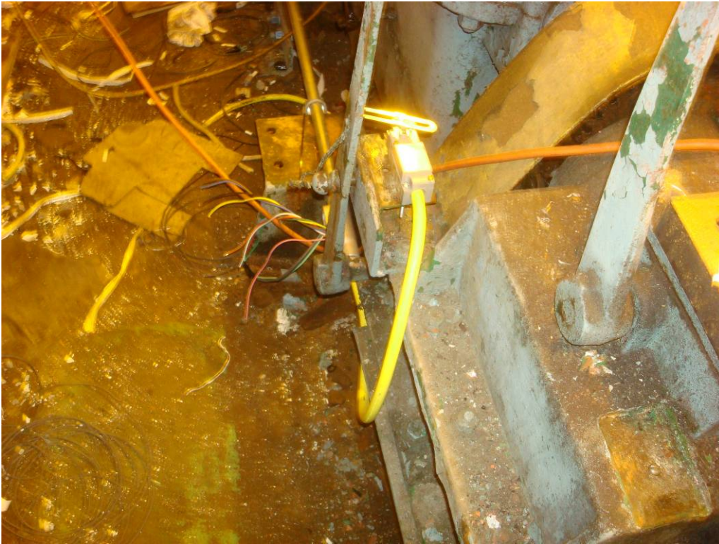
Photo 93: The wiring for the limit switch for the reverser drive is in progress.
