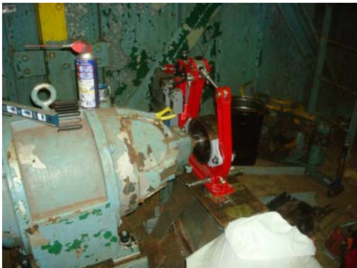
Installation of the motor brake in progress.
