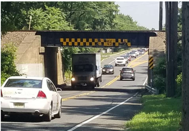
Photo 2 - NJ Transit Railroad Bridge (looking south)
