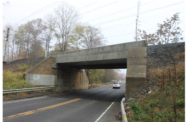
Photo 2 - 2022 Emergency Superstructure Repair (looking north)
