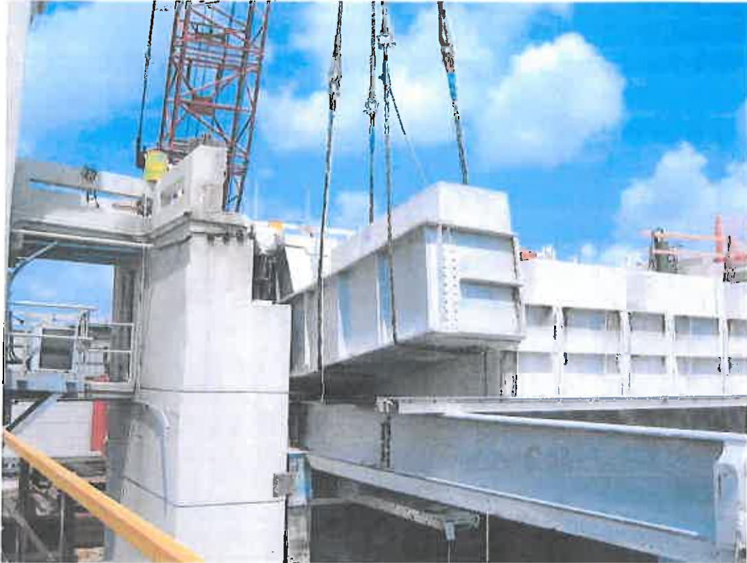
Figure 4: Counterweight section being removed.
