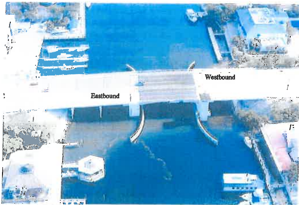
Figure 1: PGA Blvd. Bascule Bridge
