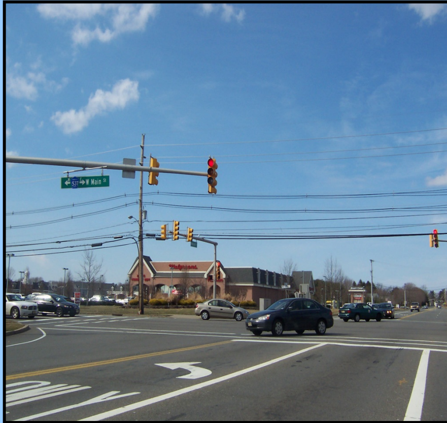
Route 537 & Wemrock Road/Stillwells Corner Road Intersection, Site of higher than average crash rates and failed traffic operations (LOS F) at peak periods
