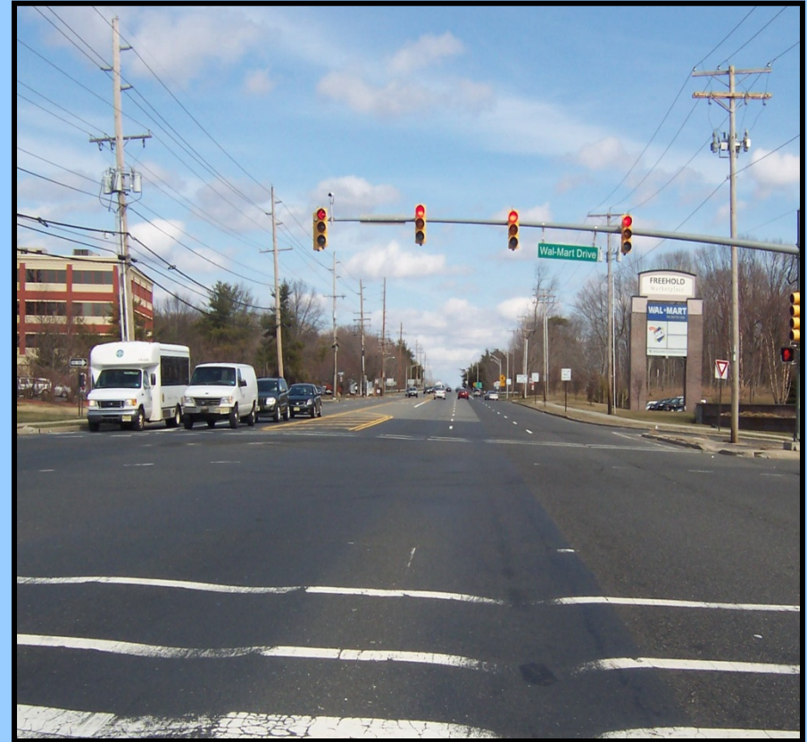
Wal-Mart Drive Intersection, No Bicycle Compatibility, Gaps in sidewalk network, no auxiliary lanes for turning movements
