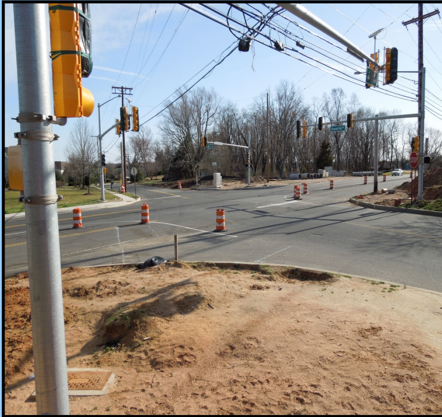
On-going Improvements at Route 537 & Gravel Hill Road Intersection
