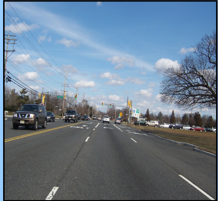
Eastbound Approaching Trotter's Way intersection (access to Freehold Raceway Mall), Site of higher than average accident rates
