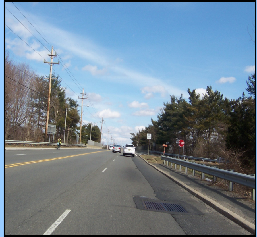
Looking East Approaching Bridge over Route 33 Freeway, Site of higher than average crash rates, substandard acceleration & deceleration lanes, gaps in sidewalk network, no bicycle compatibility, substandard vertical curve
