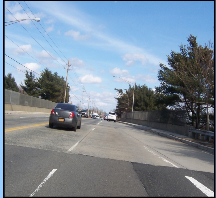
Route 537 Bridge over Route 33 Freeway – No sidewalk on Westbound Side, No Bicycle compatibility
