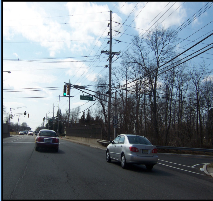
Looking Westbound Approaching bridge over Route 9, Interchange Operates in Failed Condition (Level of Service F) resulting in traffic congestion and delays during peak periods, No dedicated turning lanes, No bicycle compatibility, No sidewalk on Eastbound Side
