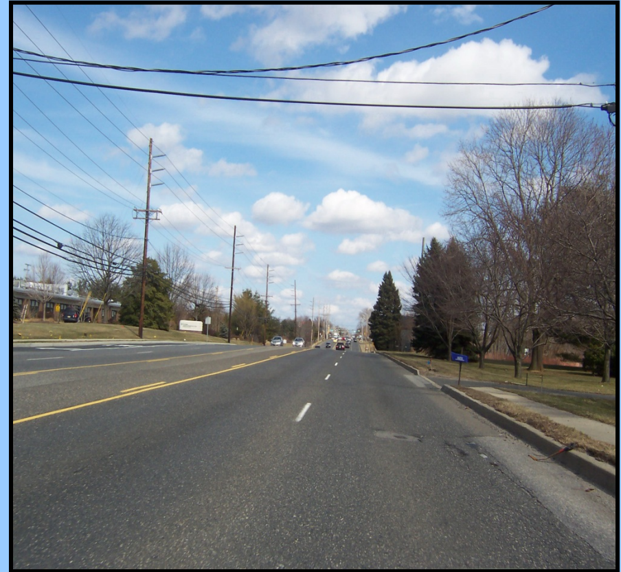
Looking East, Approaching Redwood Lane/Village Center Road, Note Substandard vertical curve (WB), Sidewalk gaps, No Bicycle Access
