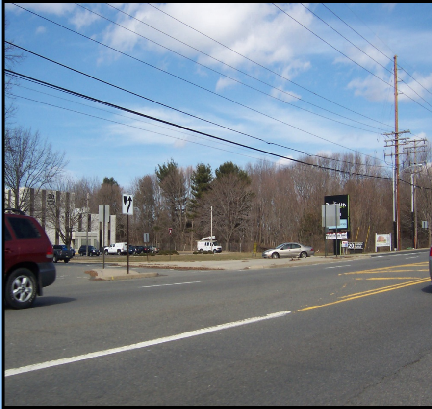
Rt.537 & Gibson Place Un-signalized Intersection, Site of higher than average crash rates and failure of traffic operations at peak periods
