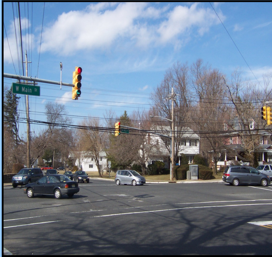
Route 537 & Route 9 Business Intersection, Site of failed traffic operations (LOS-F) during peak periods resulting in congestion and delays
