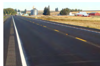
Shoulder rumble strips and center line rumble stripes are installed on this roadway. Source: FHWA
