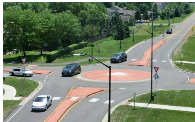
Example of a single-lane roundabout. Source: FHWA
