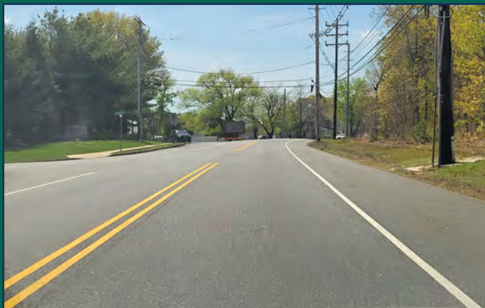
COUNTY ROUTE 17-II AT LOUISVILLE ROAD
