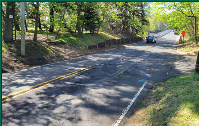
COUNTY ROUTE 8-A AT LINDEN AVENUE, MIDDLETOWN
