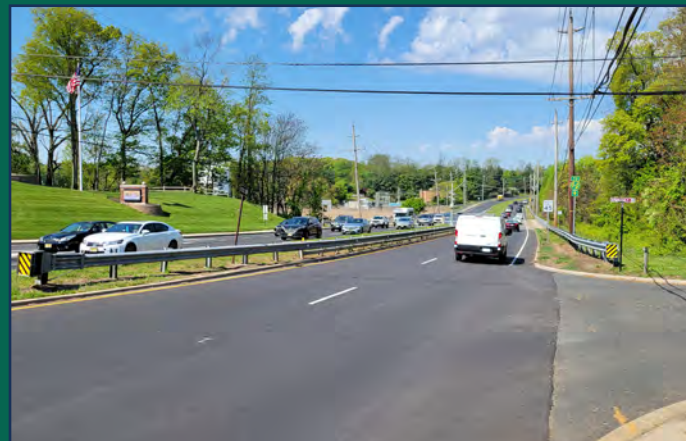
COUNTY ROUTE 520 CROSSING THE NAVESINK RIVER
