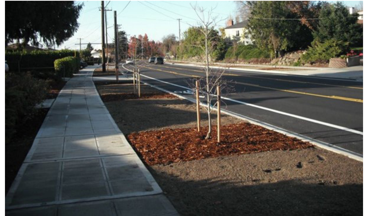
Figure 5: Wide sidewalks with a generous buffer provides a more pleasant walking experience. Buffer areas like the one shown in this photo can be used for other community-enhancing amenities such as street trees, landscaping, and green storm water management. (Image Source: NACTO)
