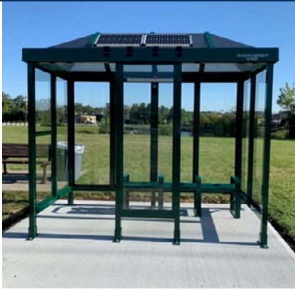
Figure 15: NJ TRANSIT's new solar-powered shelters have lighting and charging ports for electronic devices. (Image Source: NJ TRANSIT)
