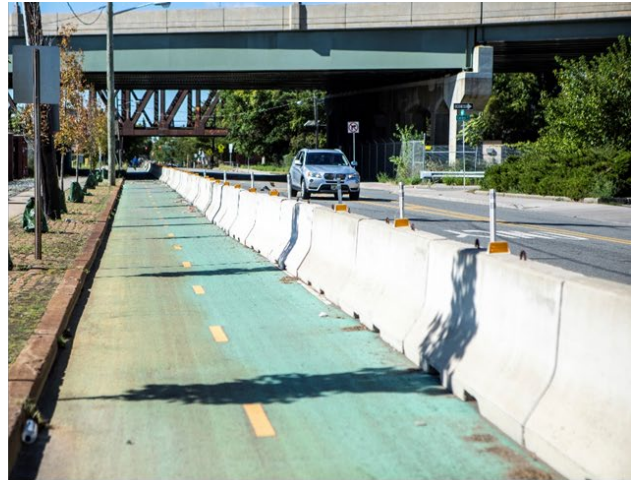
Cycle Track protected by Jersey Barrier
