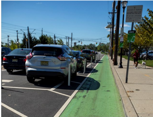
Parking-Protected Directional Bike Lane
