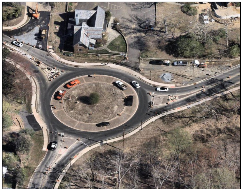
New Roundabout on County Route 8A/8B in Middletown
