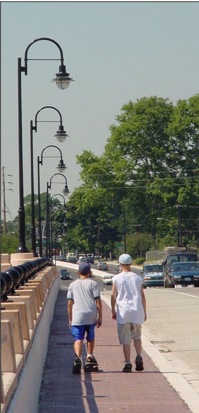
Cooper's Bridge in Red Bank
