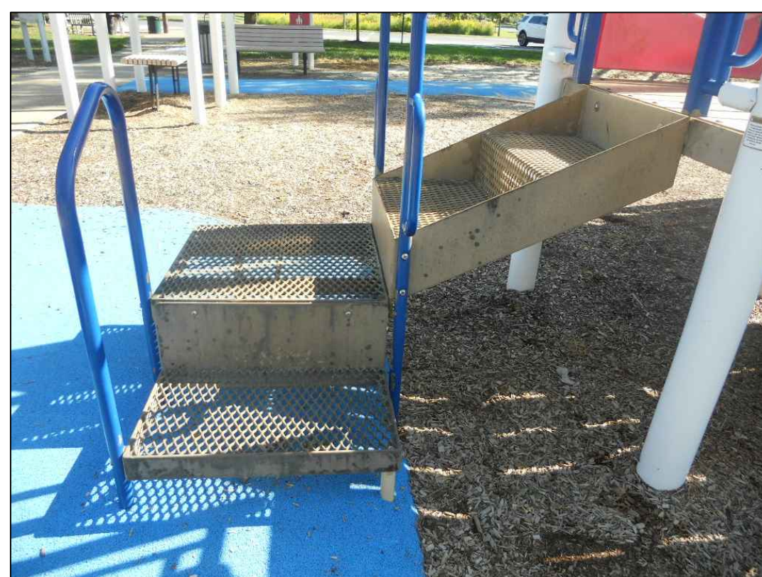
Mold and dirt on platforms and stairs.
