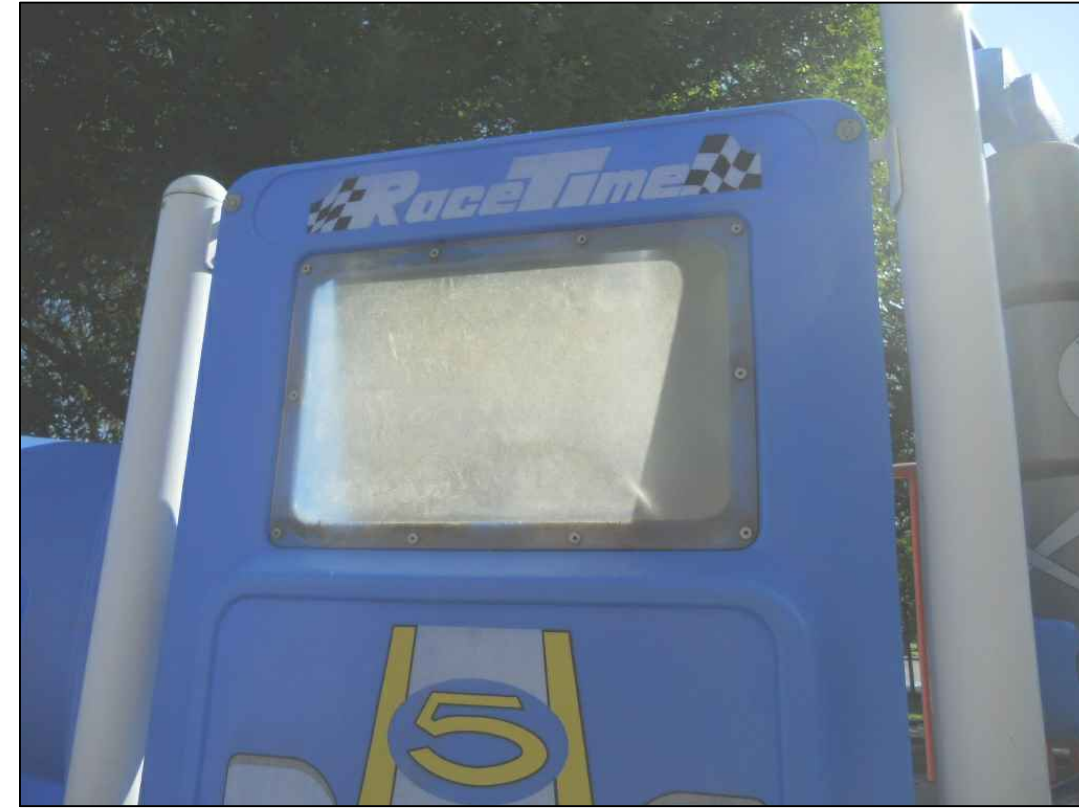
Replace clear view panel with new.
