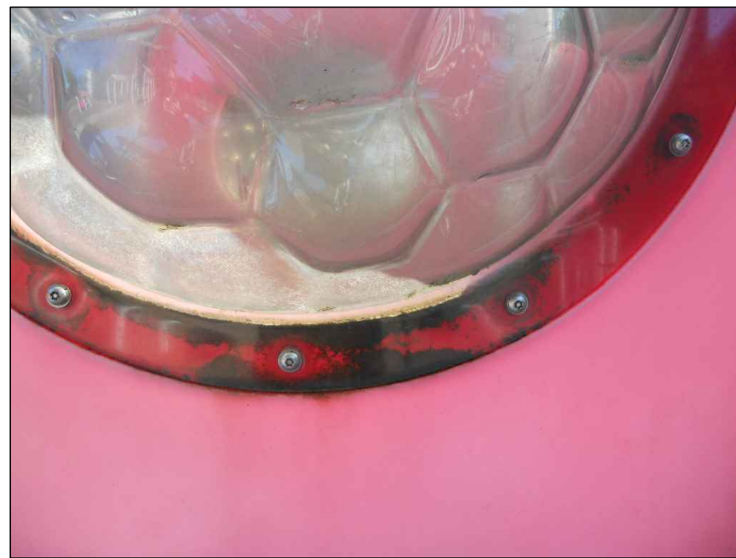
Remove panels, clean mold & dirt on both surfaces and reinstall panels.
