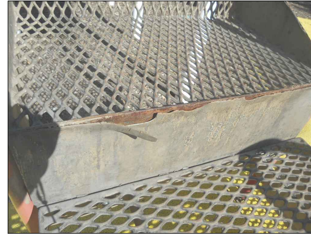
Repair thermoplastic coating of composite structure stairs and platforms
