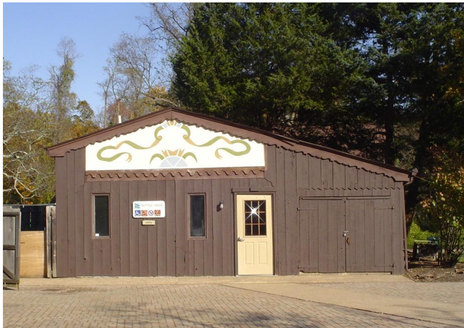
Reptile House, existing condition.
