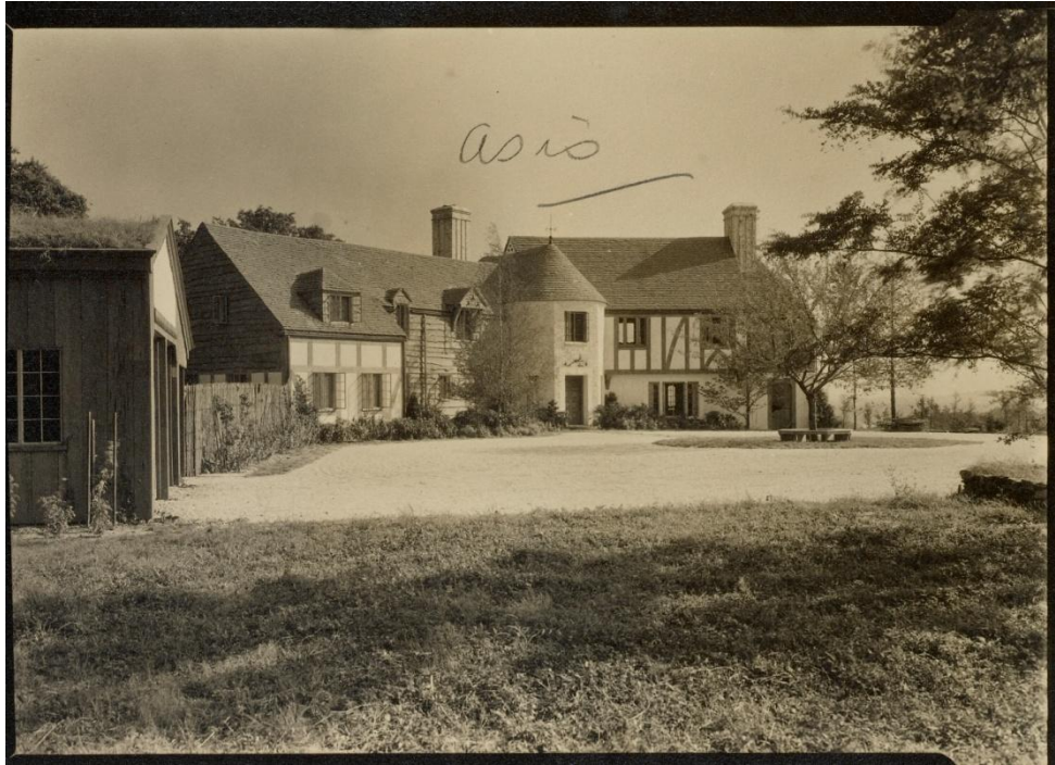
Hans Huber House and Garage, 1930. Edwin L. Howard, Architect.
