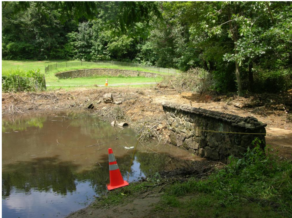
Figure 15 photo: pond head wall and retaining wall in background
