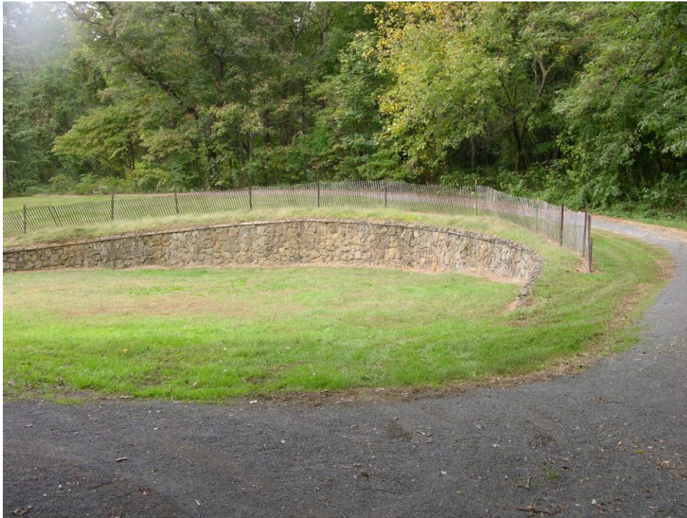
Figure 16 photo: retaining wall
