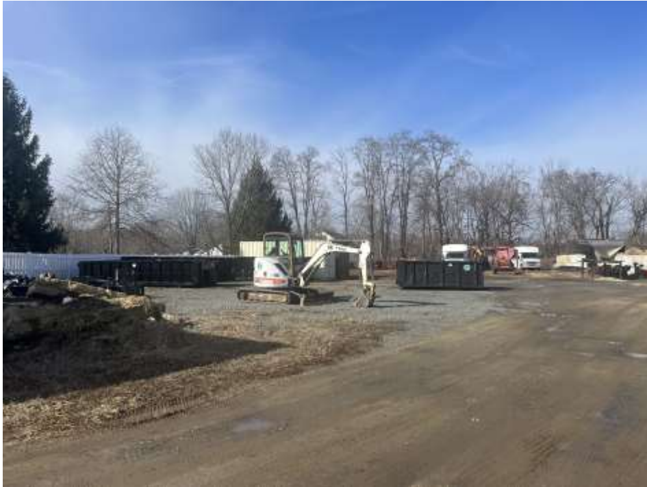
View looking northwest from the Thompson Park maintenance yard (February 2025)
