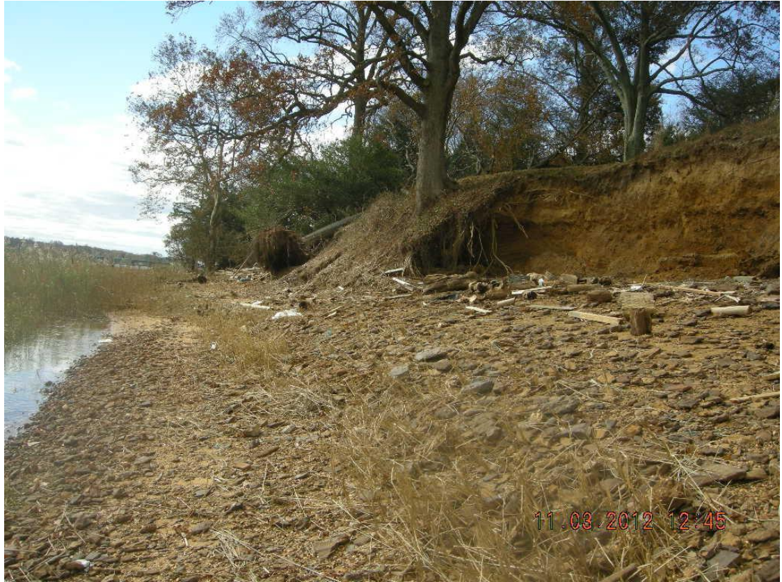
Figure 5 Shoreline Looking West October 30, 2013
