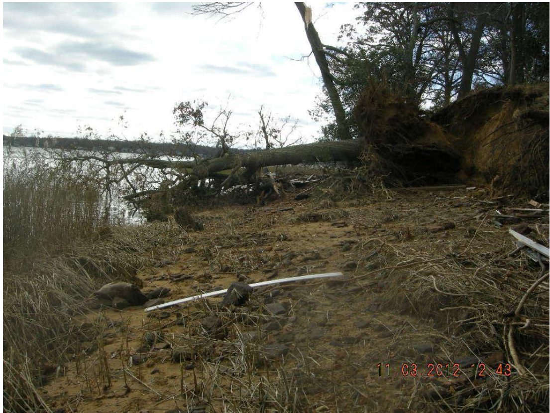
Figure 6 Shoreline looking West October 30 2013
