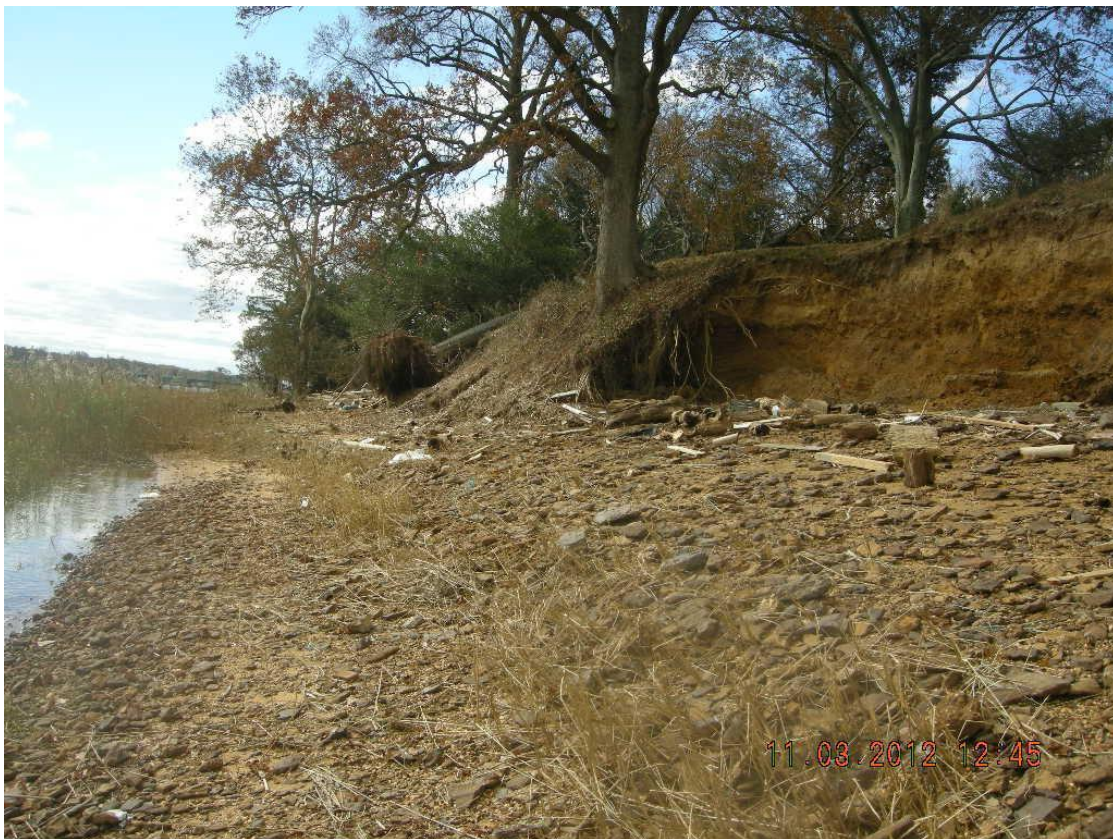
Figure 13 Shoreline Looking West October 30, 2013
