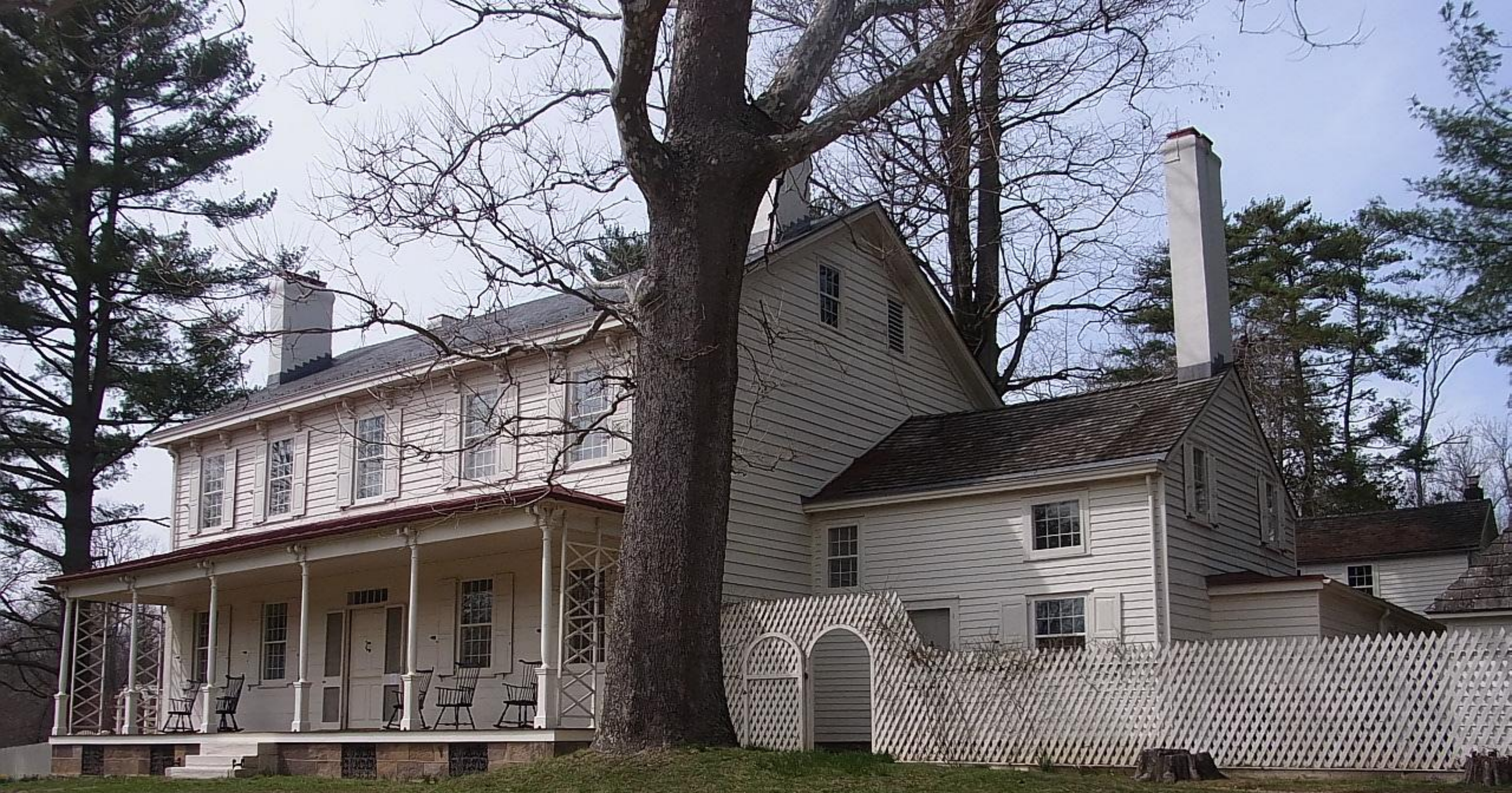
Bldg #1704 and Bldg #1720 Main Dwelling and Caretaker's Wing Historic Walnford
