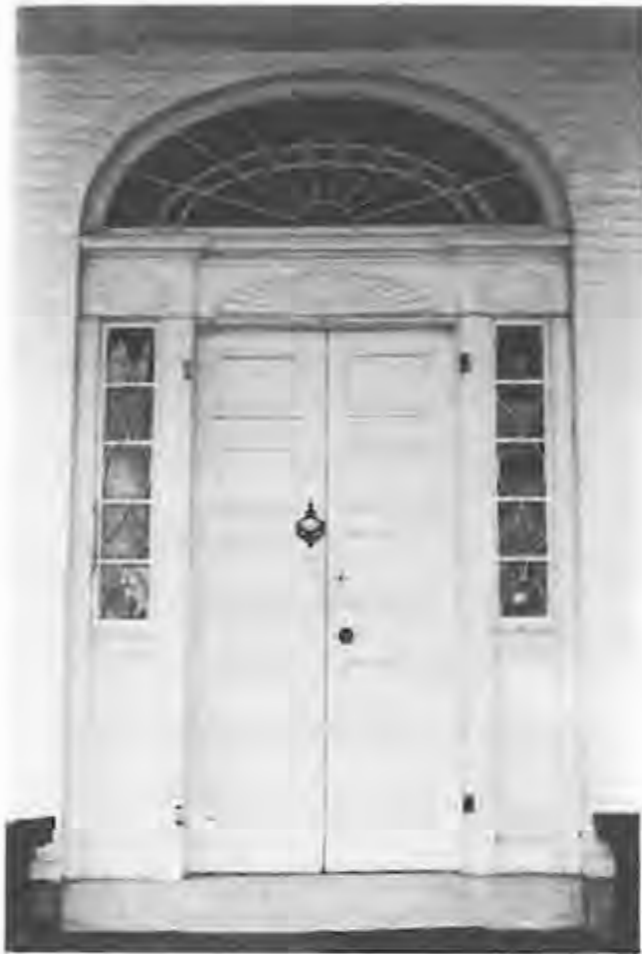
Doorway on the Samuel Wright House in Upper Freehold, built 1810. (MCHSI 1351-50)
