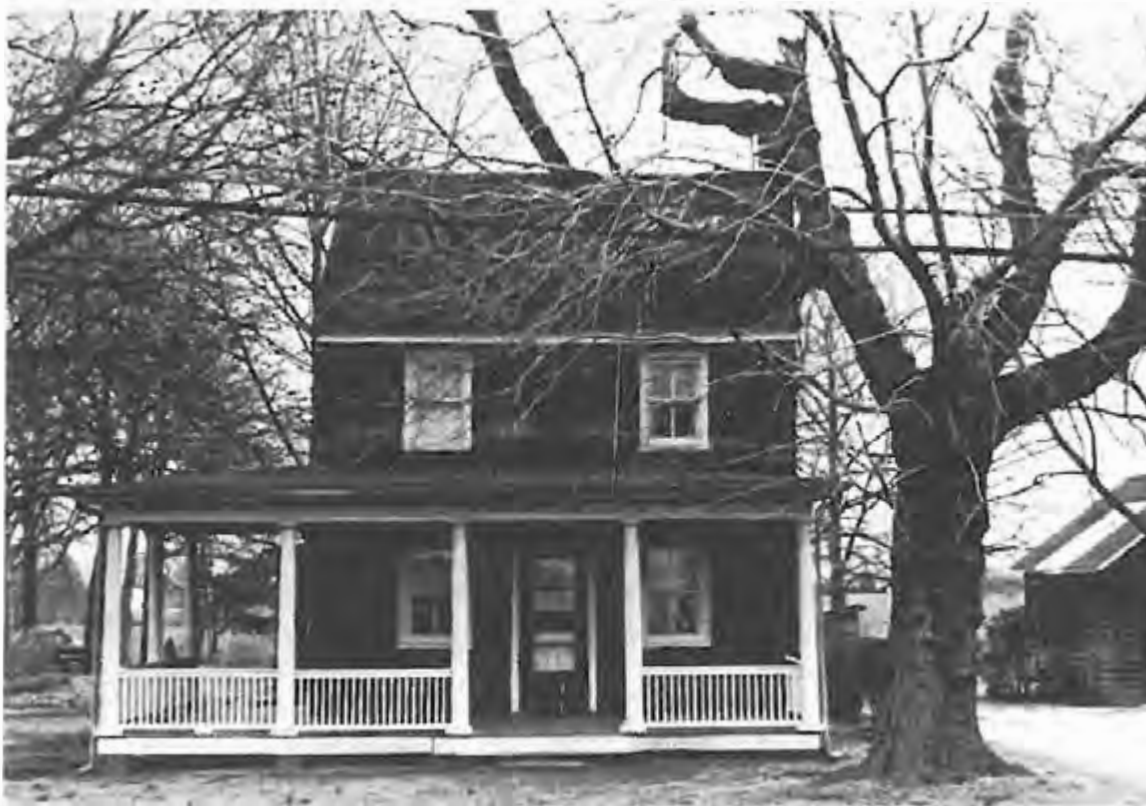
This center door house, located on the old Burlington Path in Freehold Township, probably dates from the late 18th/early 19th century. It is wood shingled with a fieldstone foundation; earlier 6/6 sash windows are visible on the sides. The porch is a later addition. (MCHSI 1316-16)
