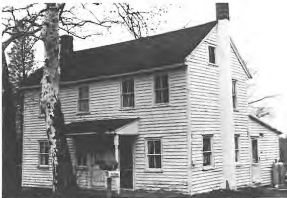
I-house with asymmetrical four over five bay facade, built early 19th century. Upper Freehold Township (MCHSI 1351-69).
