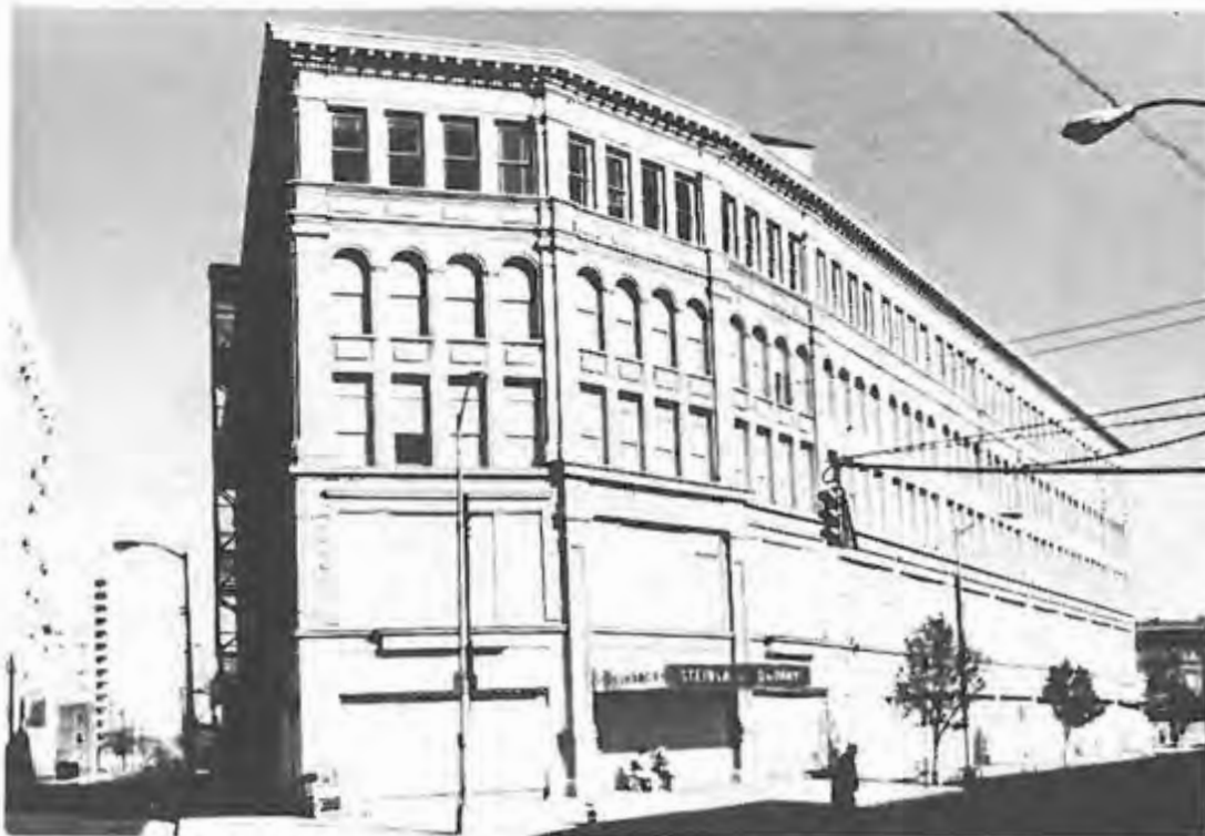
Steinbach's Department Store in Asbury Park, built 1897 with early 20th century additions. (MCHSI 1303-8)
