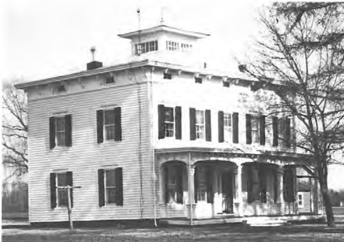
The J.W. Burtis House in Upper Freehold (MCHSI 1351-3). The simple cubic form of this 1850's Italianate residence is enhanced by the cupola, wide bracketed cornice, ornate pilastered doorway, and full porch.
