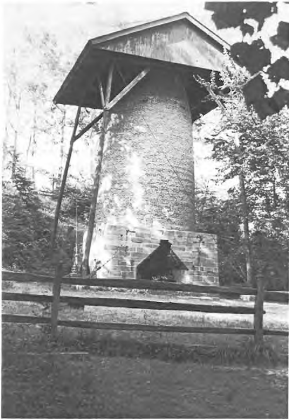
Furnace, Howell Works. Wall Township. (MCHSI 1352-1)
