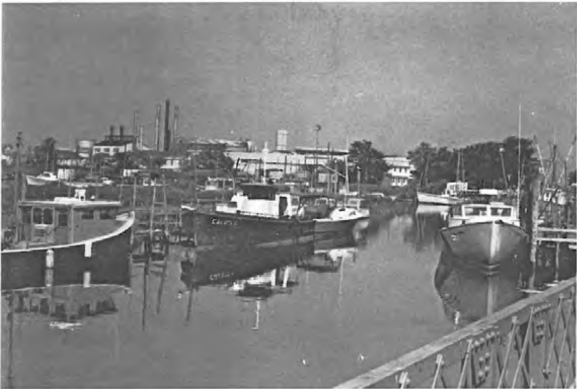
Shoal Harbor, Belford, Middletown Township. (MCHSI 1331-6)
