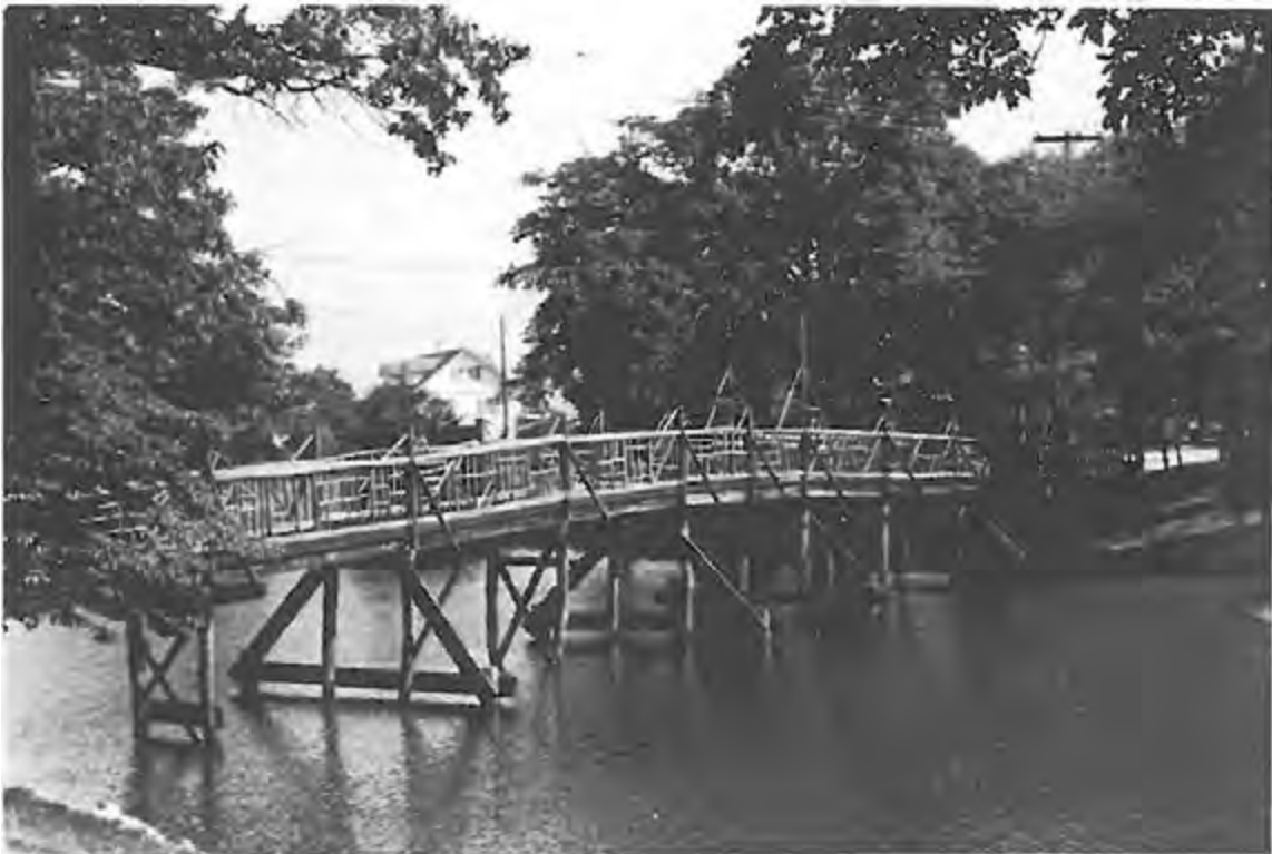
Rustic wooden footbridge over Spring Lake in Spring Lake Borough. (MCHSI 1348-38).
