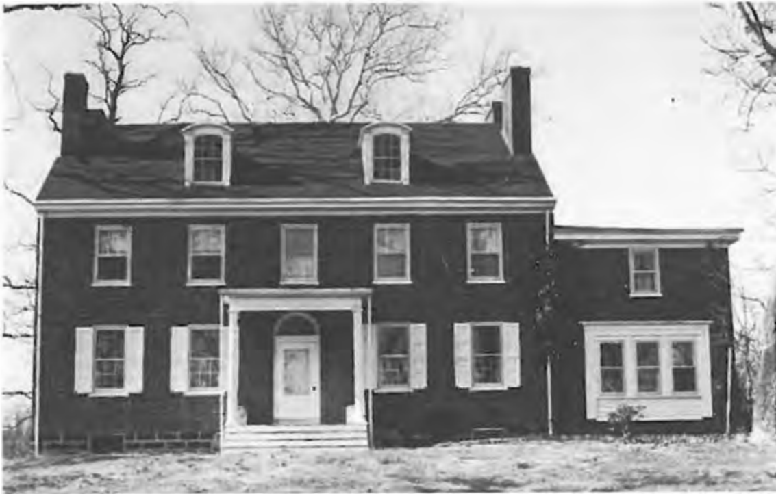
Robert Woodward House, built c. 1815-1830, Upper Freehold Township. (MCHSI 1351-37)
