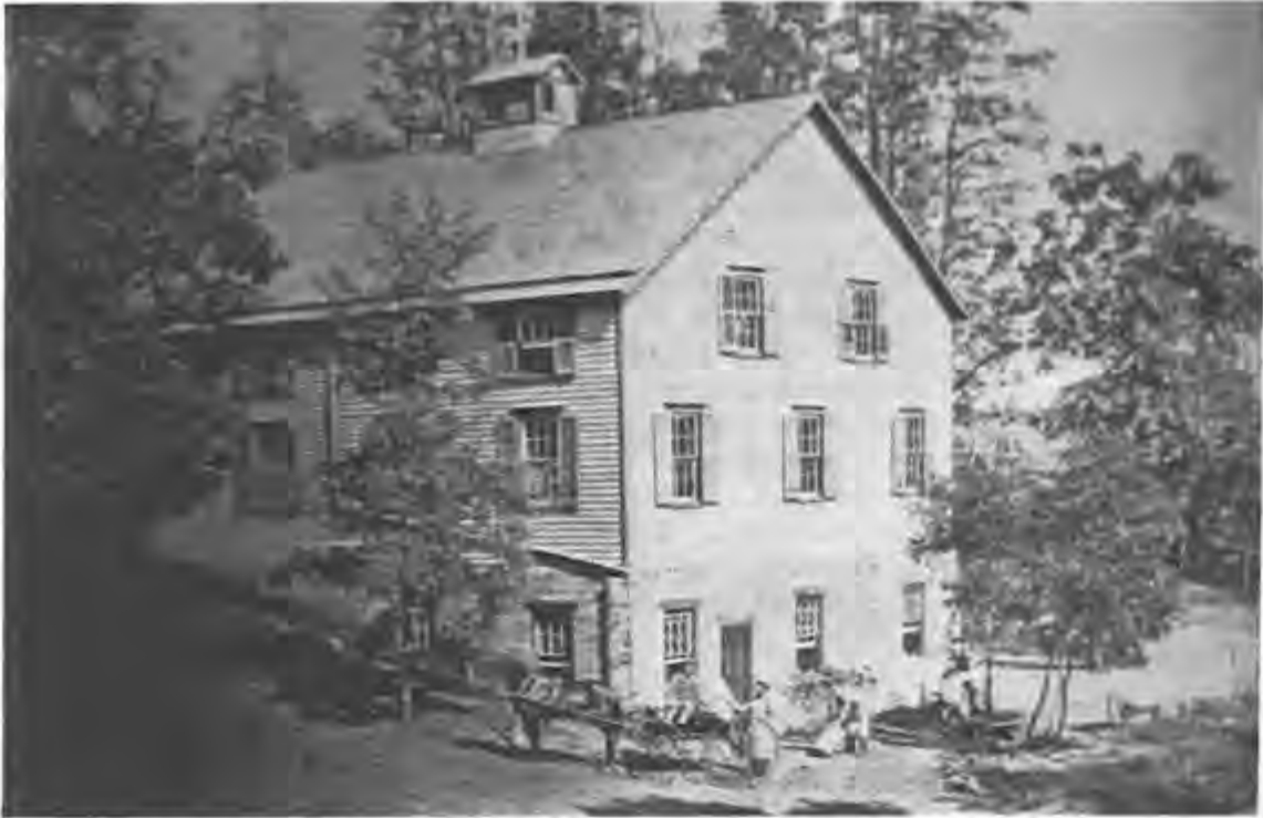
The construction of the Cream Ridge Creamery in 1881 is indicative of the rising importance of dairying in Upper Freehold in the late 19th century. (MCHSI 1351-31)
