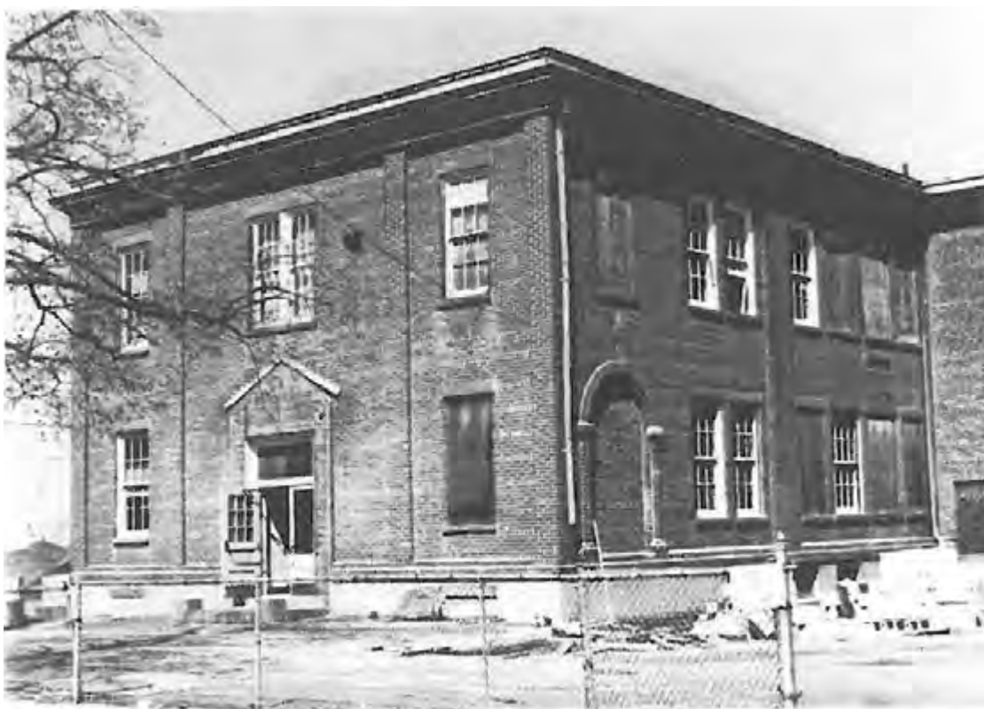
Mechanic Street School, Red Bank. (MCHSI 1340-3)
