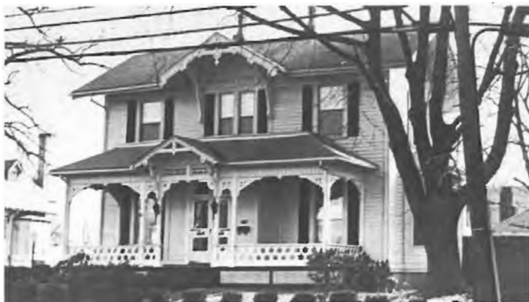
Stick Style and Eastlake ornamentation is combined on the Littlefield House in Eatontown Borough. (MCHSI 1311-5)
