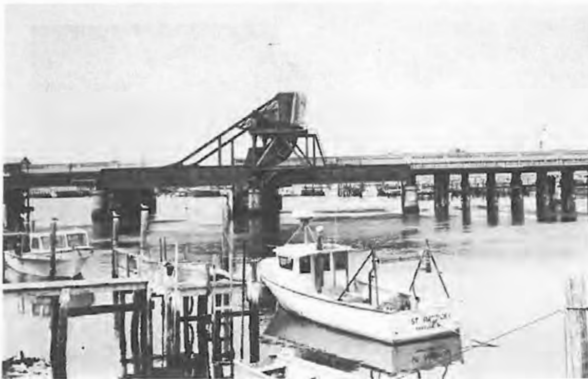
The New York and Long Branch Railroad Bridge over Shark River at Belmar is a single-leaf bascule type bridge constructed in 1935-37. (MCHSI 1306-9). In the foreground are boats and piers which are part of the considerable marine activity in the Shark River basin.
