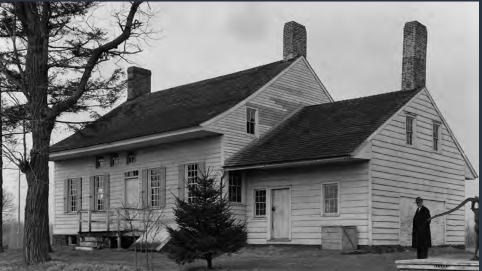
Holmes Hendrickson House, Holmdel Township, 1939. MCHSI 1318 27. Historic American Buildings Survey.
