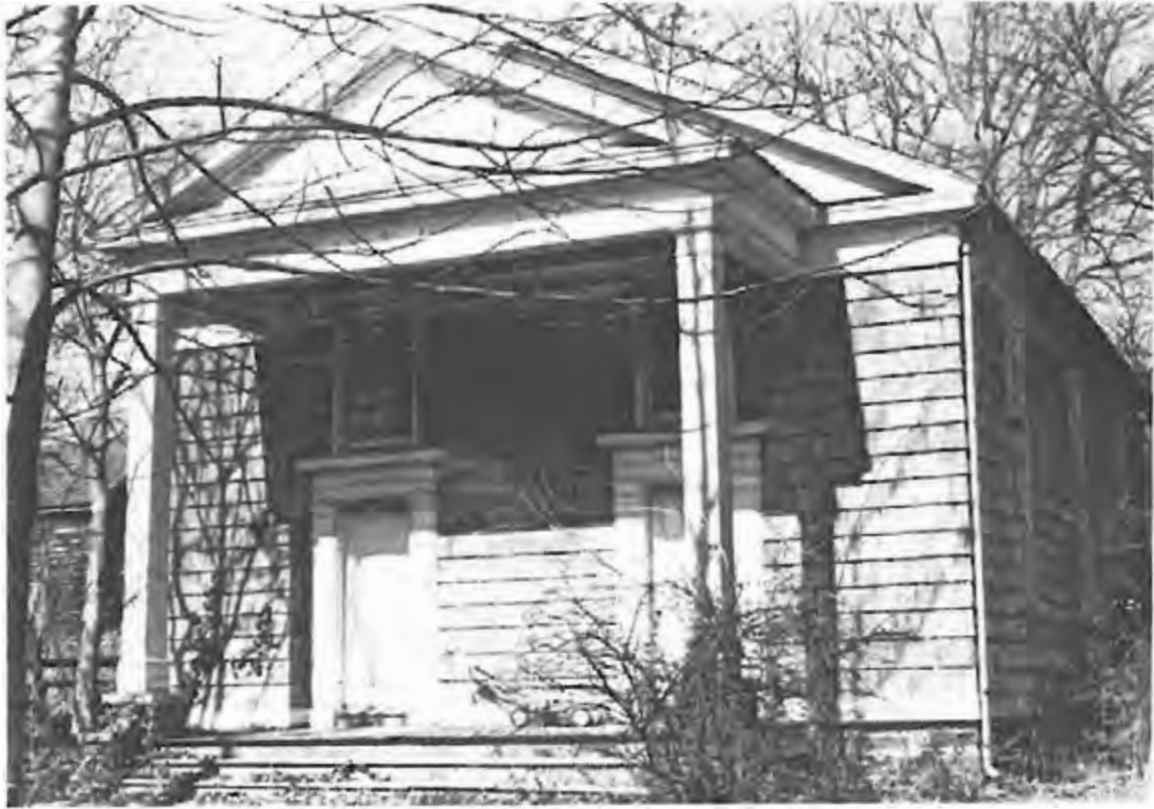
Navesink Baptist Church, Middletown Township. (MCHSI 1331-4-12)
