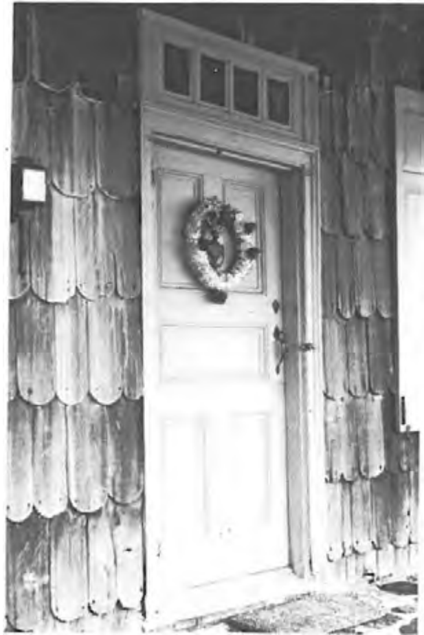
Monmouth County Georgian doorway with a split-leaf paneled door, molded surround, and four-light transom. Coward House, Upper Freehold, (MCHSI 1351-70)
