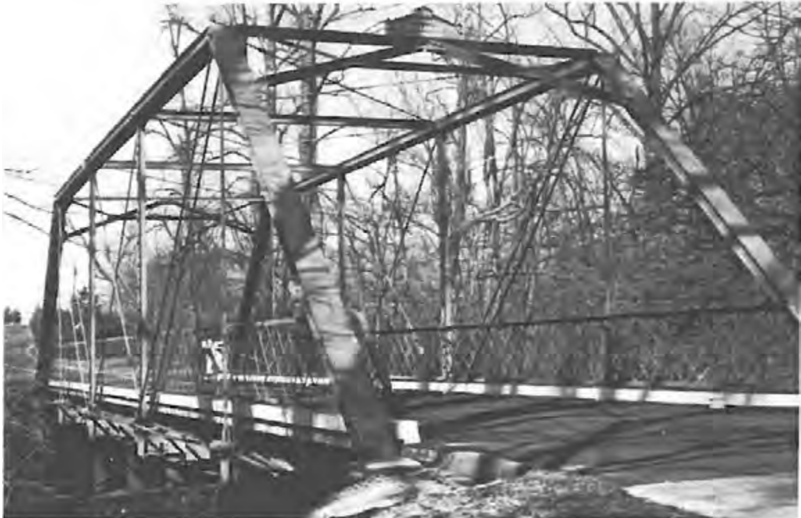
Preventorium Road Bridge, Howell Township. (MCHSI 1319-23)
