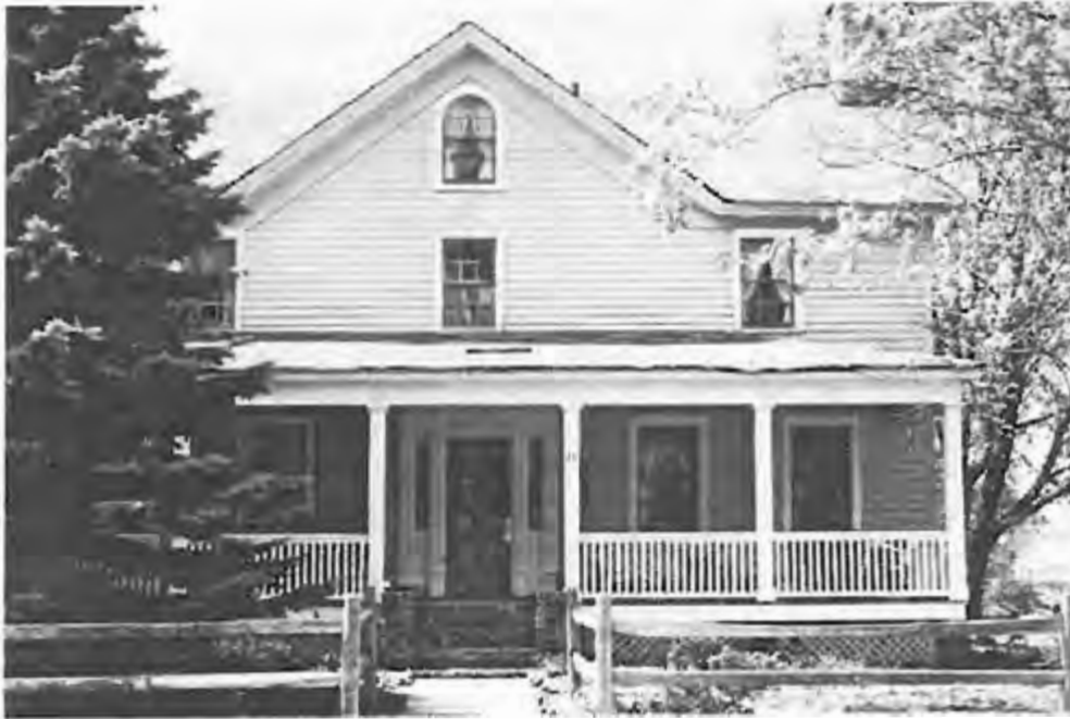
The Osborn Curtis House, built early 19th century, is among the oldest buildings now standing in Manasquan. (MCHSI 1327-4).
