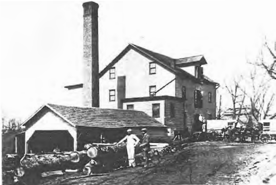
A late 19th century view of Taylor's Mill in Manalapan (no longer standing) shows a good example of a grist and saw mill complex in operation.
