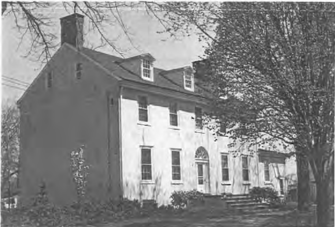
The fieldstone wing of this house, built by Anthony Woodward about 1700, is among the oldest buildings in Upper Freehold and a rare example of early stone construction in Monmouth County. The large Federal Style main block was added by the Woodwards about 1800. (MCHSI 1351-64)
