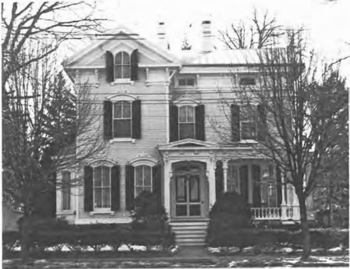
Well-conserved Victorian Italianate house in Freehold, built about 1872 by Joseph T. Laird. (MCHSI 1315-43)
