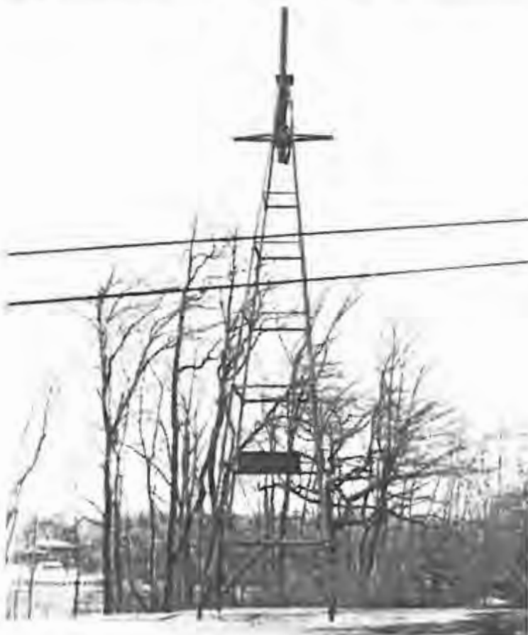
Radio antenna tower, Belmar Station. Wall Twp. (MCHSI 1352-14)
