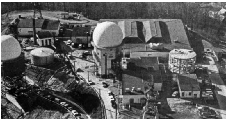
The Highlands Army Air Defense Site (H.A.A.D.S.), which housed the Missile Master control facility for the Nike missile defense of New York, seen here in the 1980s prior to demolition by the U.S. Army Corps of Engineers.
