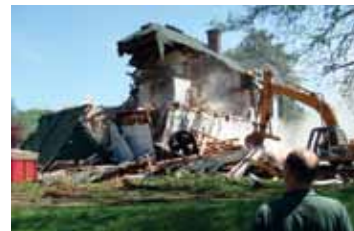
Halfway through demolition.
