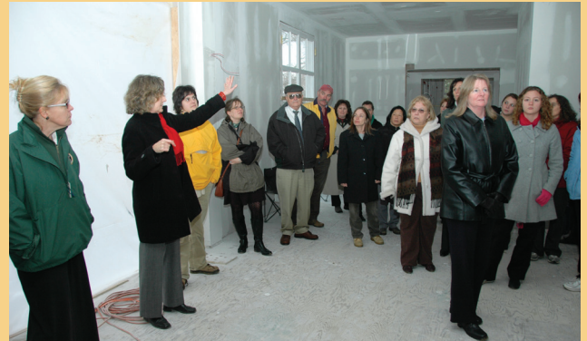
Planner and Historic Preservation Specialist Gail Hunton (pointing) managed this staff tour as well as the re-building effort, and is now the Park System's foremost expert on just about every aspect of this building and its history.
