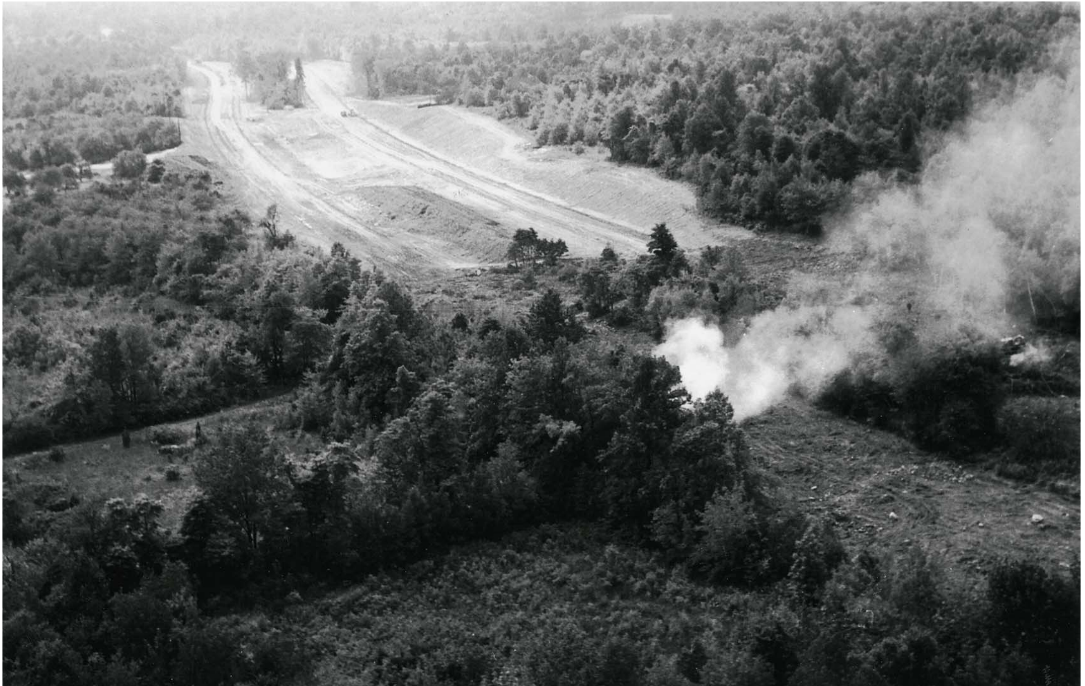
Construction of the Garden State Parkway in Wall Township, early 1950s.
