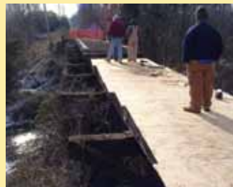
Sections of bridge on the UTT are being replaced.
