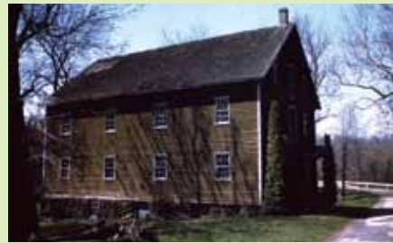
Before it was blue...the mill at Historic Wainford, 1981. (Blue was original color)
