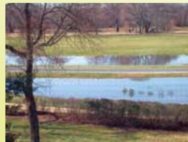
The second tier of ponds for stormwater runoff behind the Visitor Center. These are connected by pipes underneath the road, and water travels back and forth between them.
