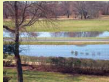
The second tier of ponds for stormwater runoff behind the Visitor Center. These are connected by pipes underneath the road, and water travels back and forth between them.
