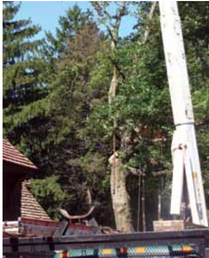
This crane removes a large tree from the roof of the Huber Woods Environmental Center.
