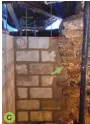
Other portions of foundation had to be removed altogether, and rebuilt from scratch. This kind of major structural work required temporary steel beams to support the south corner of the house while work got underway (A). The old foundation was replaced with this rebar-enforced, concrete footing (B) followed by a new concrete block wall (C). Note how the stone masons expertly 'joined' new wall to old. They also topped the new wall with salvaged old stones so no one would notice repairs from the outside.
