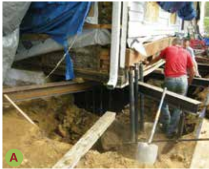
Other portions of foundation had to be removed altogether, and rebuilt from scratch. This kind of major structural work required temporary steel beams to support the south corner of the house while work got underway (A). The old foundation was replaced with this rebar-enforced, concrete footing (B) followed by a new concrete block wall (C). Note how the stone masons expertly 'joined' new wall to old. They also topped the new wall with salvaged old stones so no one would notice repairs from the outside.
