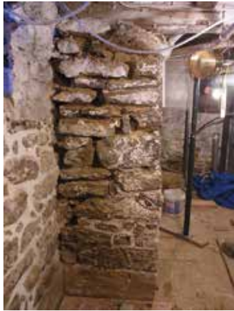
Some portions of the original stone foundation underneath the house needed re-pointing [that's when the crumbling old mortar is removed (left) and re-filled with new mortar (right)].
