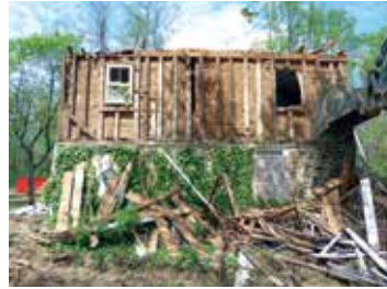
The Millhouse during demolition, note the ivy covered stone wall.
