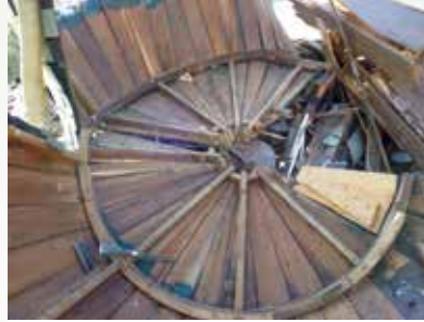
A close-up inside the demolished silo, shows how it was built.
