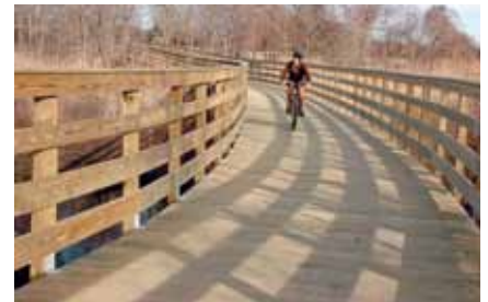
Ryan Kimble of Outdoor Adventures tests the new bridge over Marlu Lake, completed January 2012. The bridge itself is 10 feet wide and 543 feet long-or 181 yards (that's almost two football fields, minus the end zones of course).
