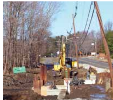
The MT-52 bridge along Route 520, as of late January.
