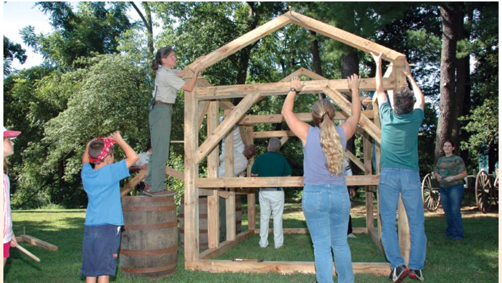
Could you assemble this frame without hammer or nails? Sarah Bent (standing on barrel, left) and Sandy Byard (third from right) show program attendees at Walford how to frame this model barn with fitted wood beams held together by pegs.
