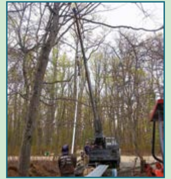
Installing a well requires some big equipment.
