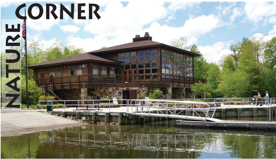
Enjoy striking views of the water and treescape at the Manasquan Reservoir Visitor Center. Three sides of this building have windows that frame the surrounding reservoir. (left)
