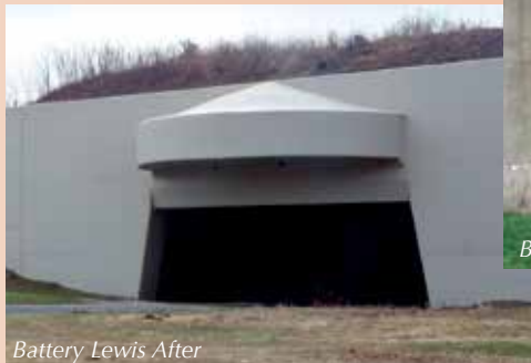
Battery Lewis After
