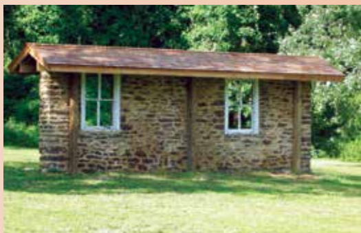
Salvaging this stone wall from a demolished mill house, to be used as a kiosk, helps remind visitors of the history of the Claypit Creek Section of Hartshorne Woods Park .
