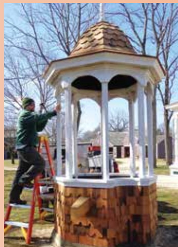
Park System carpenters restored this Longstreet Farm well house in 2013.
