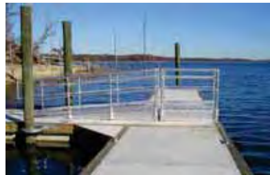
A new floating dock.
