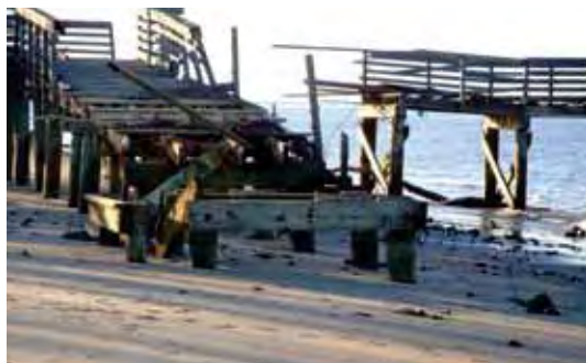
This storm damaged fishing pier was quickly repaired.
