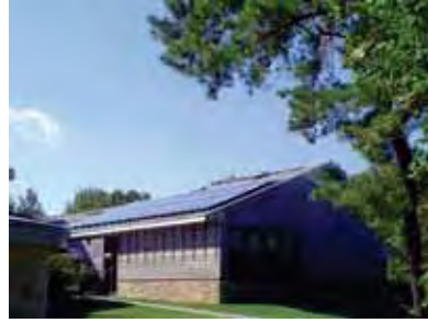
New solar panels.
