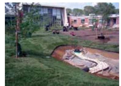
Park staff helped design this water-conserving rain garden in Holmdel, shown here under construction.
