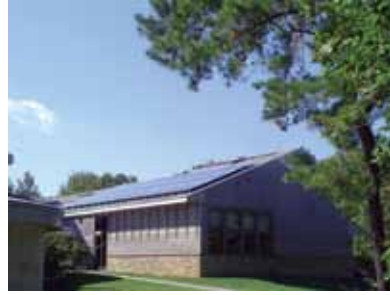
New solar panels.
