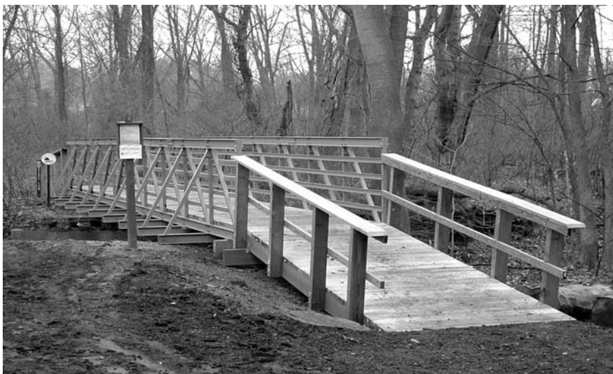
New trail bridge in the Ramanessin section of Holmdel Park
