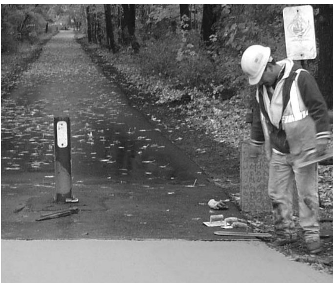
Repared 7,966 feet of the Henry Hudson Trail
