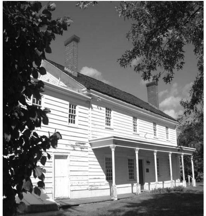
Seabrook Wilson House at Bayshore Waterfront Park
