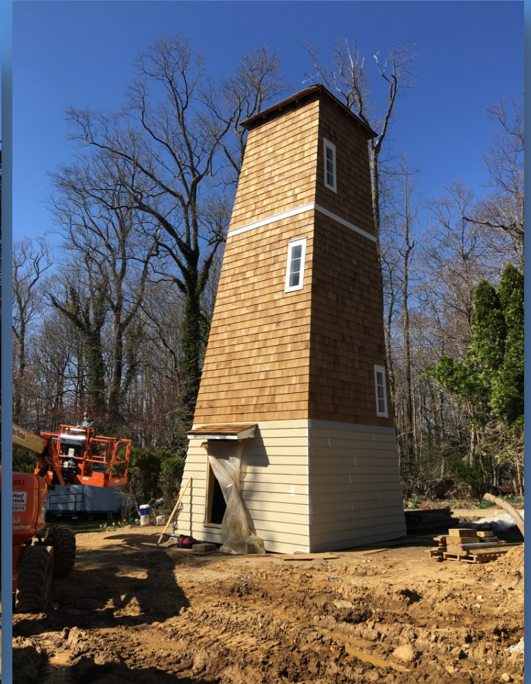
Restored 1880s Water Tower
