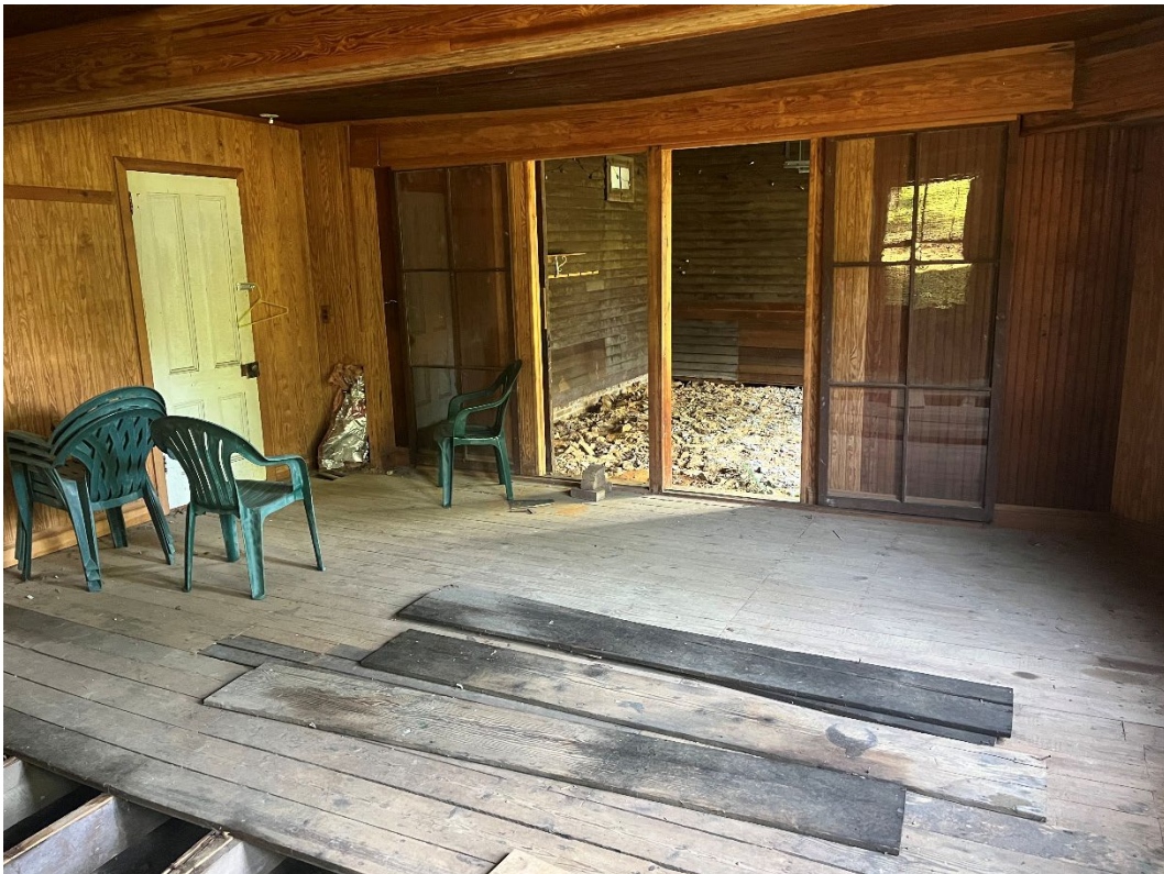
Portland Place Carriage House, Interior Conditions
