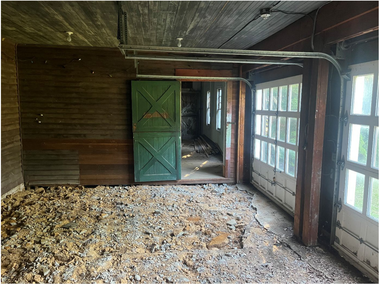
Portland Place Carriage House, Interior Conditions
