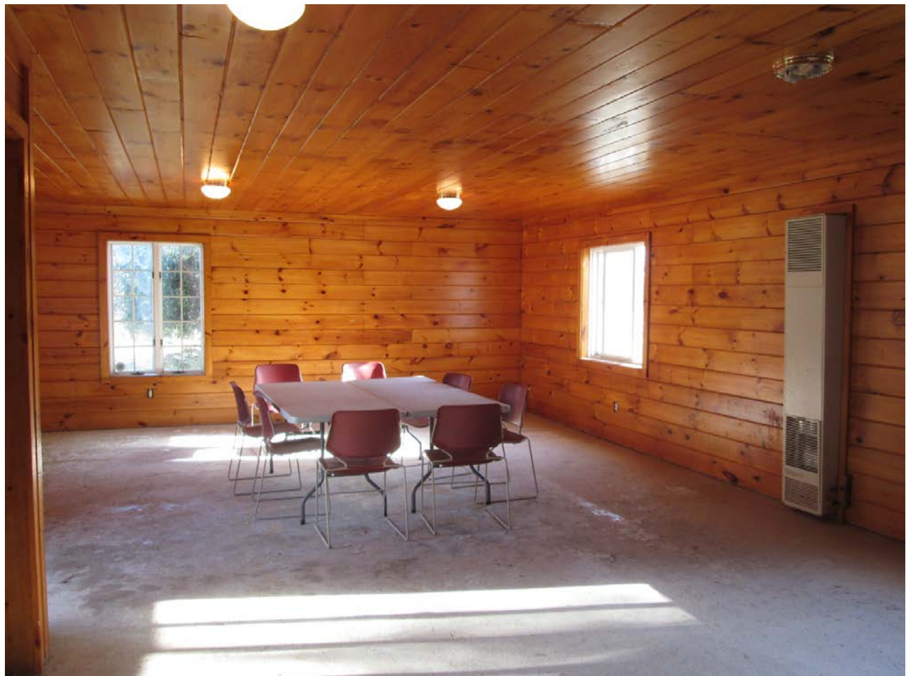
Former tack room to be converted to programming space
