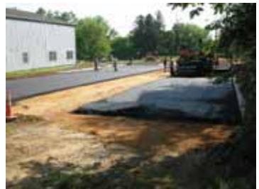
Then, they finally began laying asphalt.
