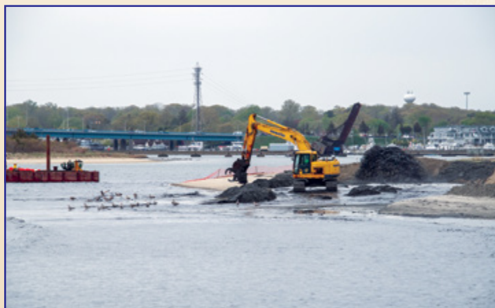
Wills Hole emergency dredging project from April in Point Pleasant and Manasquan to improve navigation safety in the channel. The $1.35 million dollar project restored the channel to a safe navigable depth by dredging approximately 32,000 cubic yards. Photo taken at Fisherman's Cove Conservation Area.
