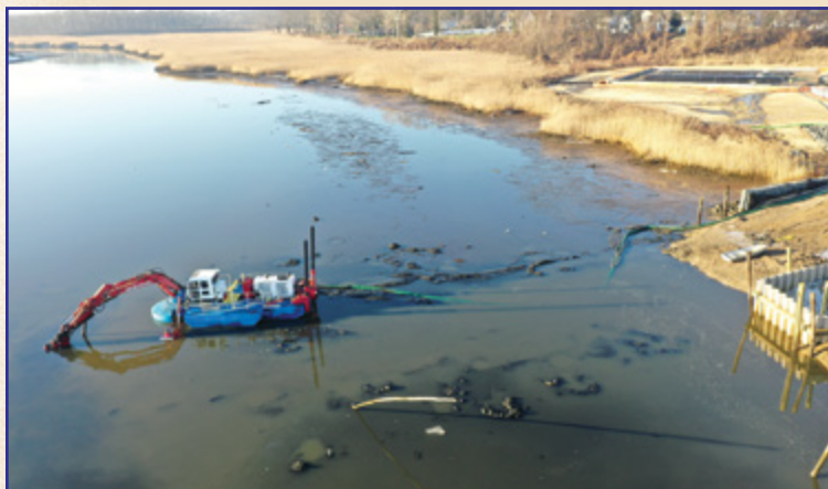
Wills Hole emergency dredging project from April in Point Pleasant and Manasquan to improve navigation safety in the channel. The $1.35 million dollar project restored the channel to a safe navigable depth by dredging approximately 32,000 cubic yards. Photo taken at Fisherman's Cove Conservation Area.
