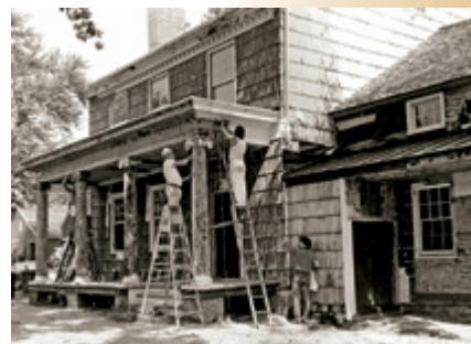
Longstreet Farmhouse Restoration-1981
