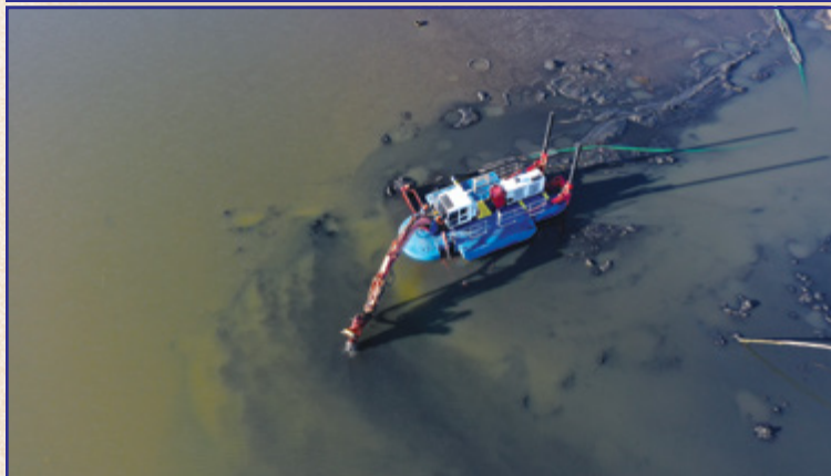
Dredging boats removed a total of 14,000 cubic yards of sediment from the channel. The river is now at least four feet deep at mean low water from the Swimming River Park boat ramp to the Rt. 35 bridge. The dredged material was beneficially utilized as cover at the Monmouth County landfill in Tinton Falls.
