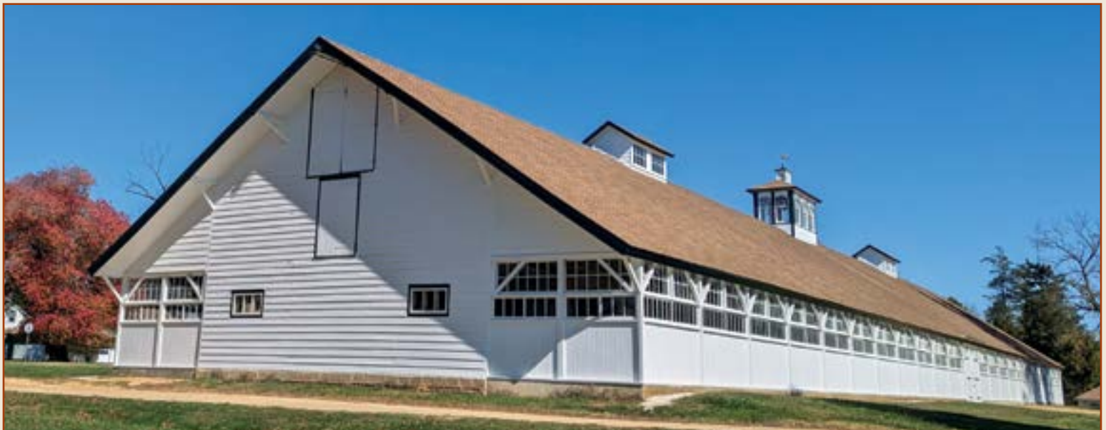
The Historic Racing Stable after rehabilitation, 2024.
