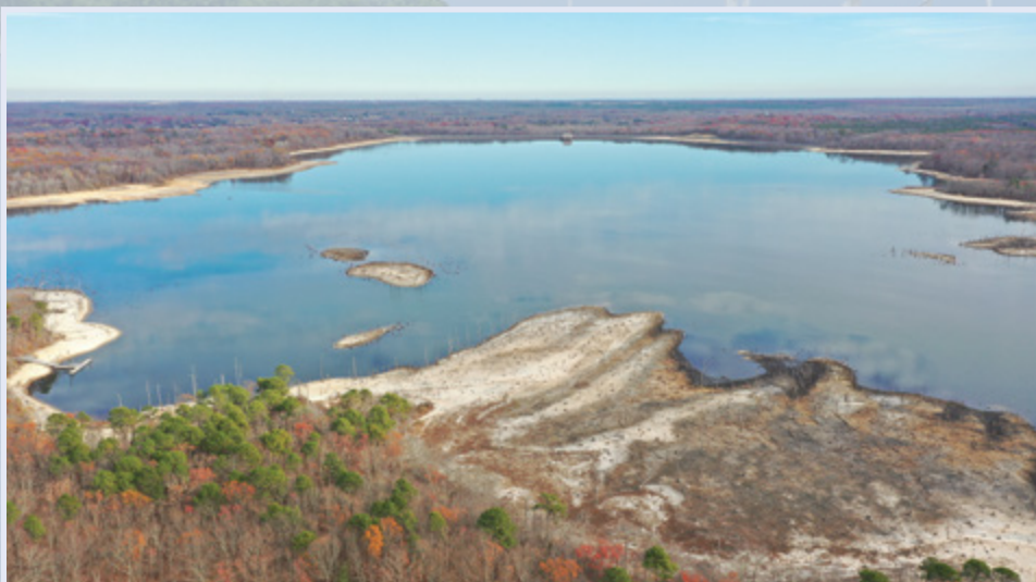
Arial View of the Manasquan Reservoir in November 2024
