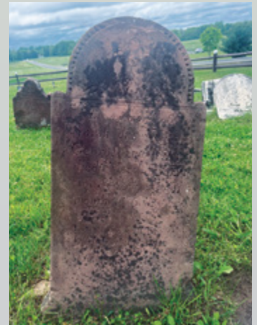
The sandstone headstone of Sarah Smock (left), who died in March 1794, remains in excellent condition despite the abundance of bio growth and atmospheric pollutants.
