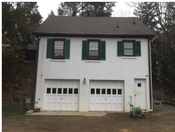
Photo Above: Building #1402 Cottage
