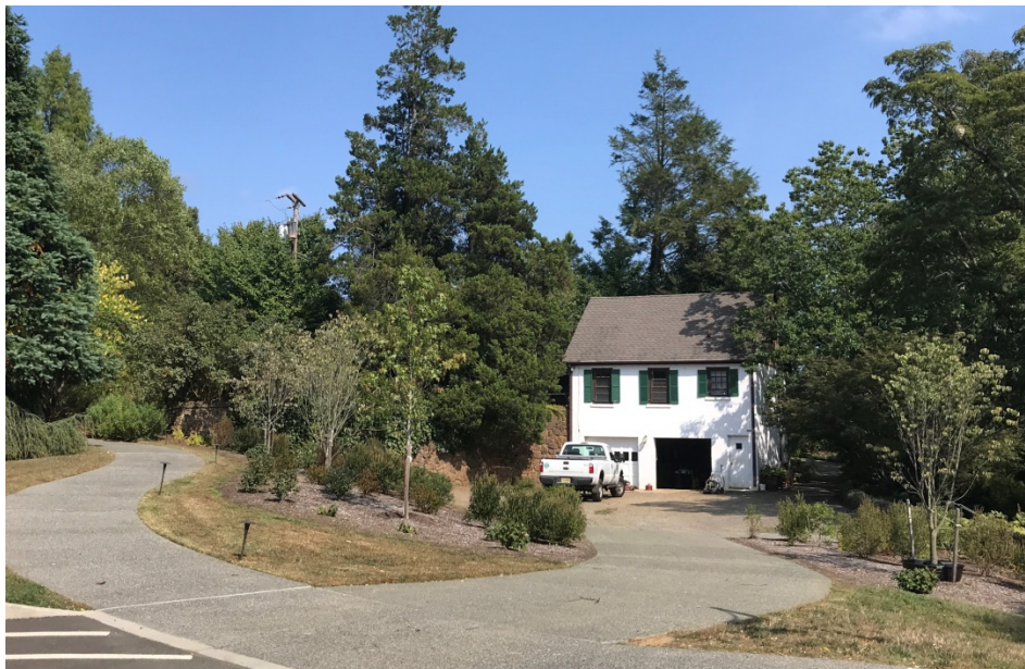
Photo Above: Building #1402 Cottage
